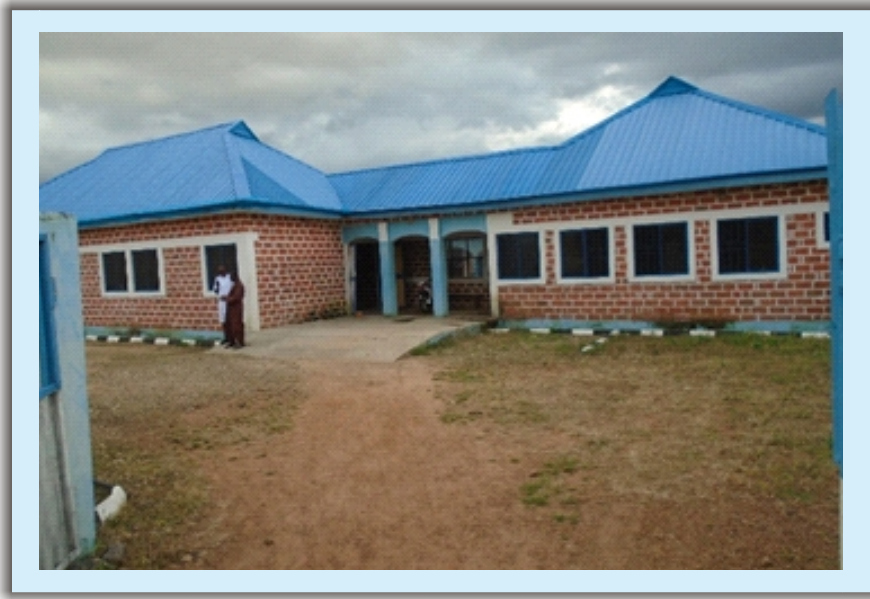
RENOVATED & EQUIPPED BERI PRIMARY HEALTH CARE CENTRE
