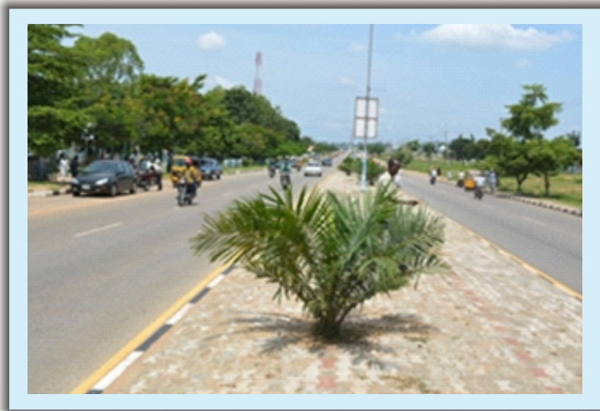
MINNA CITY INTERLOCK PROJECT
