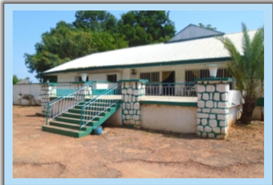
RENOVATED GOVERNMENT LODGE BIDA
