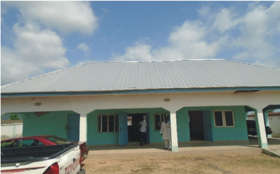
RENOVATION OF SHARIA COURT OF APPEAL, PAIKO
