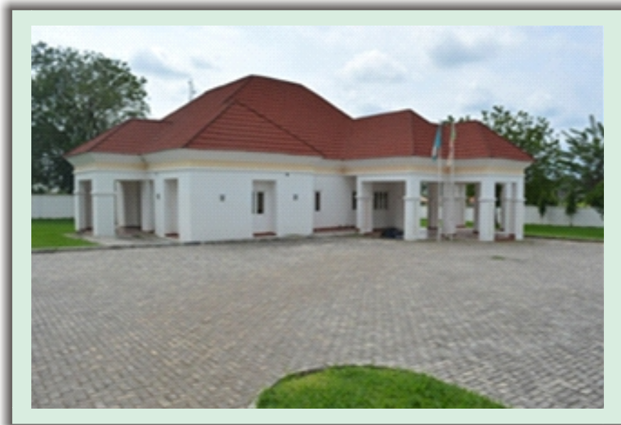
RENOVATED GOVERNMENT LODGE BIDA
