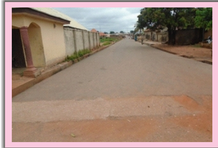
ON-GOING CONSTRUCTION OF 4NOS ROADS IN KONTAGORA
