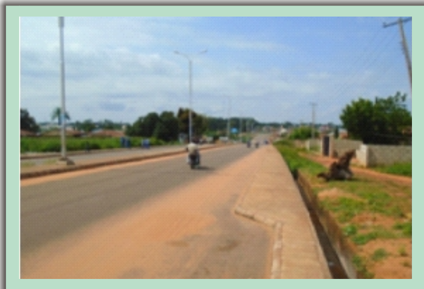
CONSTRUCTED 2.6KM BANGAIE DARACHITA ROAD BIDA
