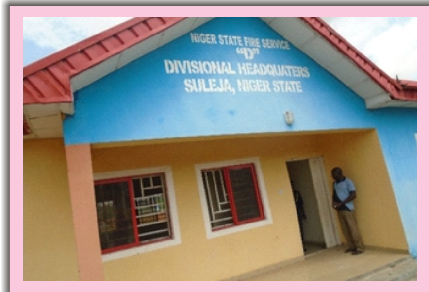
ON-GOING CONSTRUCTION OF FIRE SERVICE STATION, SULEJA
