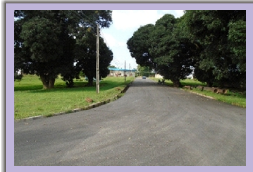
ACCESS ROAD CONSTRUCTED WITHIN CHANCHAGA WATER WORKS, MINNA
