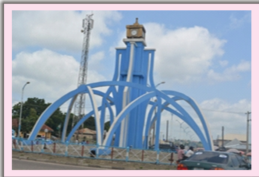
CONSTRUCTION OF MOBIL OBASANGO AND BAHAGO ROUNDABOUT
