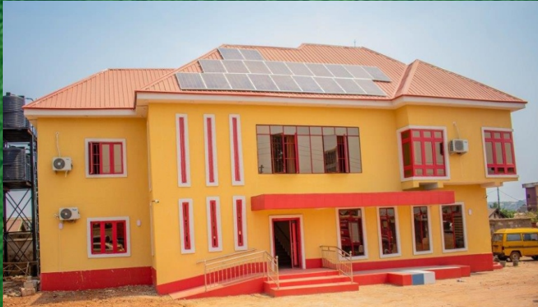
FIRE SERVICE HQRTS ENUGU
