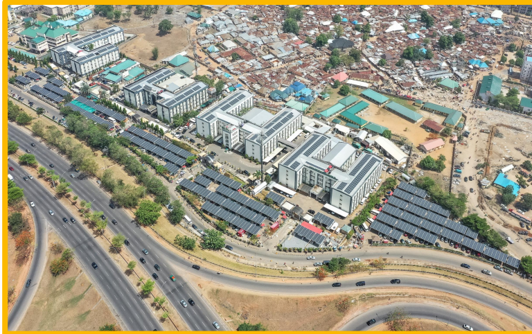
Deployment of Renewable energy (Solar + Hydro + Storage)
