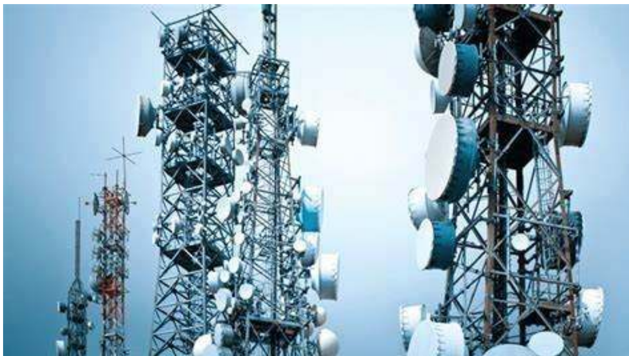
Figure 44: Telecommunication in Nigeria
