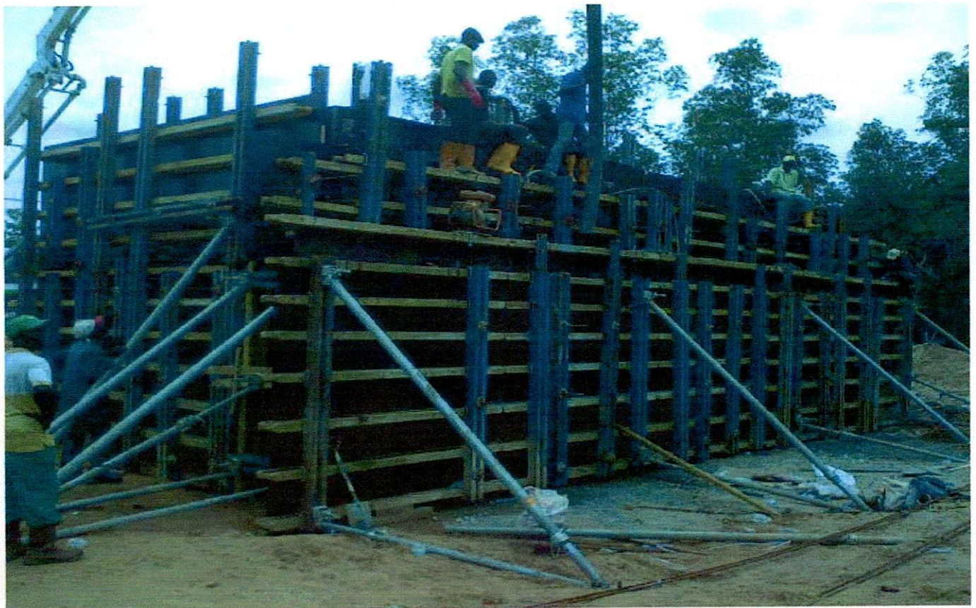
TRANS-WARRI COVERAGE SHUTTERS OF ABUTMENT AT BRIDGE 7-IJALA SPUR
