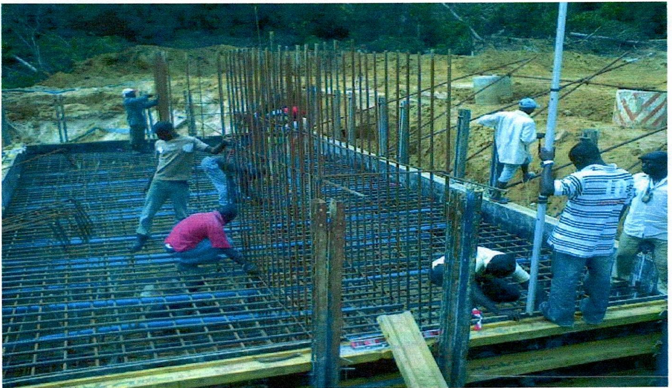
TRANS-WARRI COVERAGE SHUTTERS OF ABUTMENT AT BRIDGE 7-IJALA SPUR
