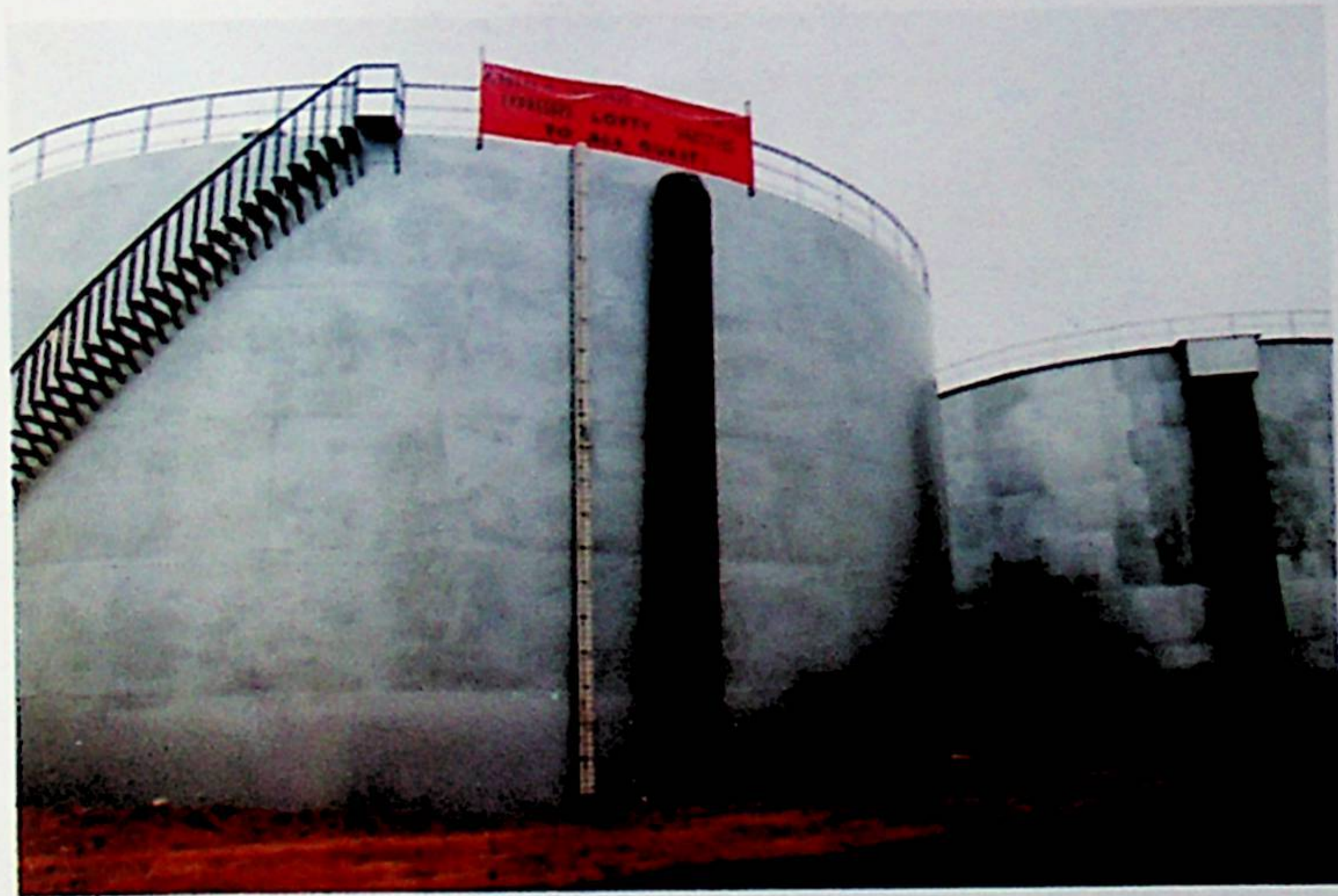
20 million gallons Asare Water project
