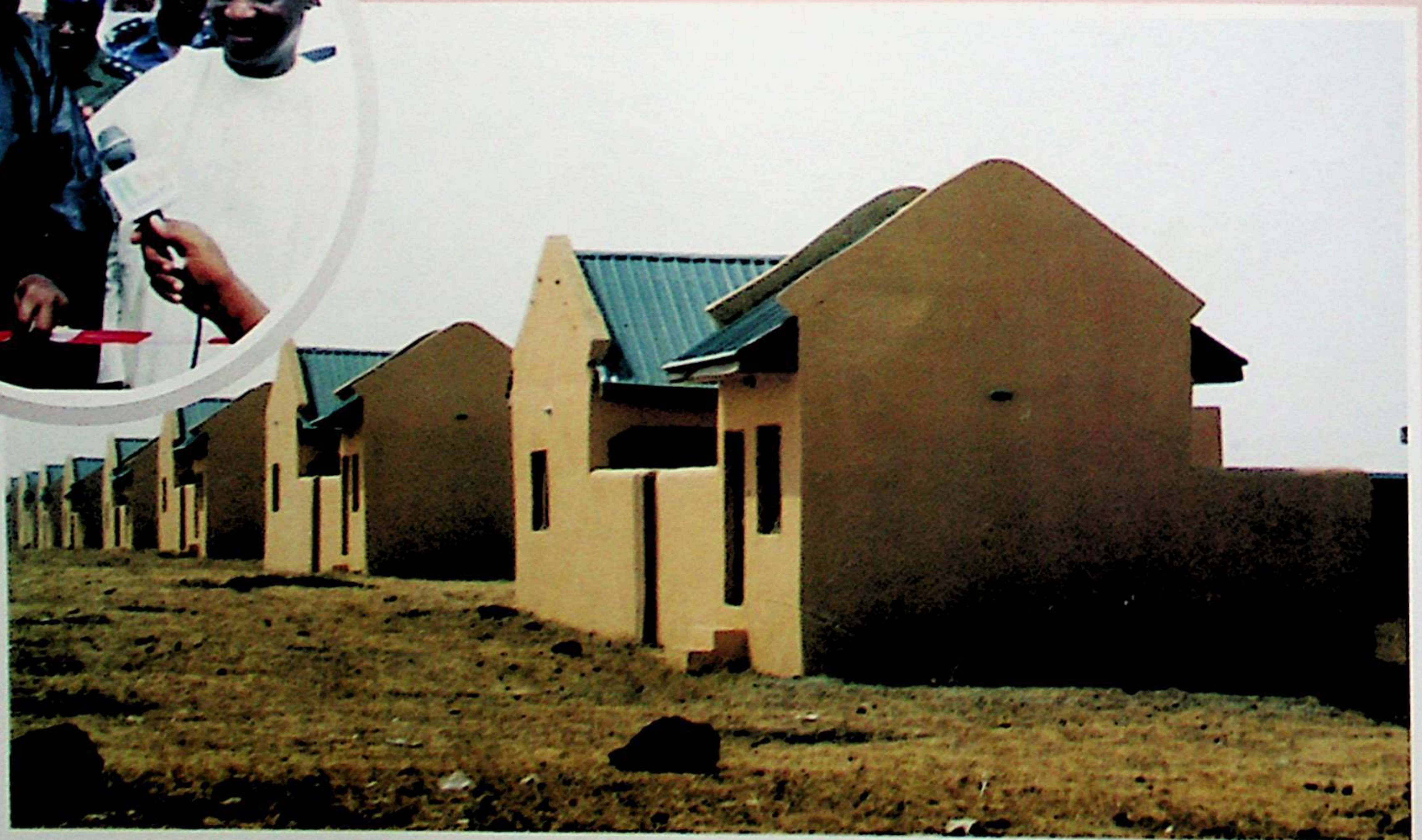
350 housing units for 2010 flood victims at Tsaro in Gada local government
