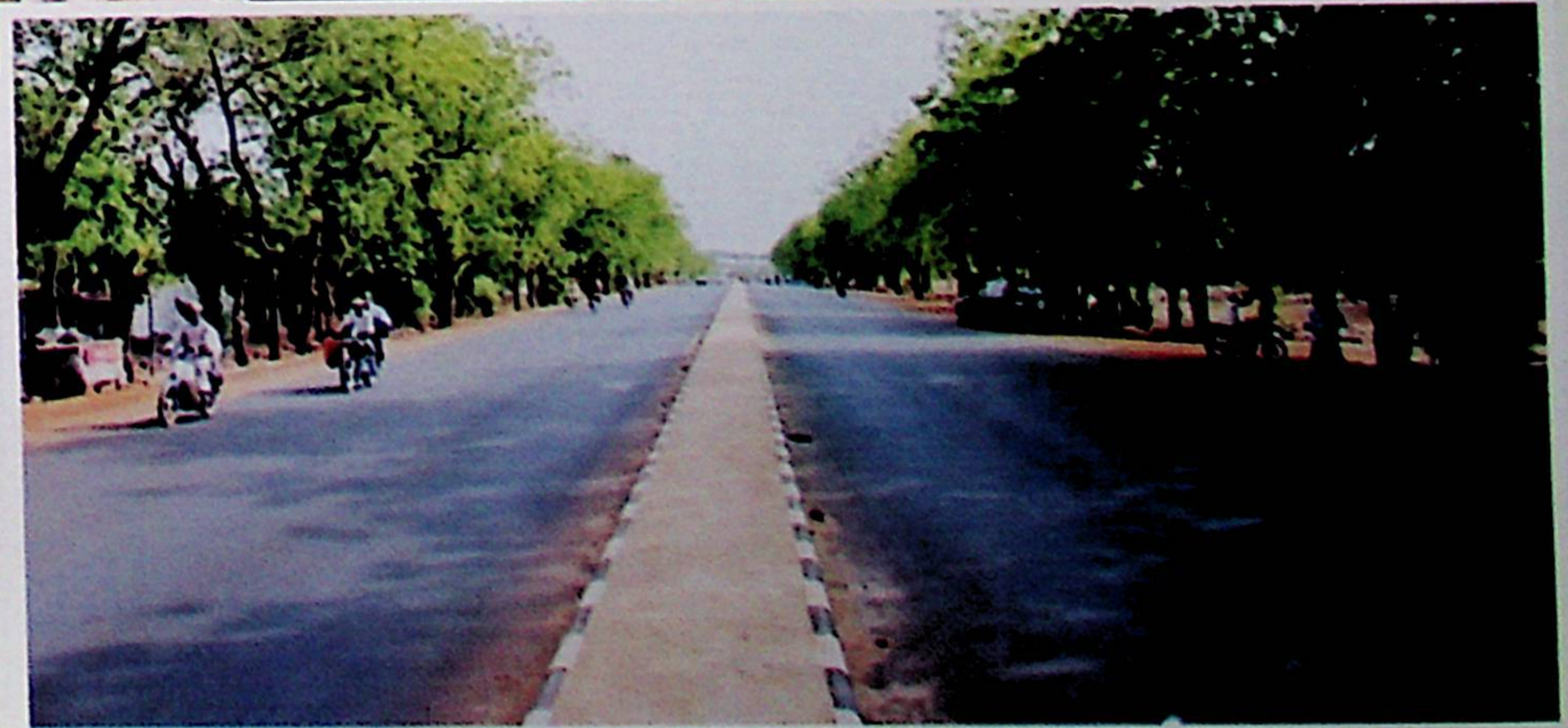
On-going construction of multi billion naira Western bye-pass road by Gov. Wamakko
