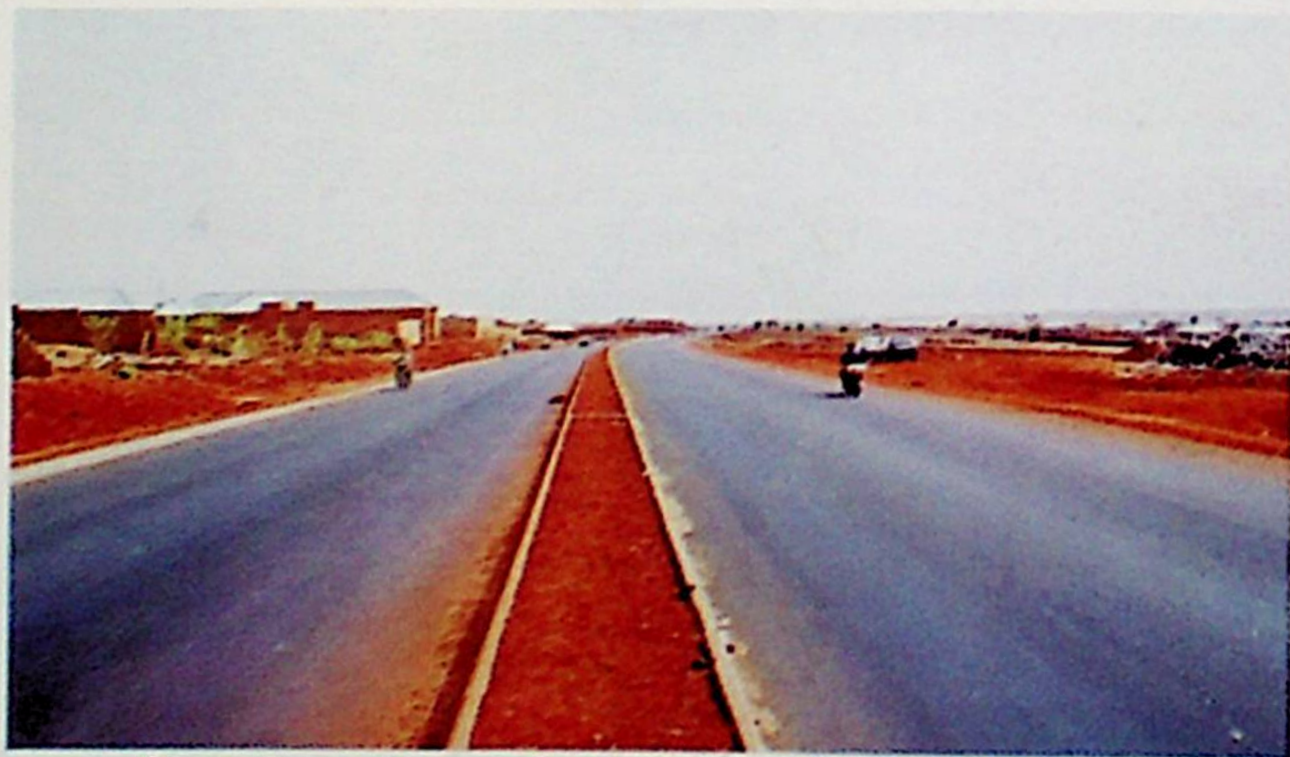
On-going construction of multi billion naira Eastern bye-pass road
