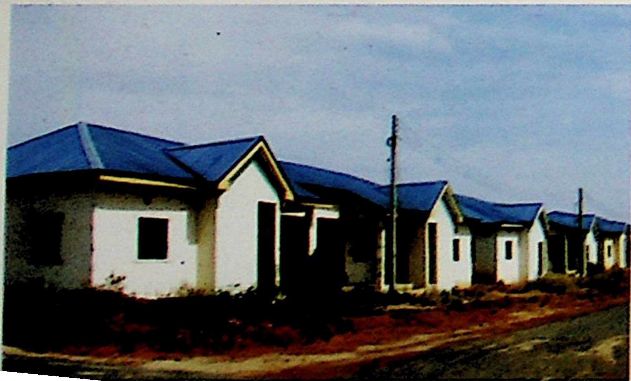
Housing estate at Bado
