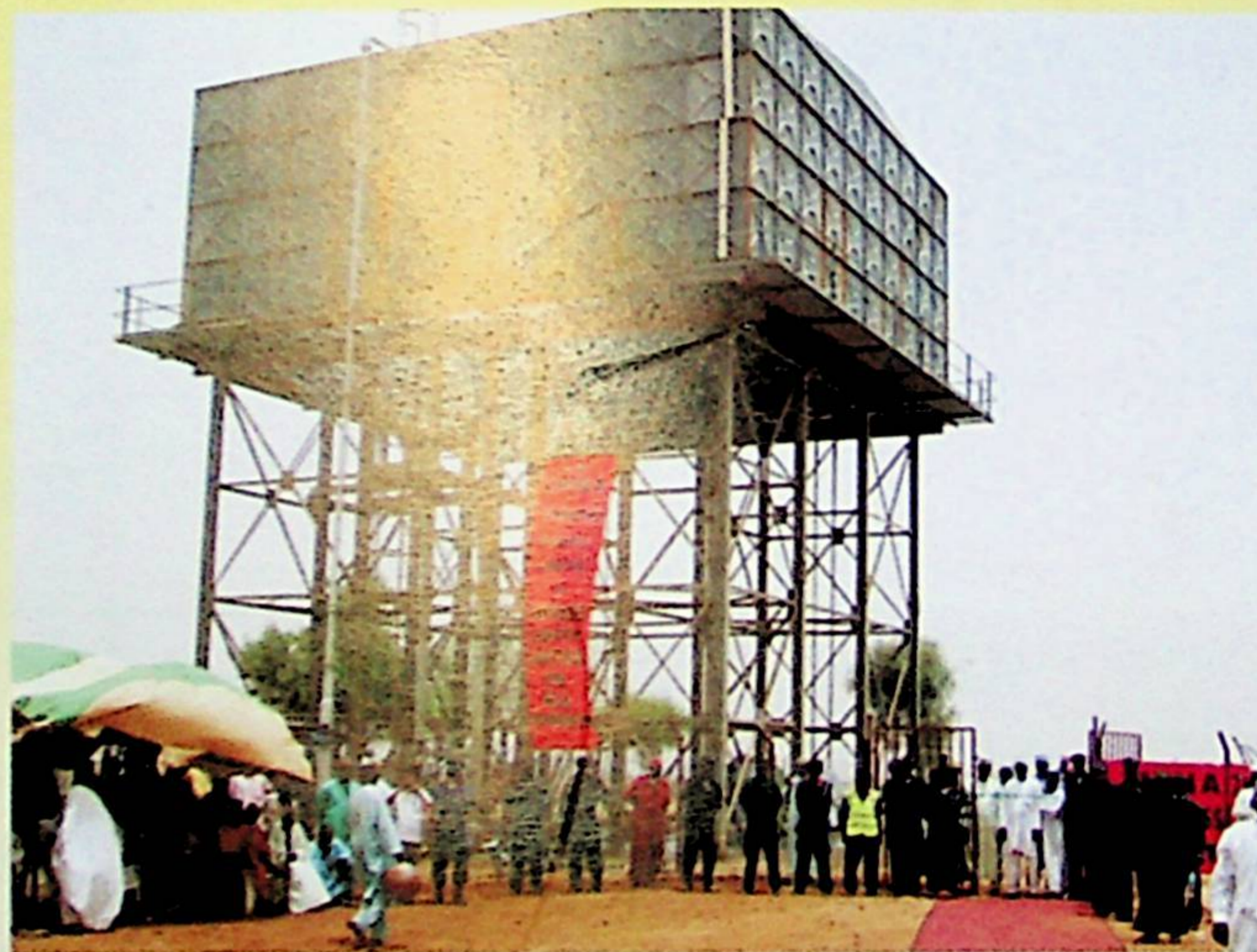
One of the various water projects executed by Gov. Wamakko's administration
