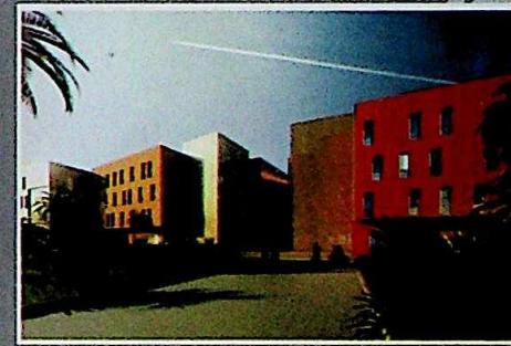
View of a secondary facade of Engineering School
