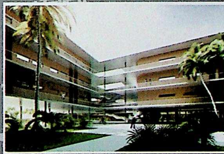
Interior view from the courtyard of Engineering School
