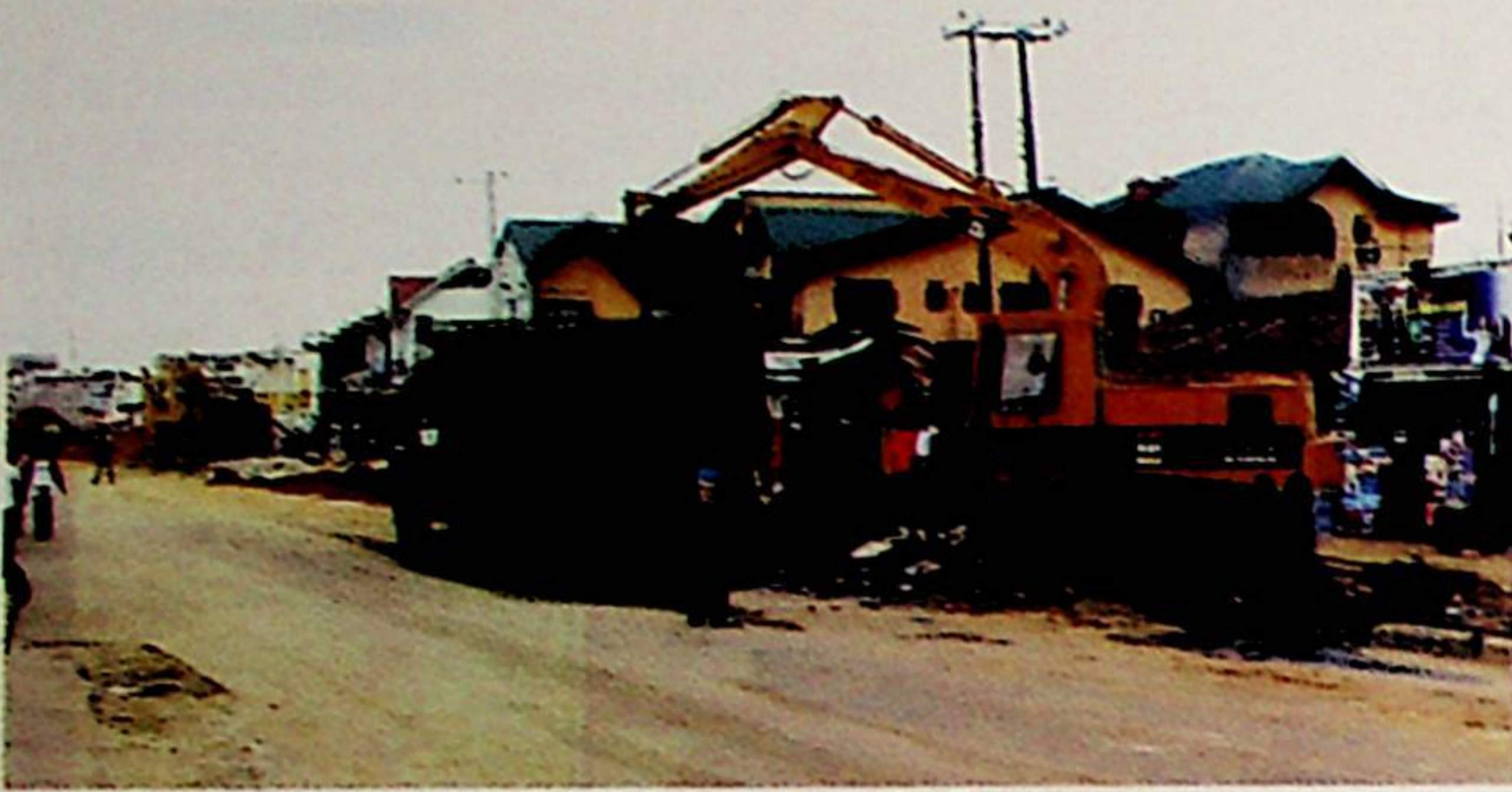
Work in progress on the Apani internal roads, Ikwerre
