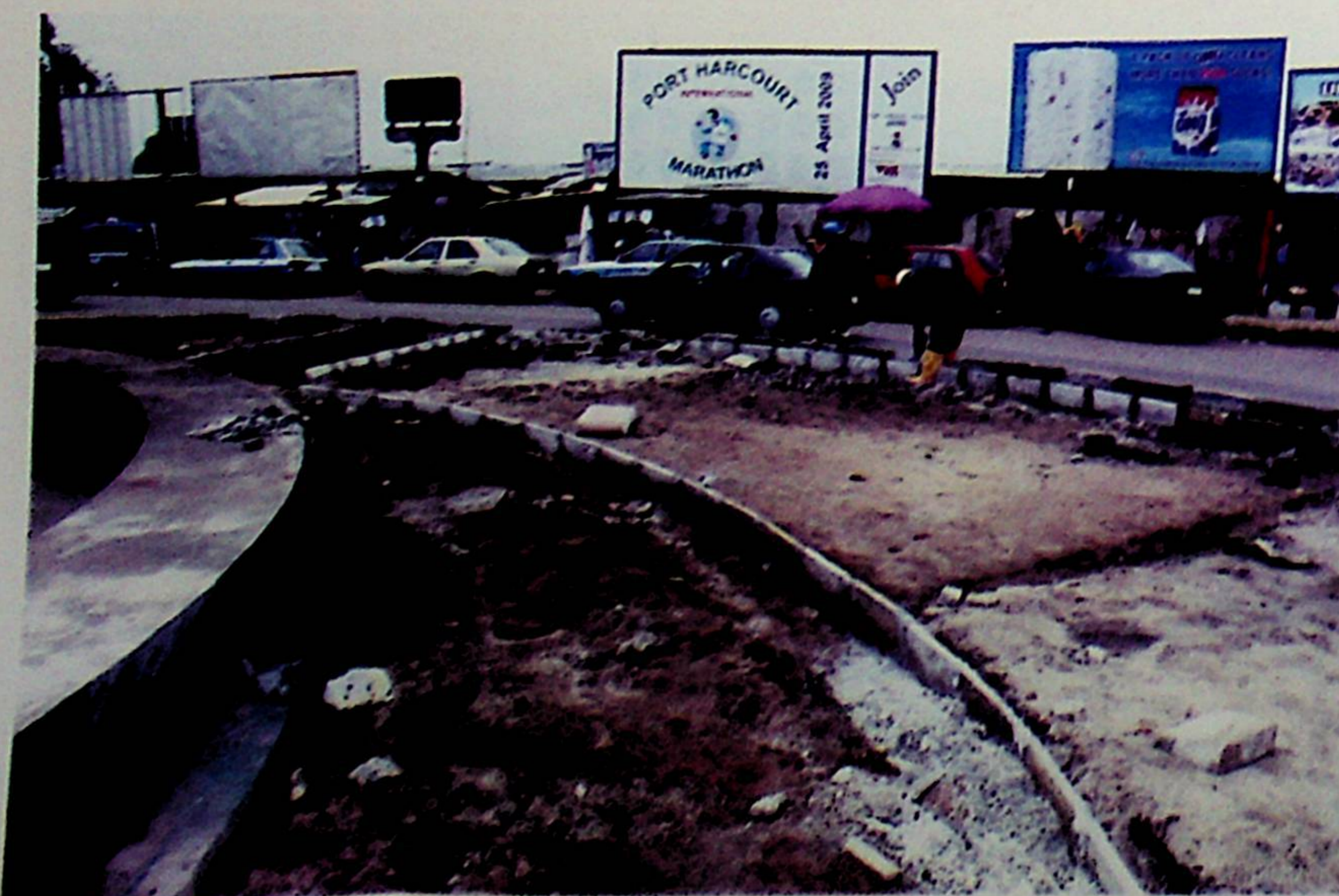
Beautification of a Port Harcourt road underway
