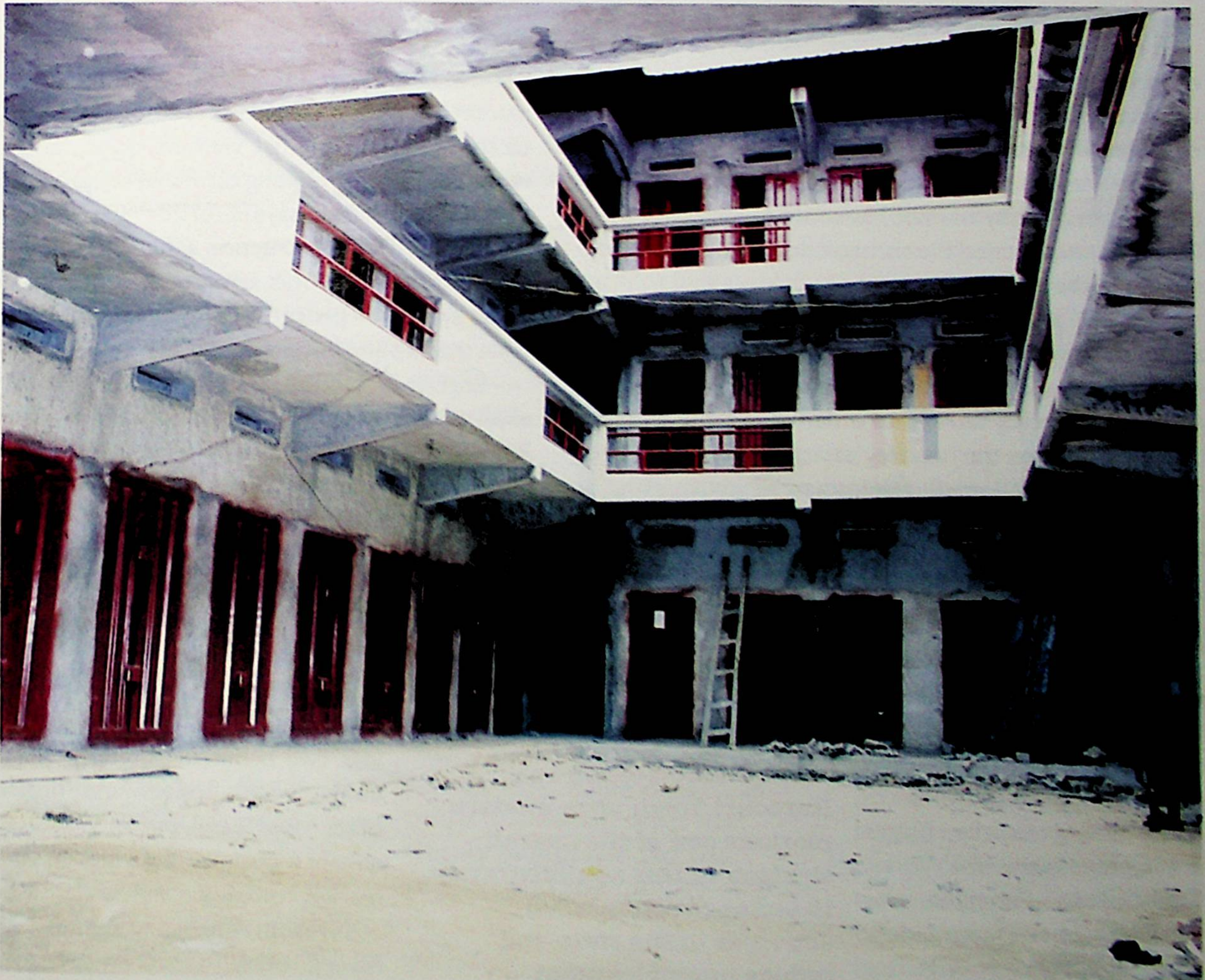
Mile One ultra modern market near completion
