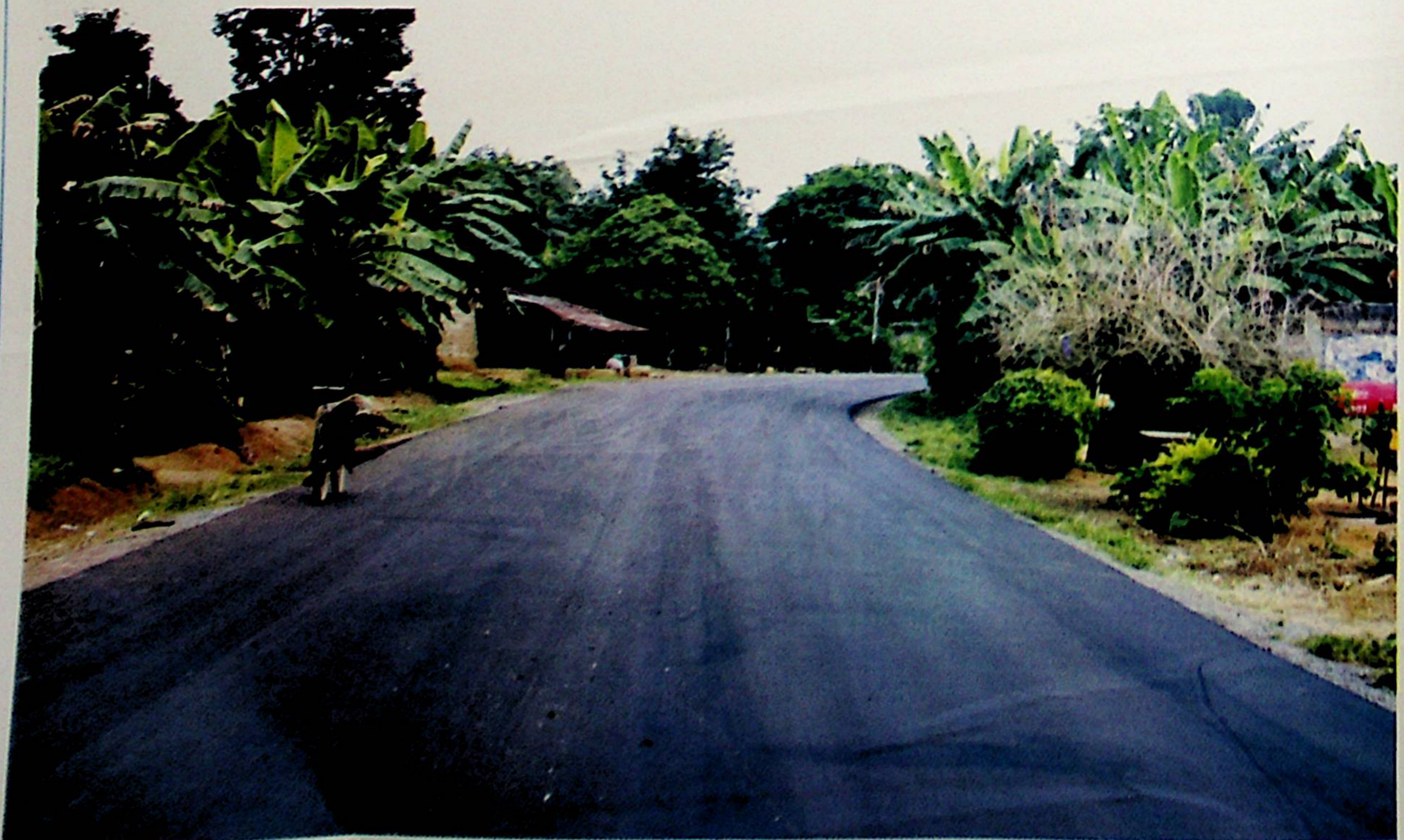
A rural road project in Ikwerre LGA
