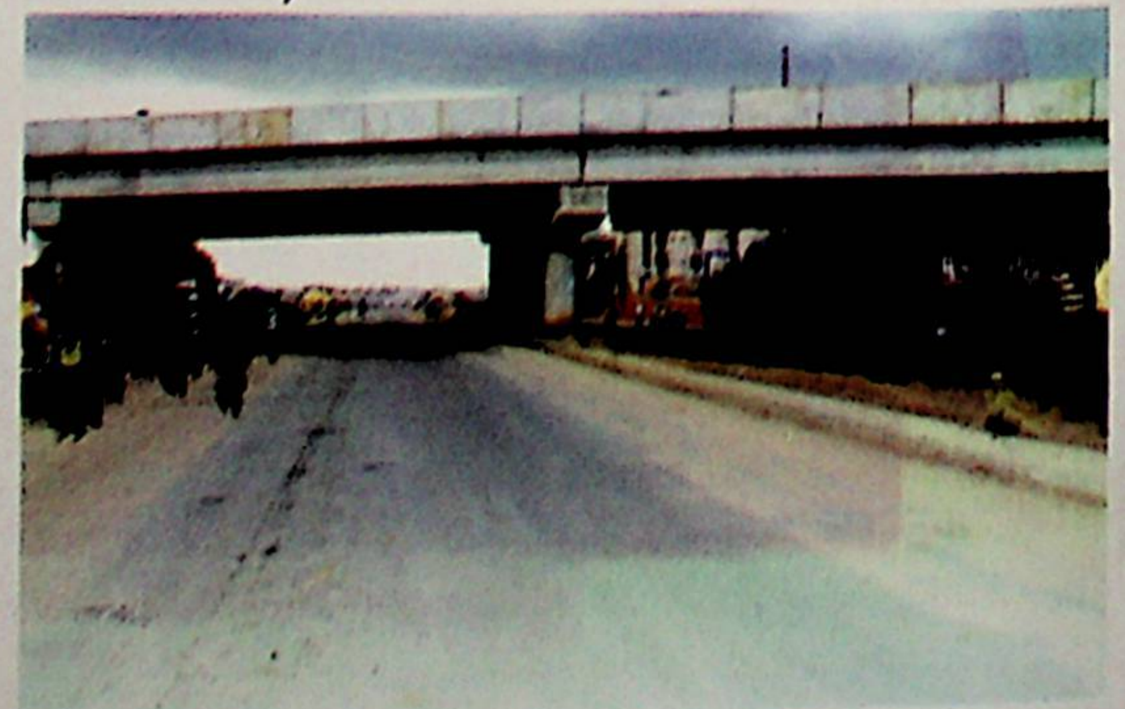
Eleme junction flyover on interchange
