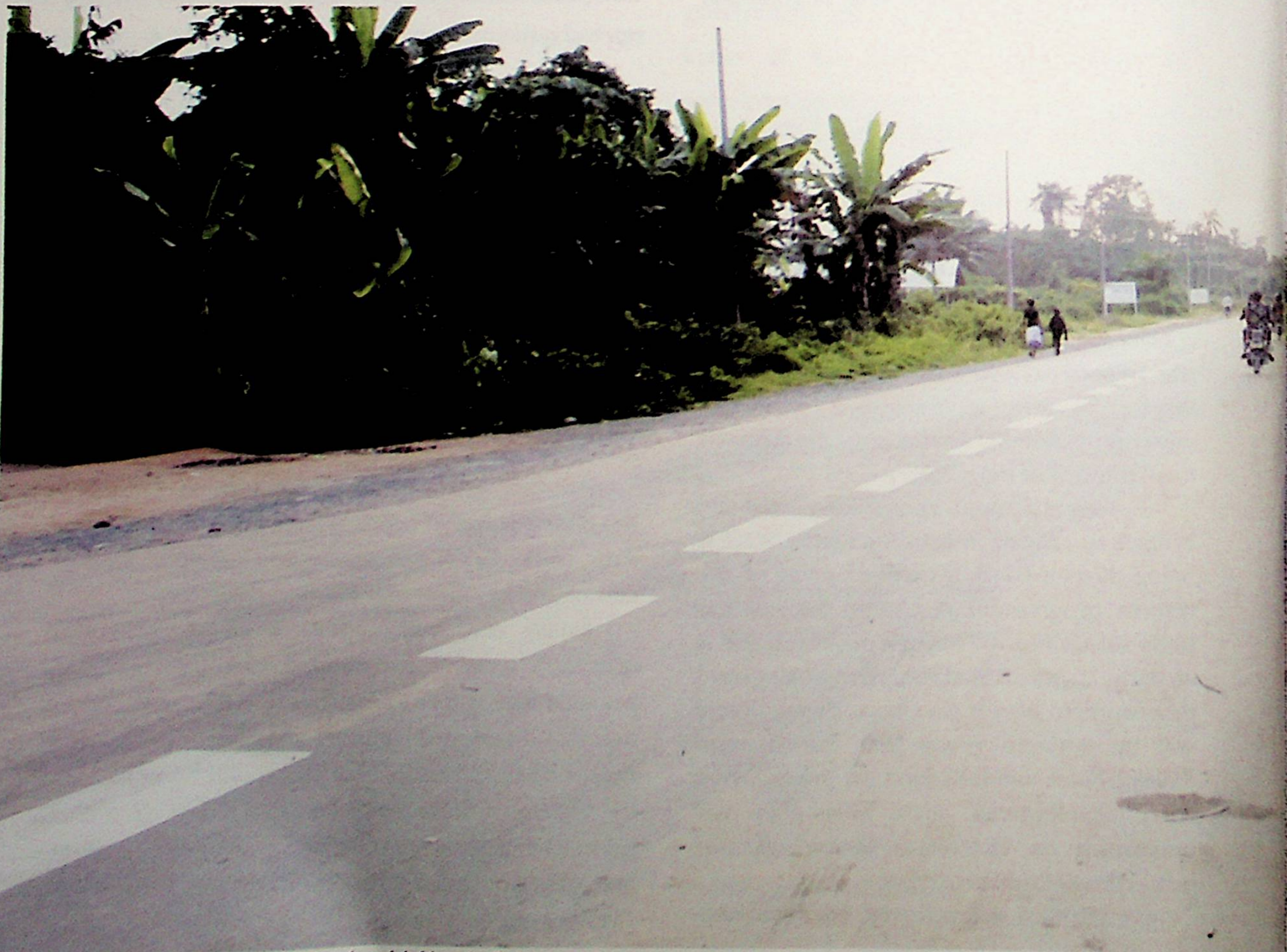
Construction of Omerehu-Ozuzu-Okehi Road and bridges in Etche
