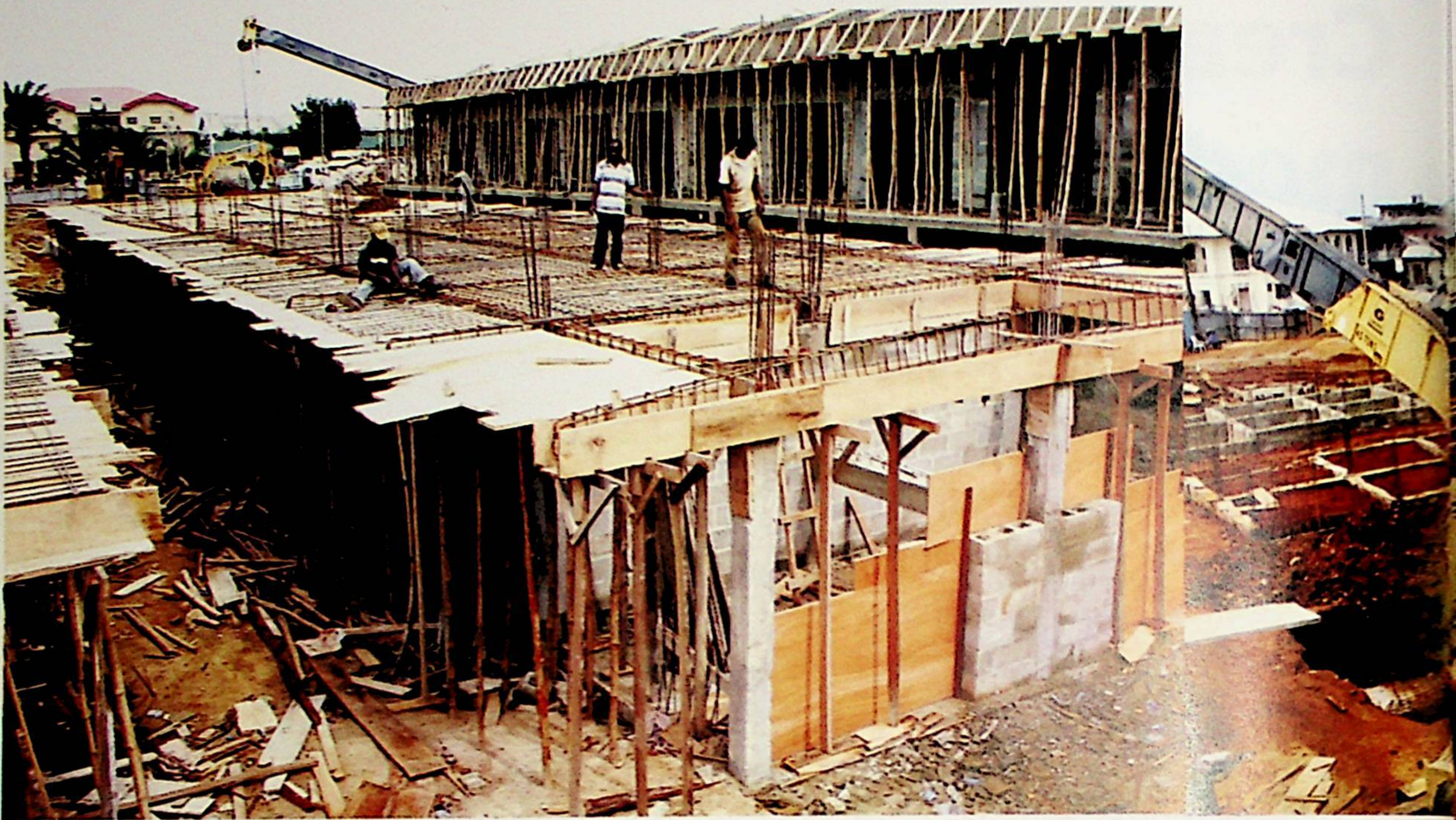
Construction of the Mile One Ultra-Modern market
