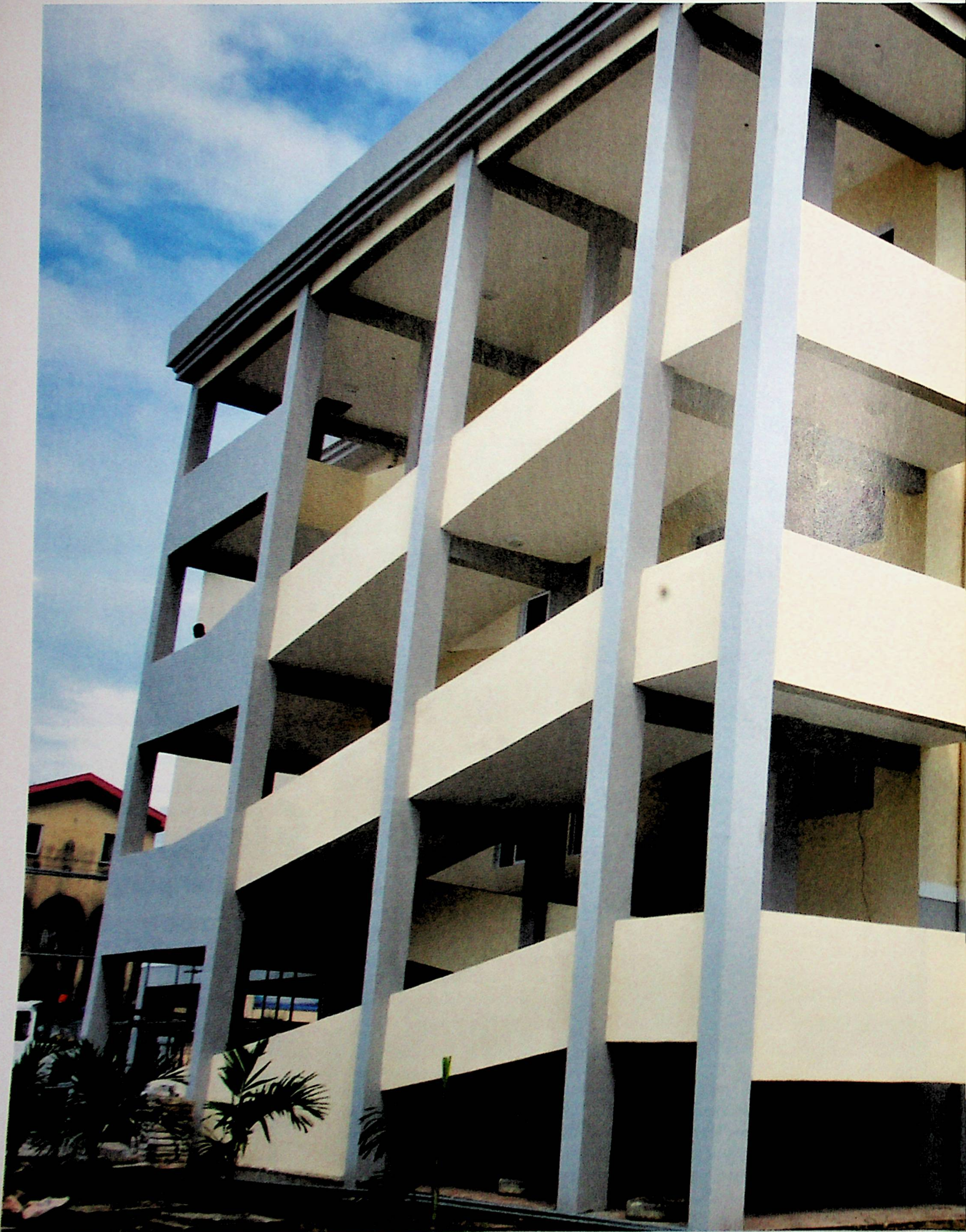
Kelsey Harrision Hospital, Port Harcourt
