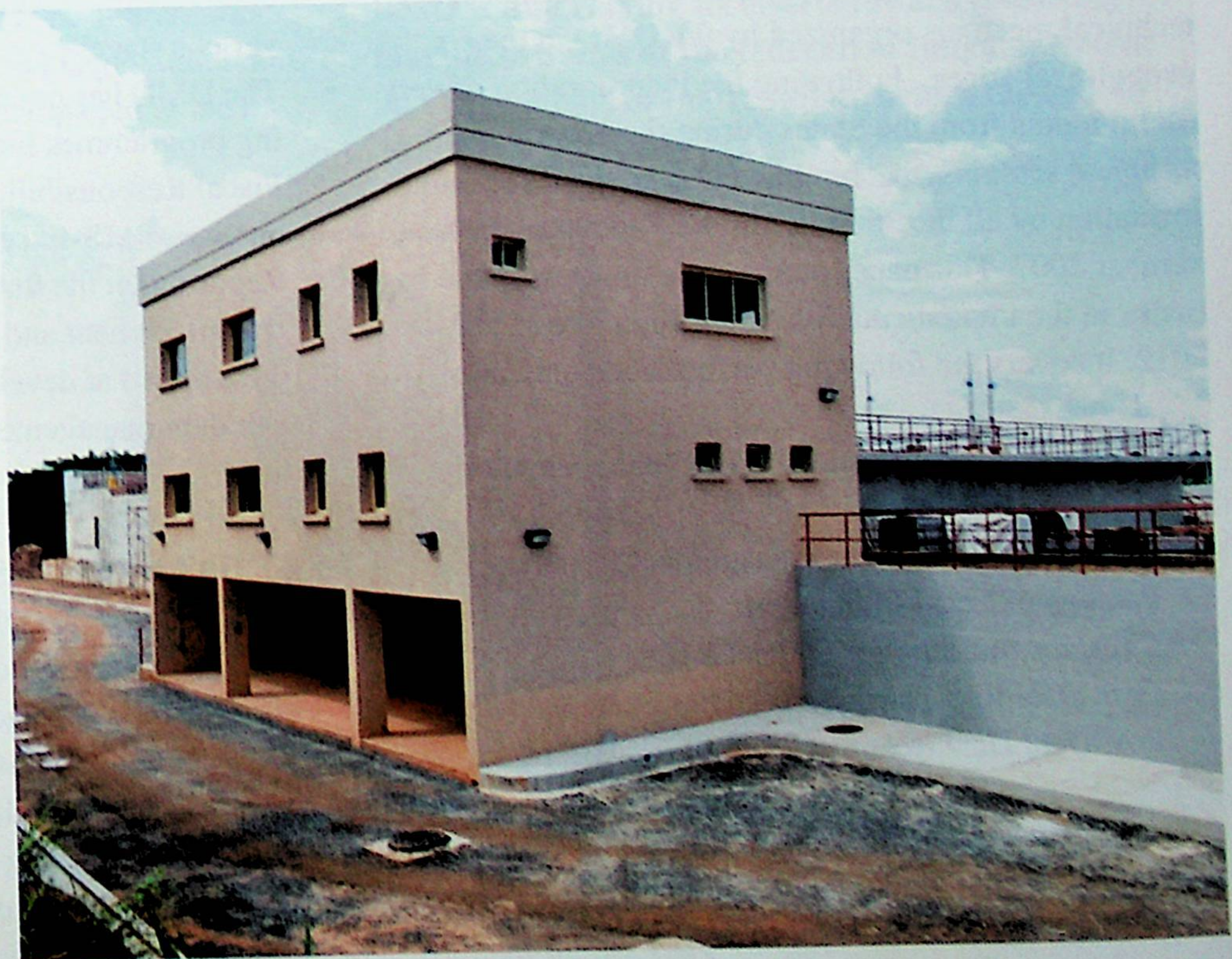
Greater Makurdi Water Works
