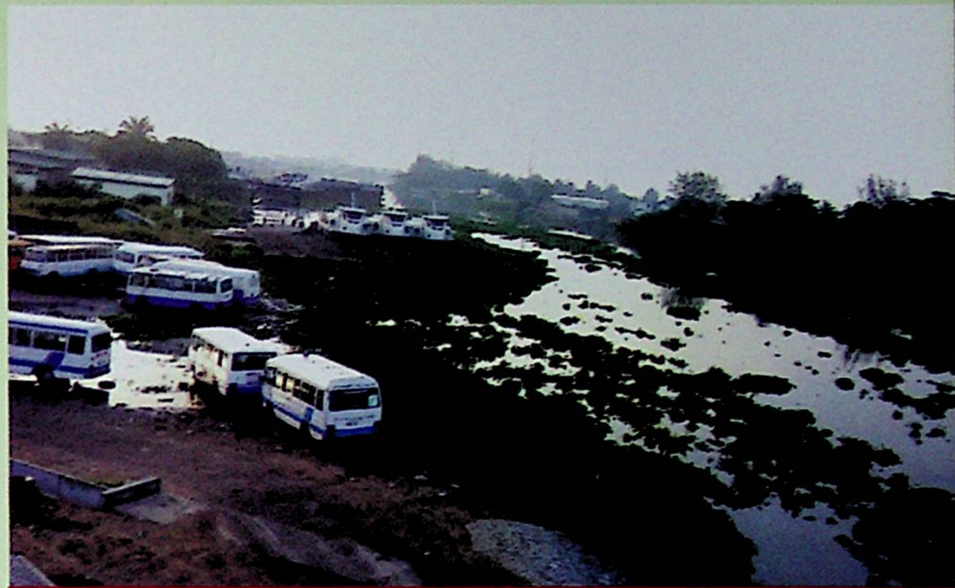
Mile 2 jetty covered by weeds
