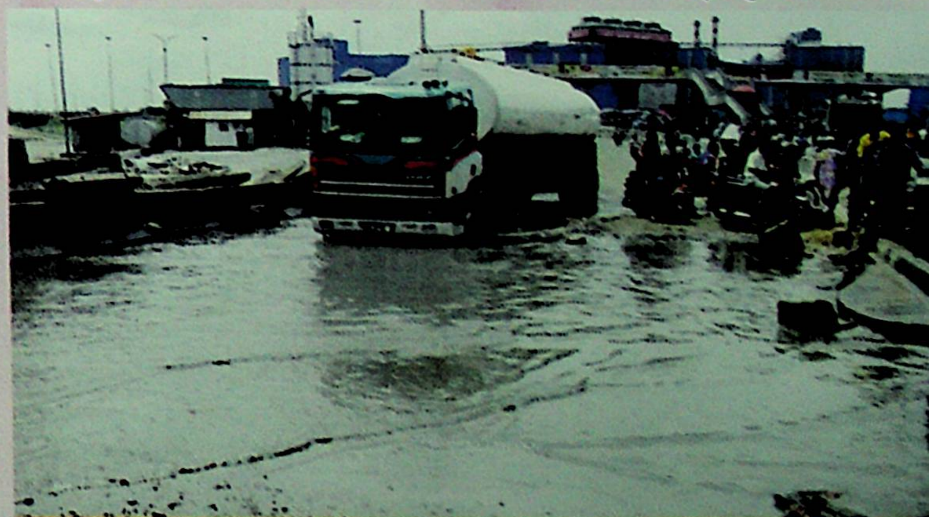
Permanent flood on a section of wharf road
