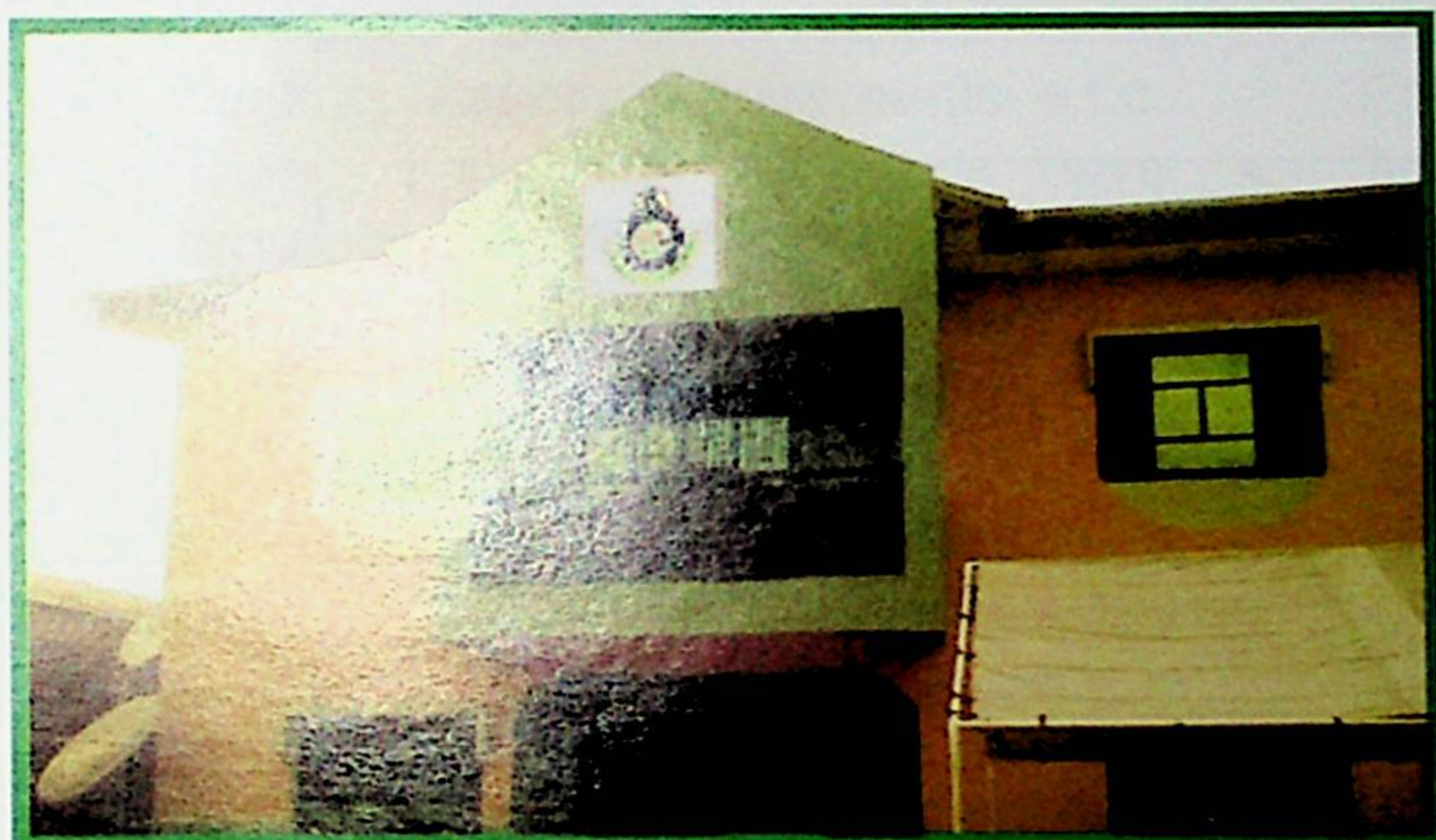
CENTRE'S FRONT VIEW
