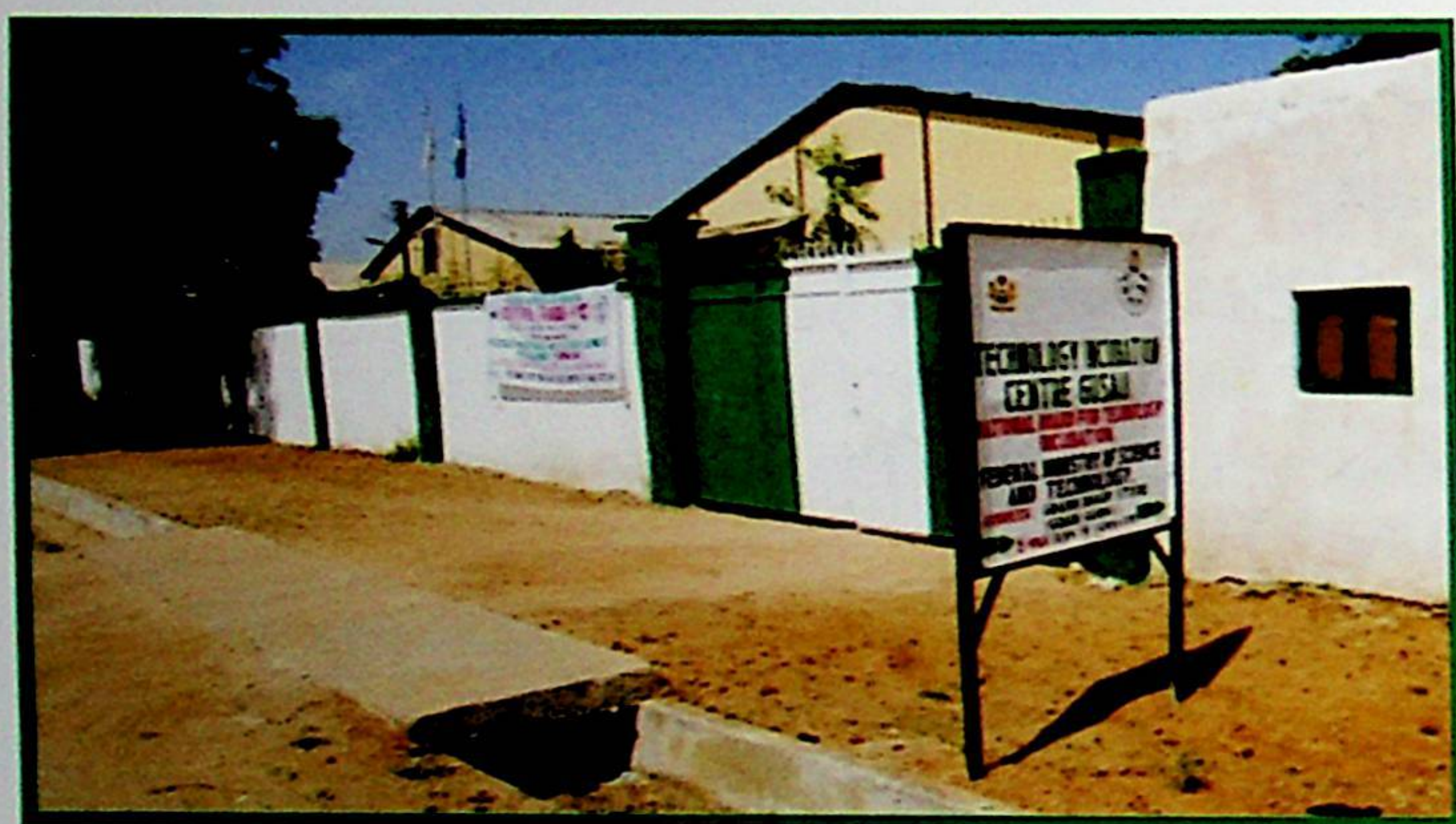
CENTRE'S FRONT VIEW
