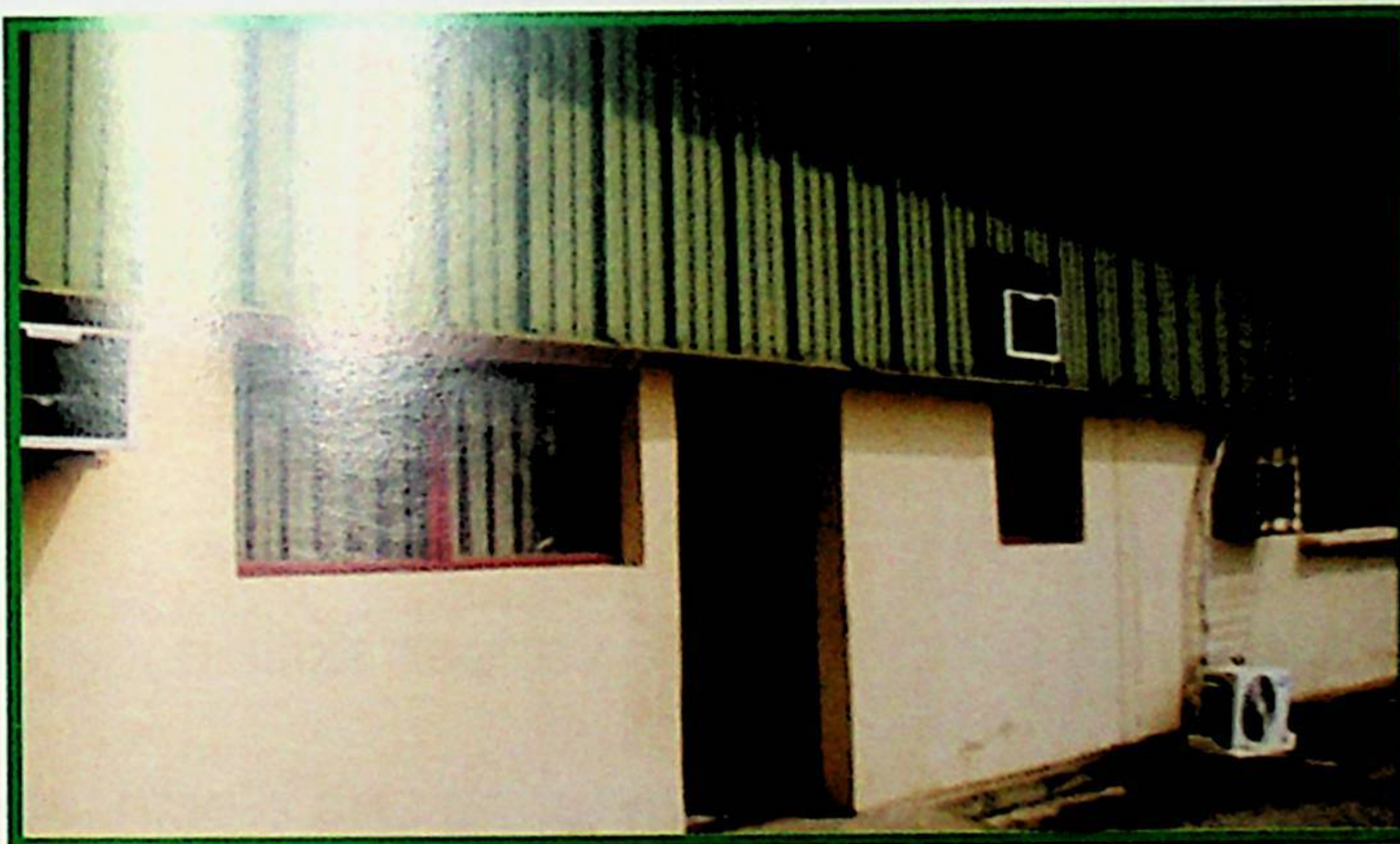
CENTRE'S FRONT VIEW
