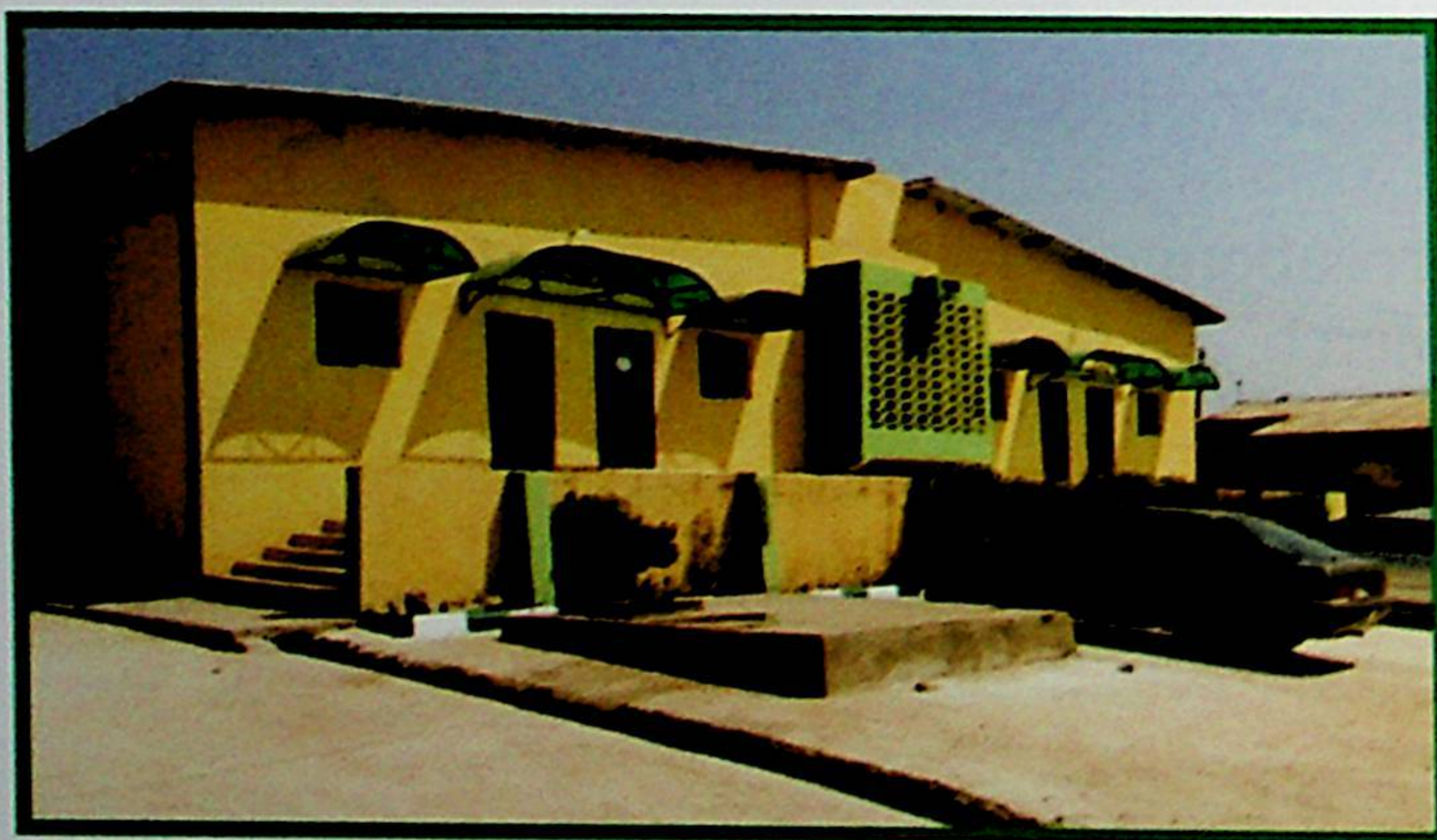
CENTRE'S FRONT VIEW
