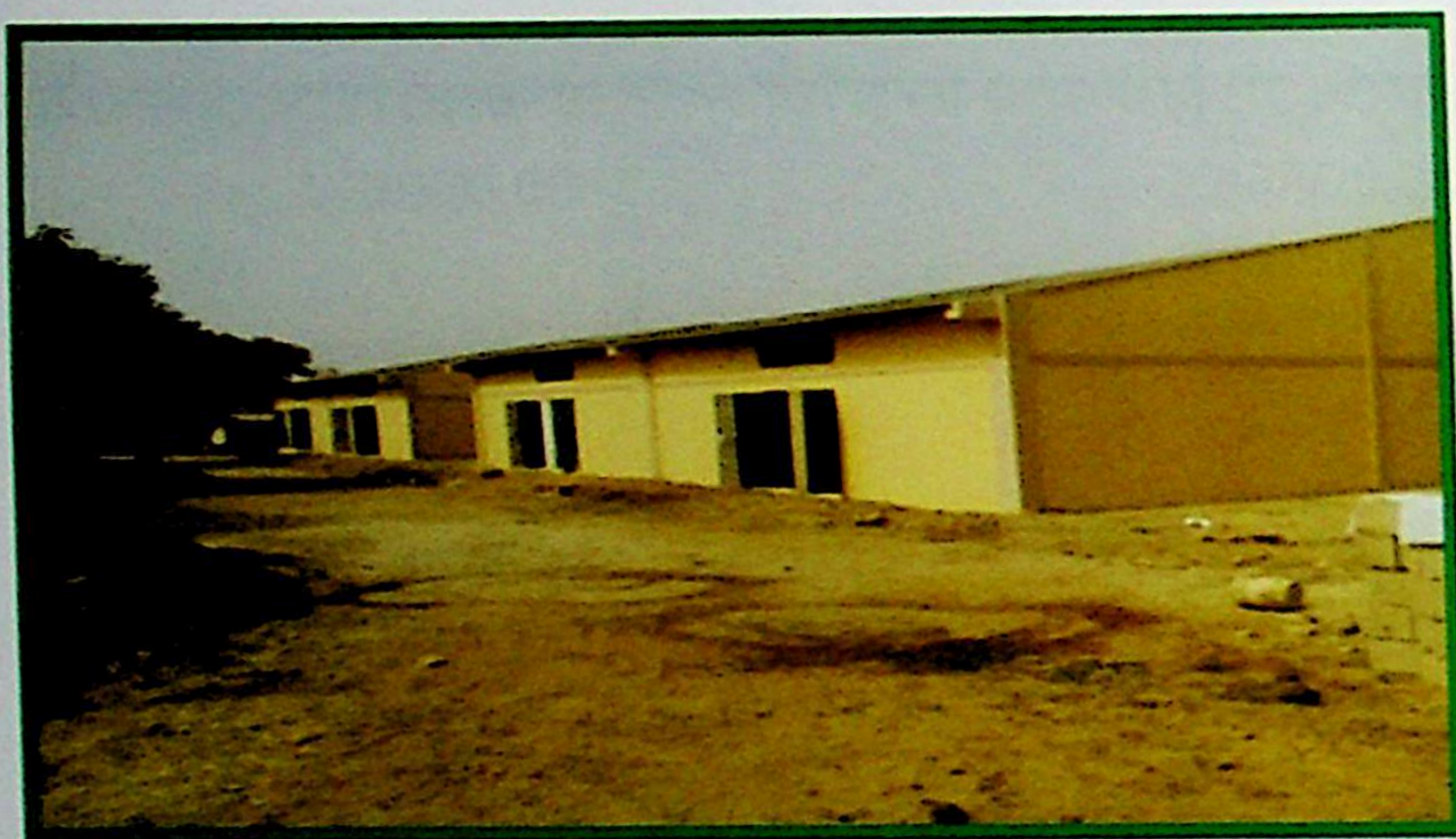
CENTRE'S FRONT VIEW
