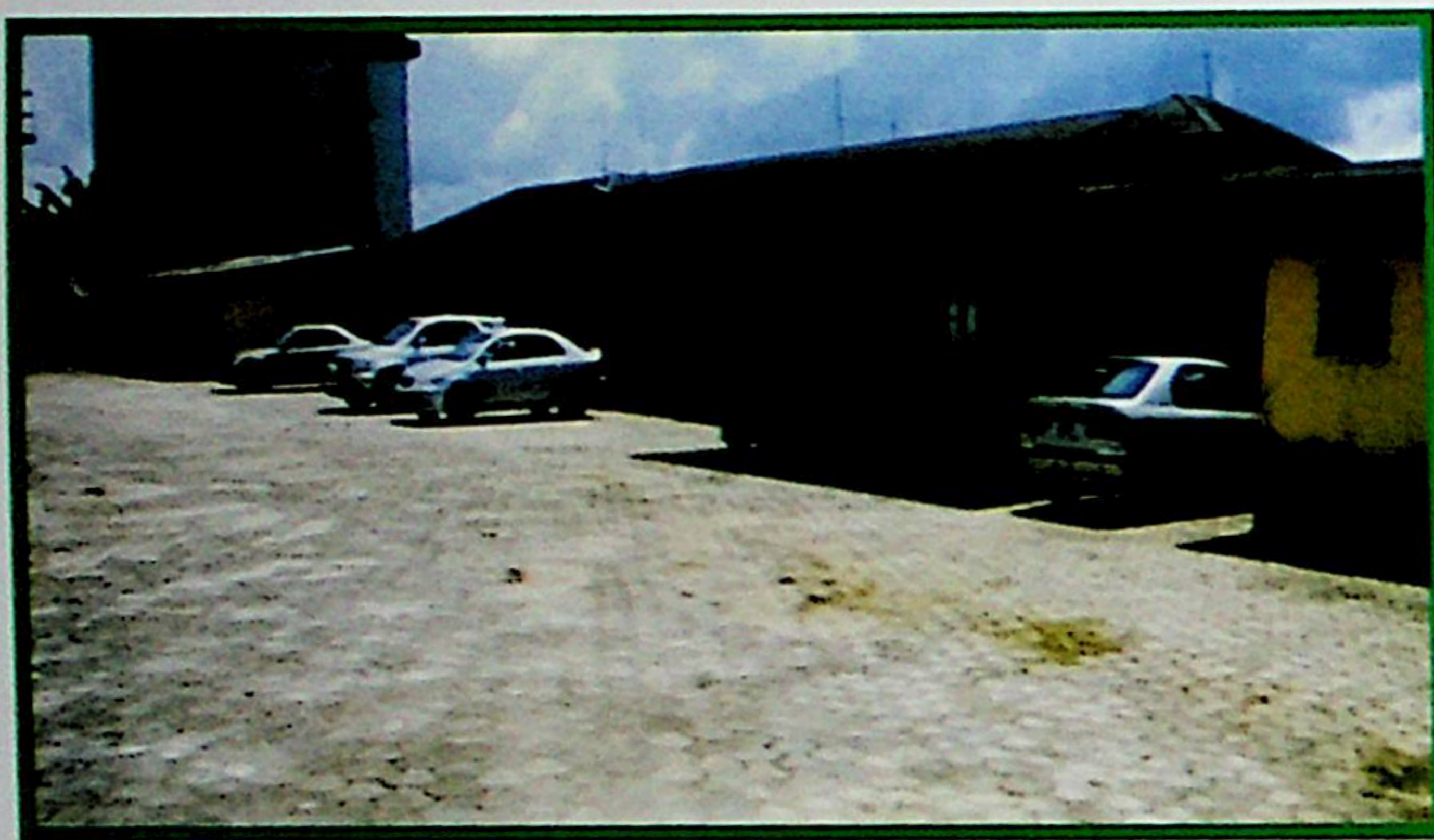
CENTRE'S FRONT VIEW
