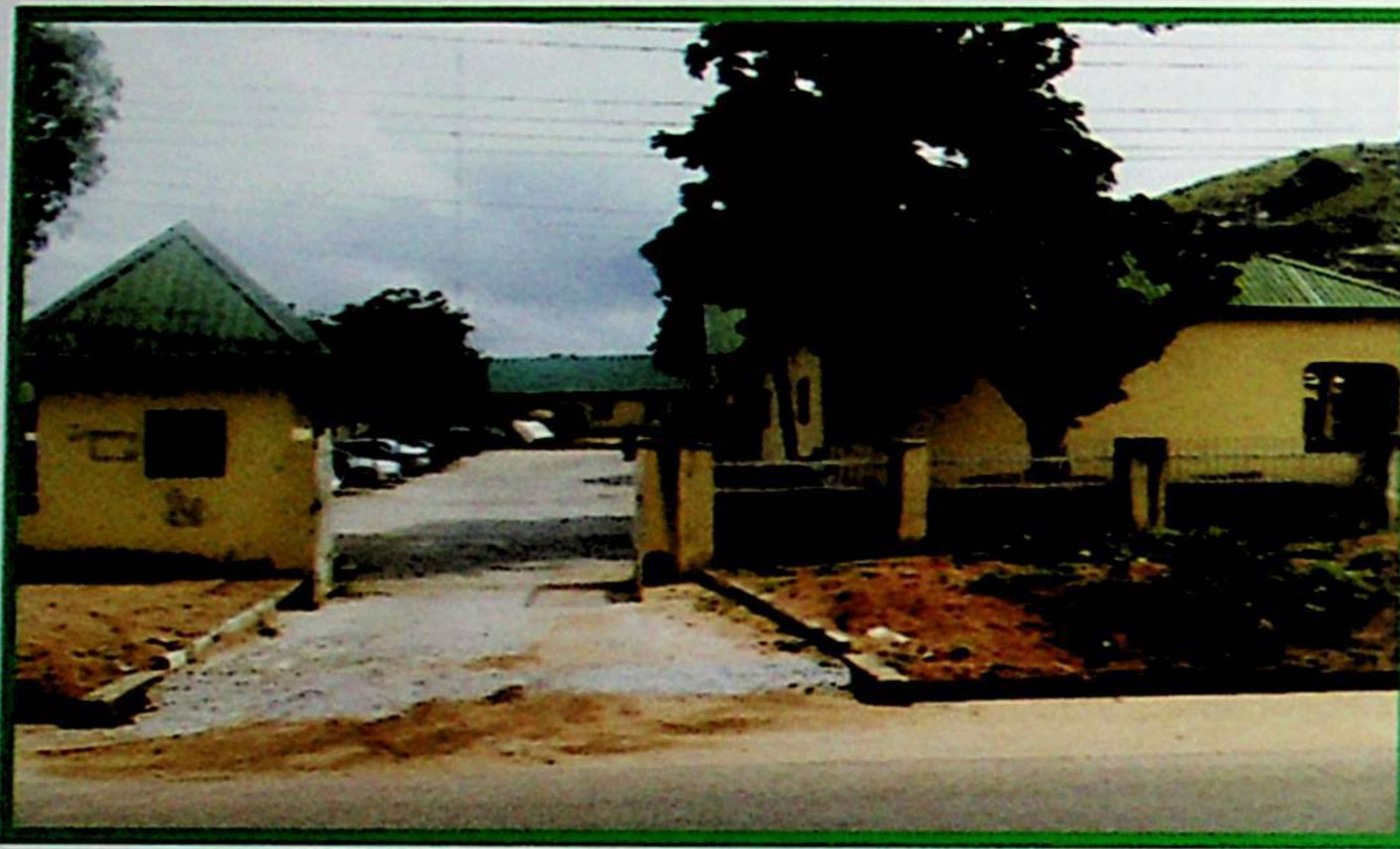
CENTRE'S FRONT VIEW
