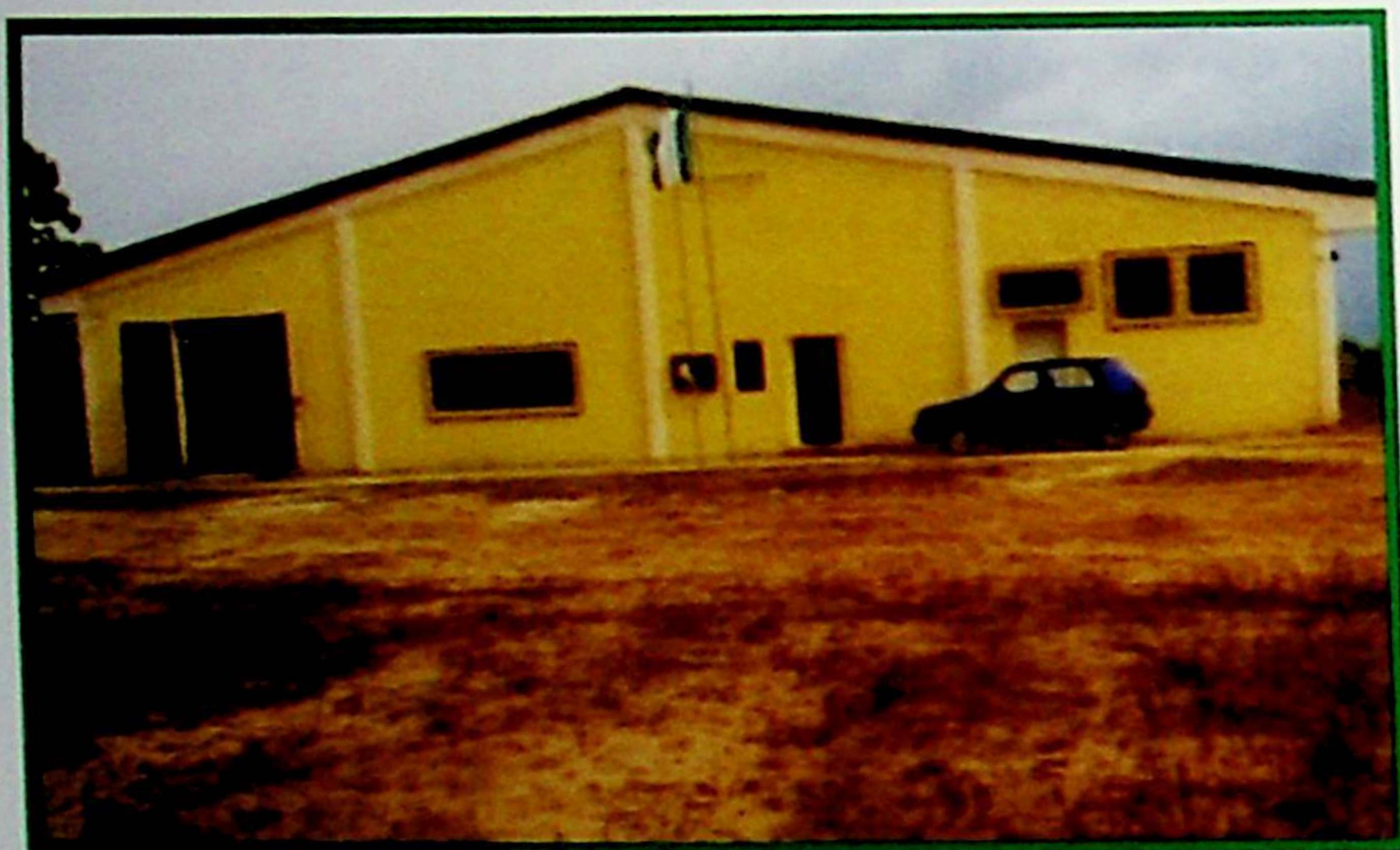
CENTRE'S FRONT VIEW
