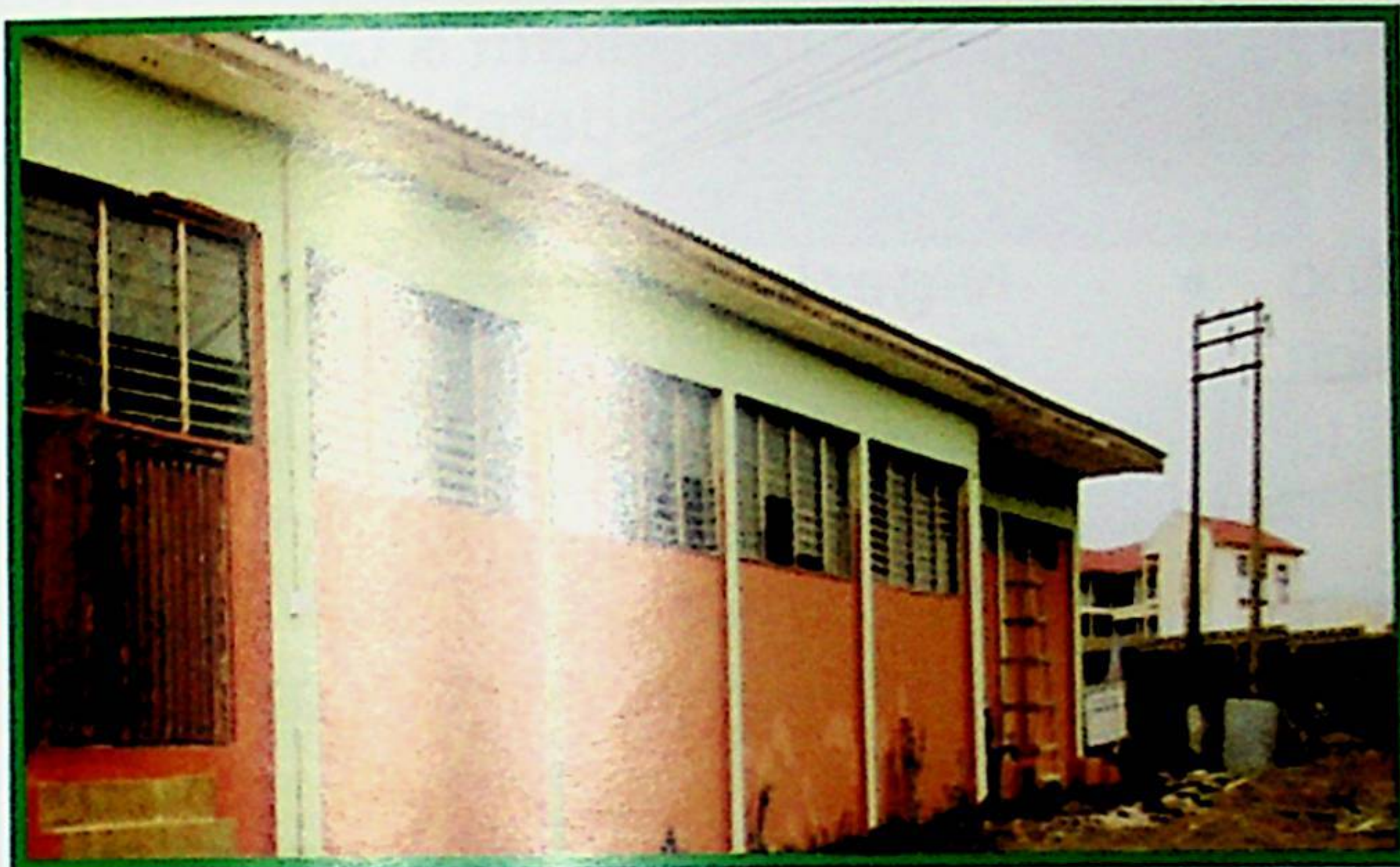
CENTRE'S FRONT VIEW
