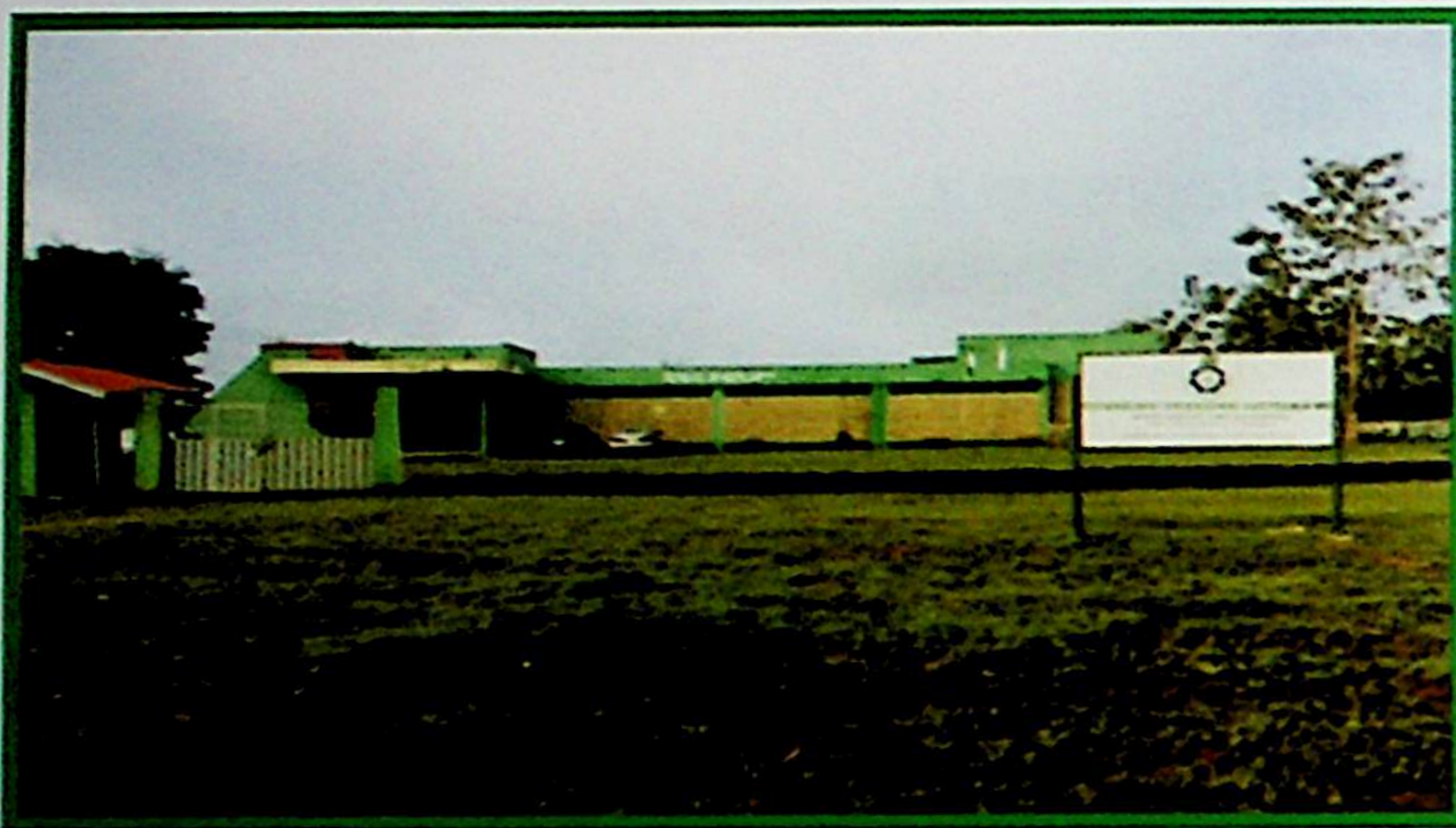
CENTRE'S FRONT VIEW
