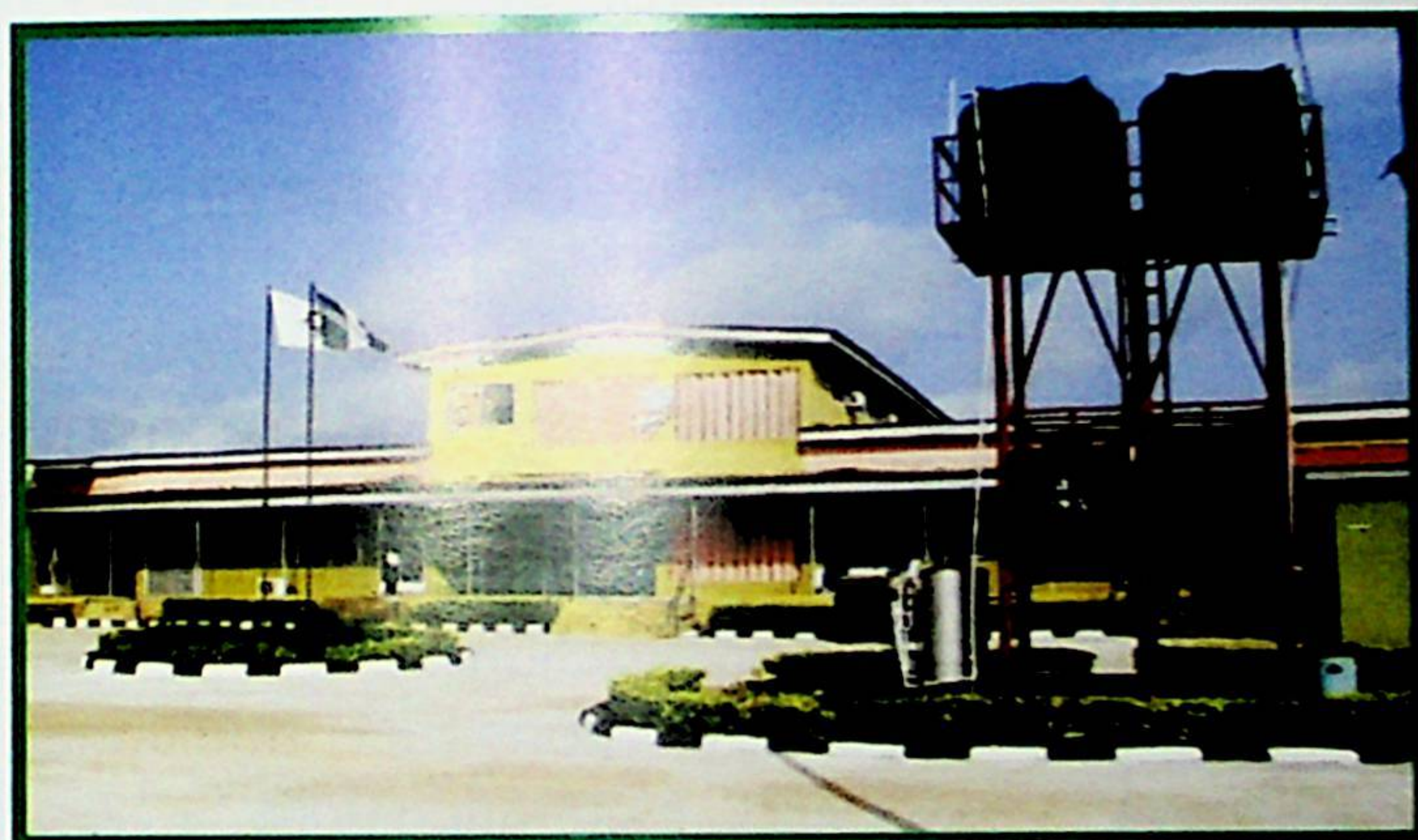
CENTRE'S FRONT VIEW
