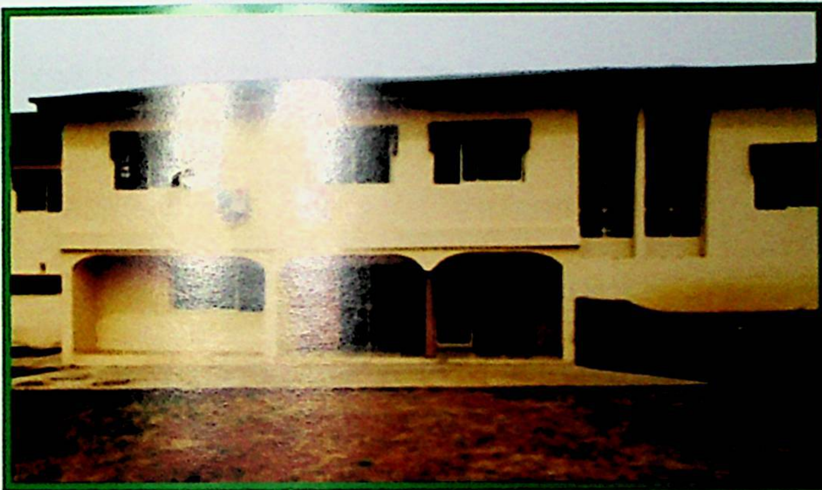
FRONT VIEW OF ADMINISTRATIVE BLOCK
