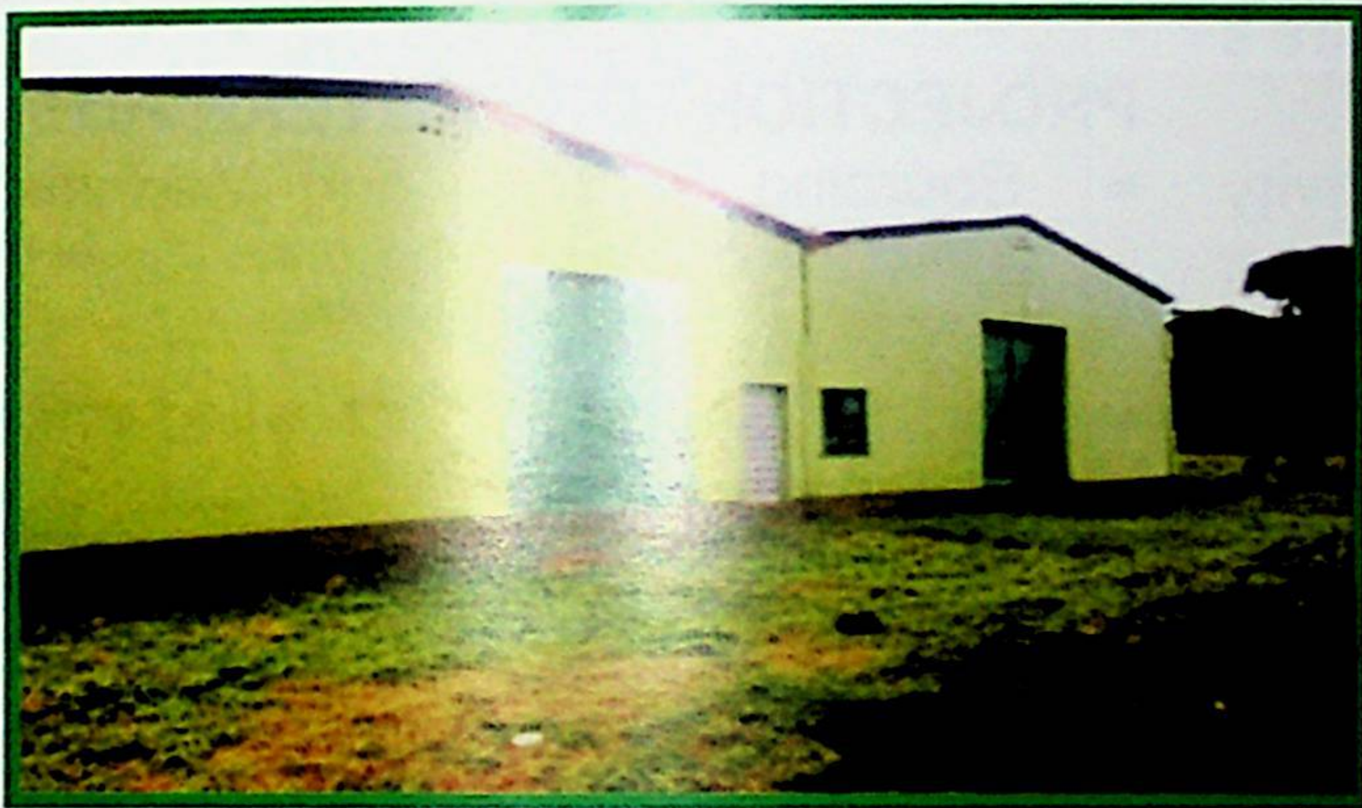
CENTRE'S FRONT VIEW
