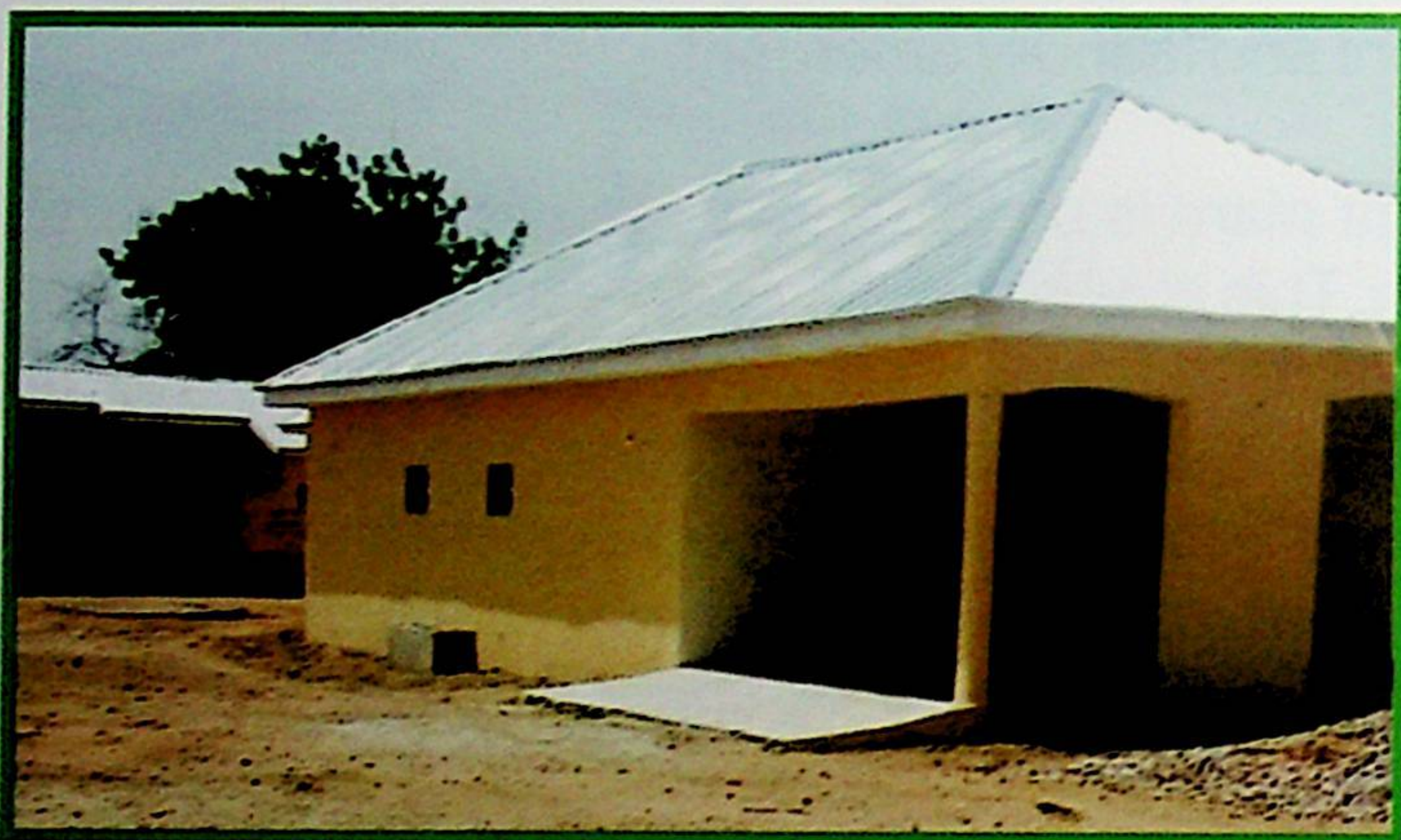
CENTRE'S FRONT VIEW
