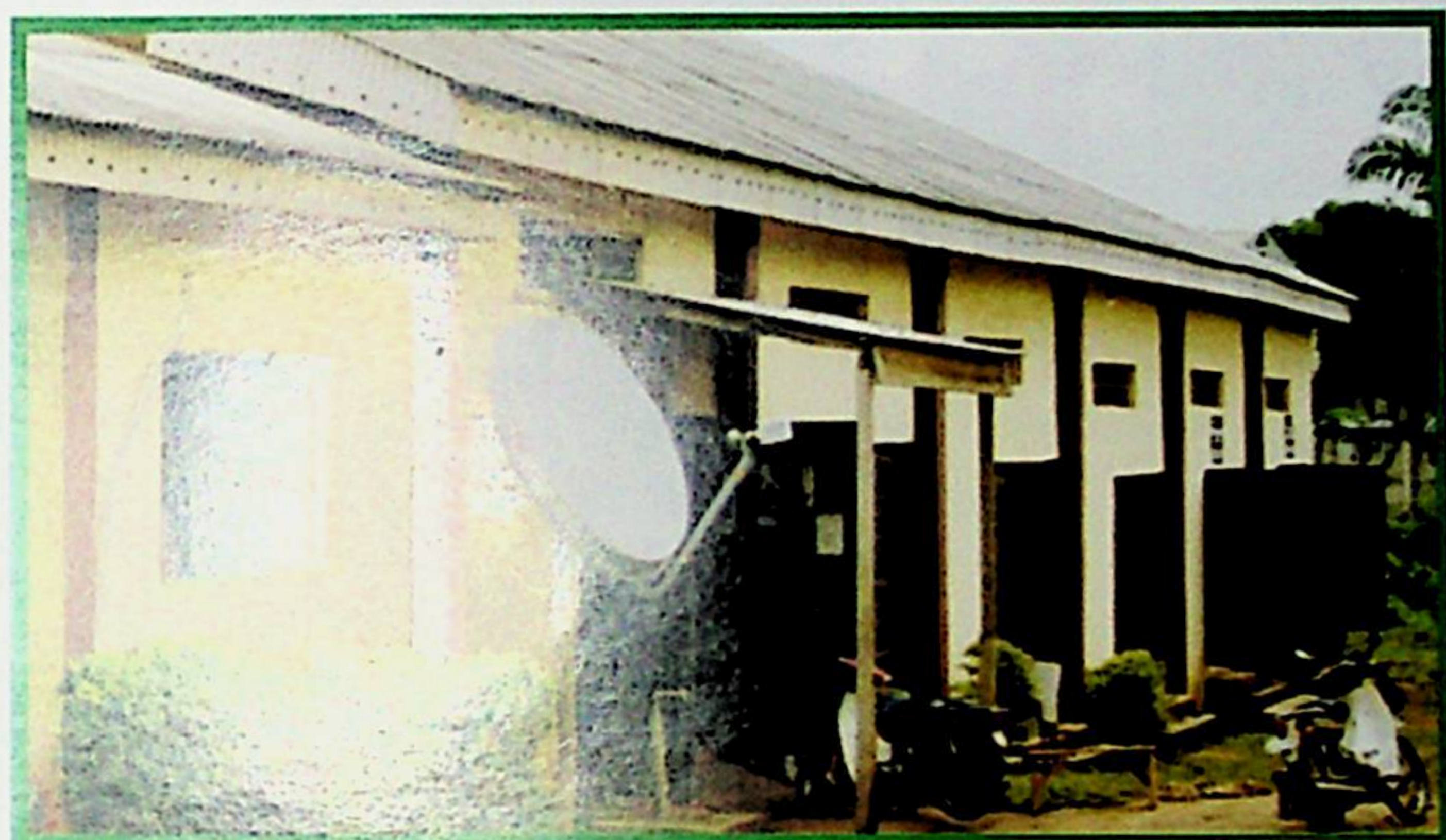
CENTRE'S FRONT VIEW
