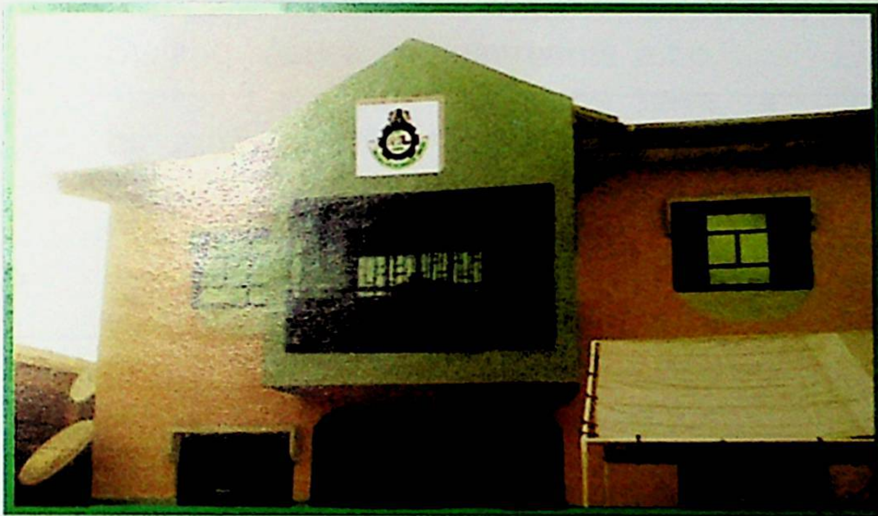
CENTRE'S FRONT VIEW
