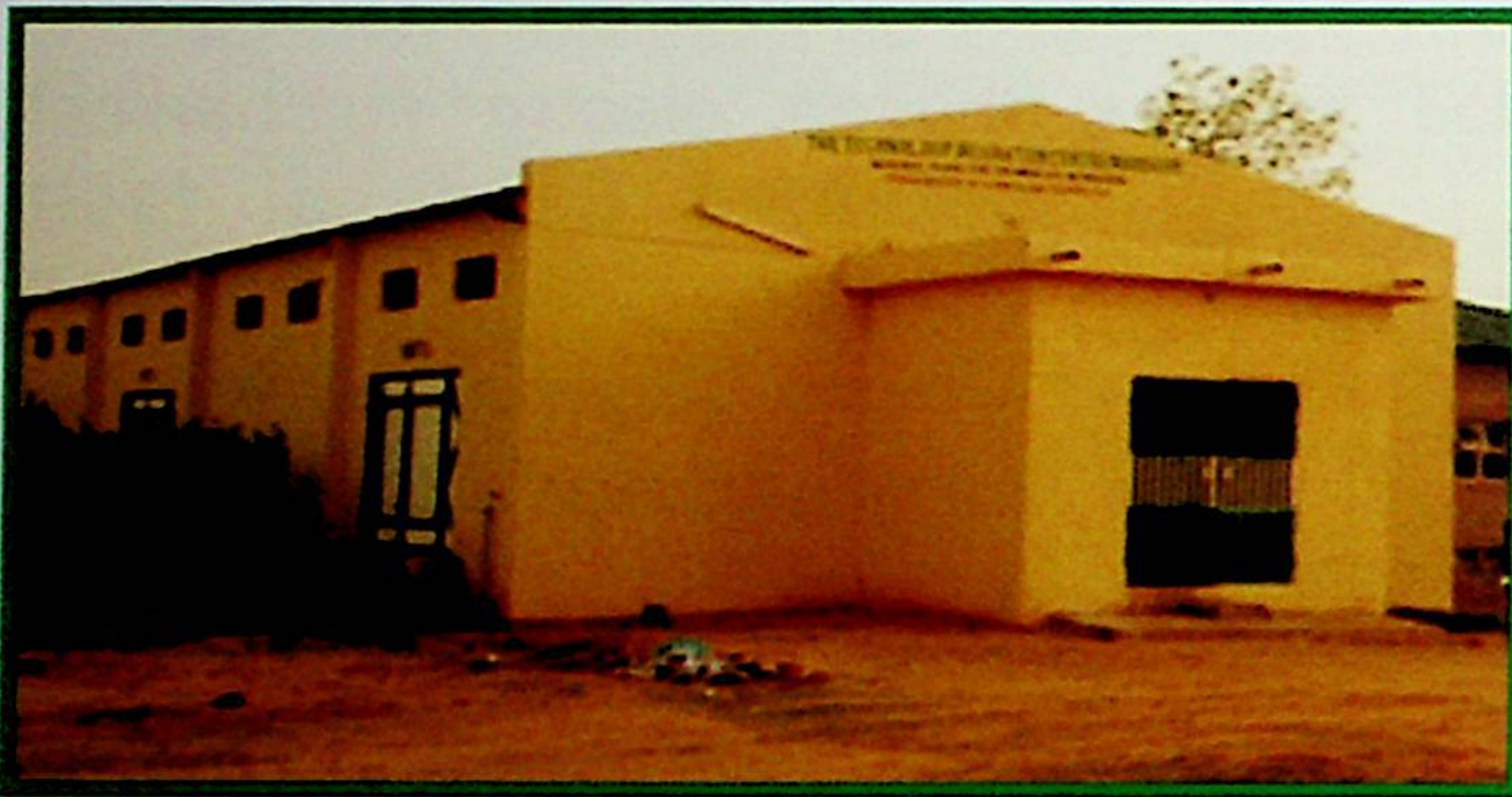
CENTRE'S FRONT VIEW
