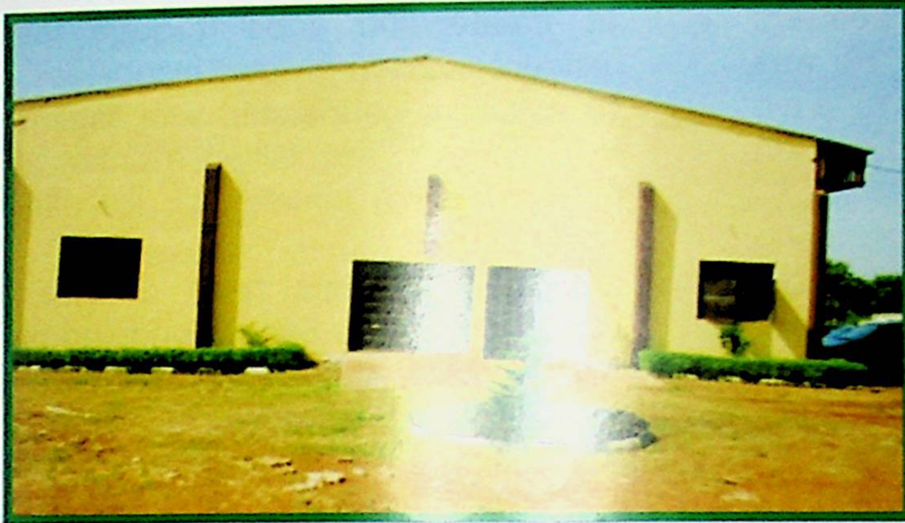
CENTRE'S FRONT VIEW
