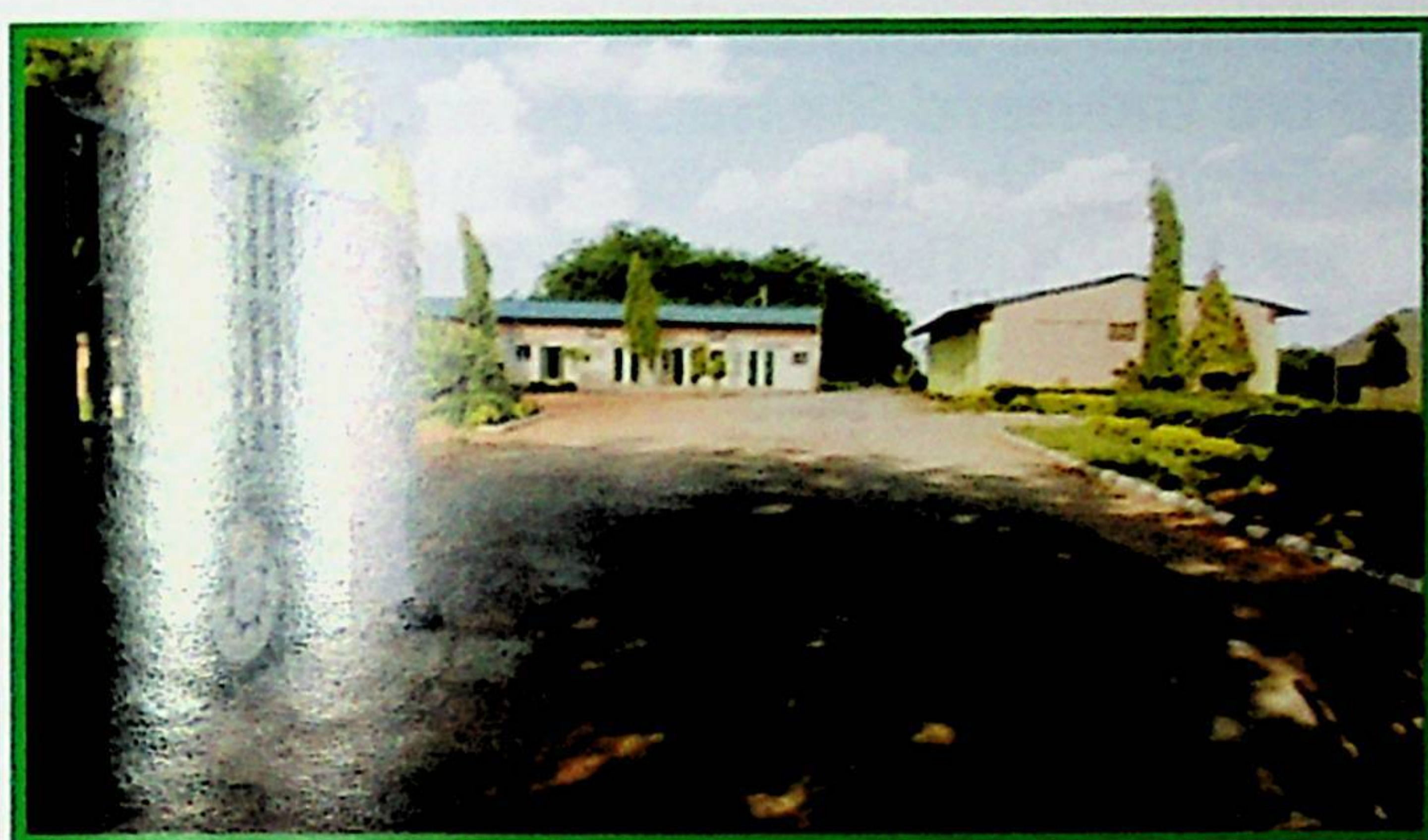
CENTRE'S FRONT VIEW
