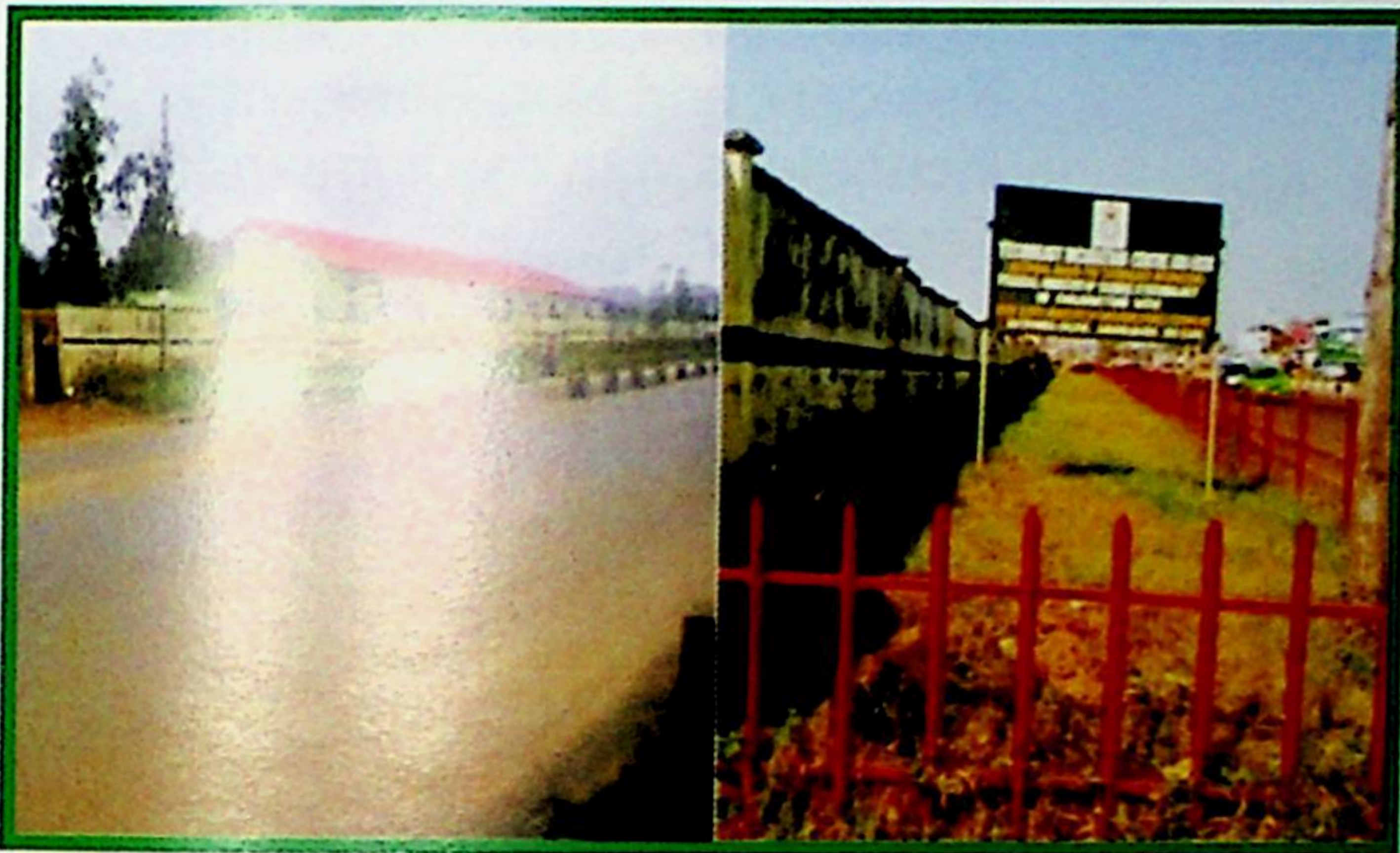
CENTRE'S FRONT VIEW
