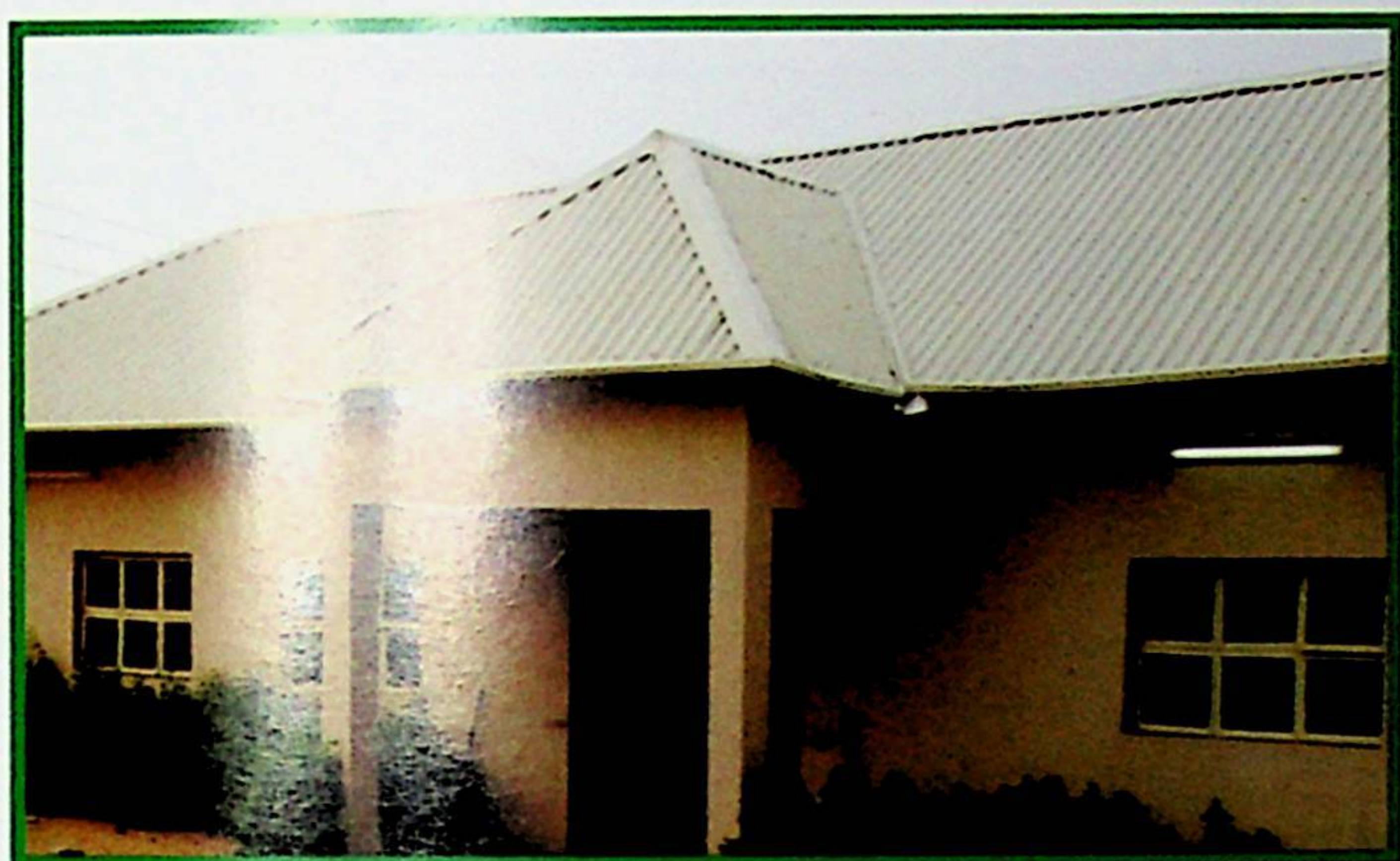
CENTRE'S FRONT VIEW
