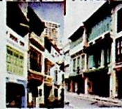
BOAT QUAY RESTORATION (13 UNITS)
