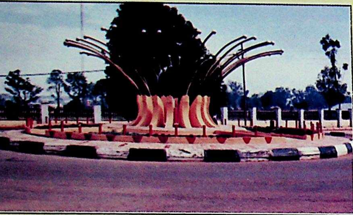
One of the rehabilitated roundabouts in Jos and Bukuru metropolis.
