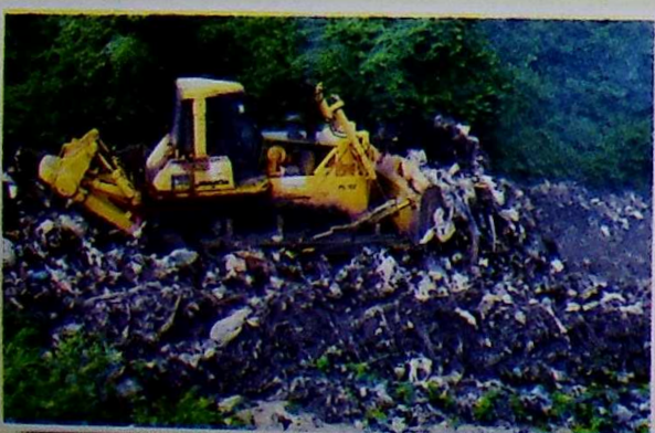
Clearing of Dump Site at Saje (during clearing)
