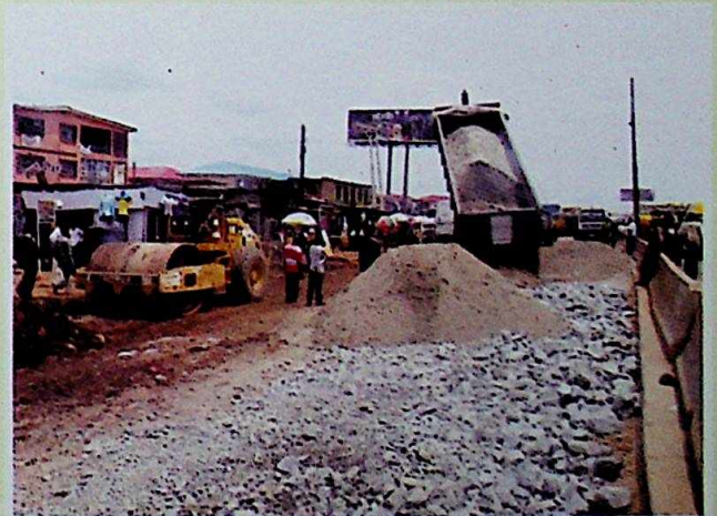
Lagos-Abeokuta Expressway Road During Rehabilitation
