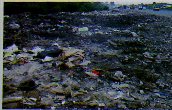
Clearing work in Progress at Iseri-Ibafo
