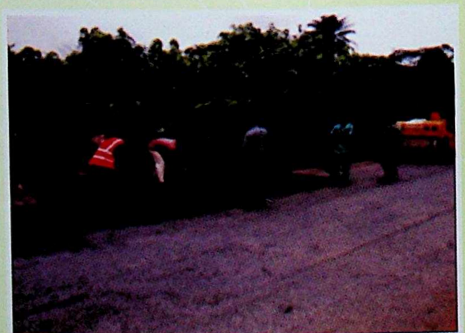
Abeokuta - Sagamu Expressway (During rehabilitation)
