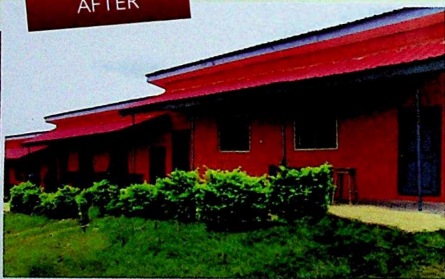
The Newly Renovated Block 'B' of Four (4) Class Room Salvaged from total Collapse, at Co-operative College, Ijeja - Abeokuta
