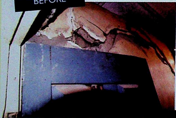
Entrance of the Student Toilet
