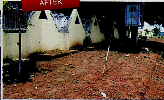
The Governor's Entrance Office After Clearing
