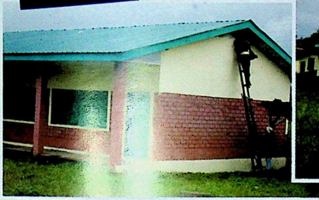
Newly Completed Classroom
