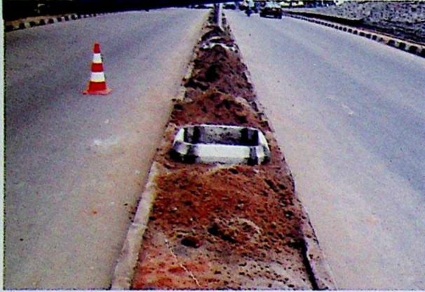
LandScaping, Beutification work in progress at Ibara Road
