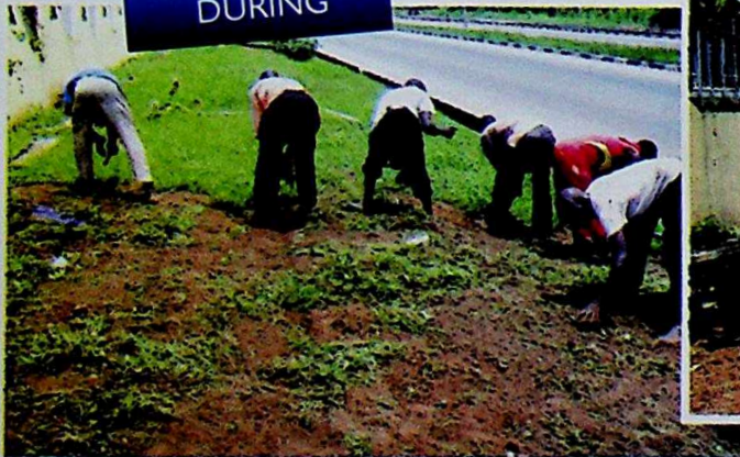
The Governor's Entrance Office During Clearing
