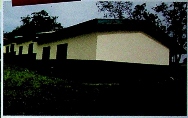
Newly Completed Classroom
