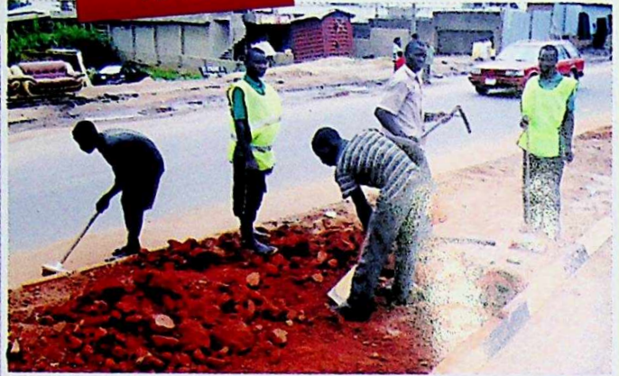
LandScaping, Beutification work in progress at Ibara Road
