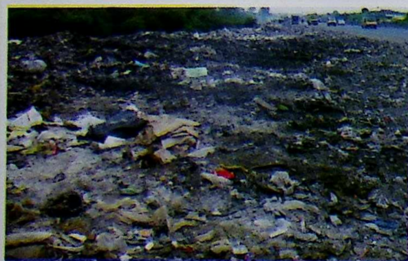
Clearing work in Progress at Iseri-Ibafo
