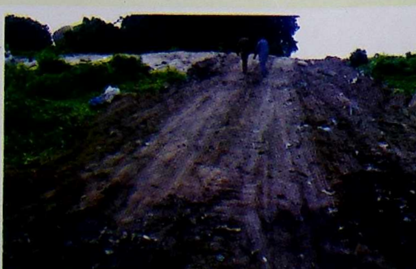
Clearing of Dump Site at Saje (After Clearing)
