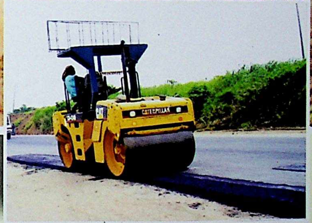
Lagos-Ibadan Expressway (During Rehabilitation)
