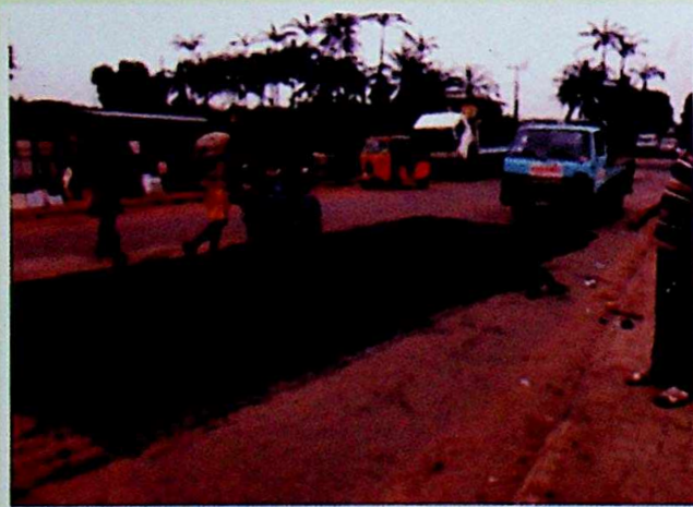
Ejirin Road Ijebu-Ode (During rehabilitation)
