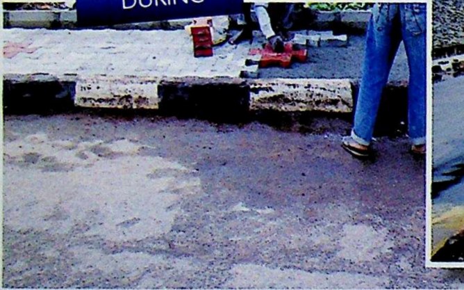
Landscaping Beautification at Isale Igbein- Sapon, Abeokuta (Work in Progress)
