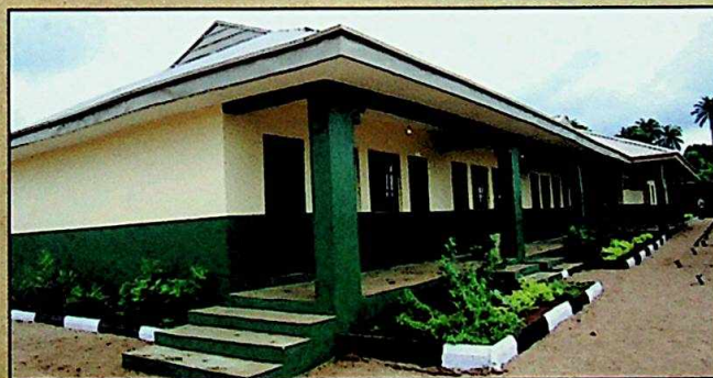
Commissioning of A block of Classrooms donated by Property Mart Real Estate Ltd to the State Govt. by SSG
