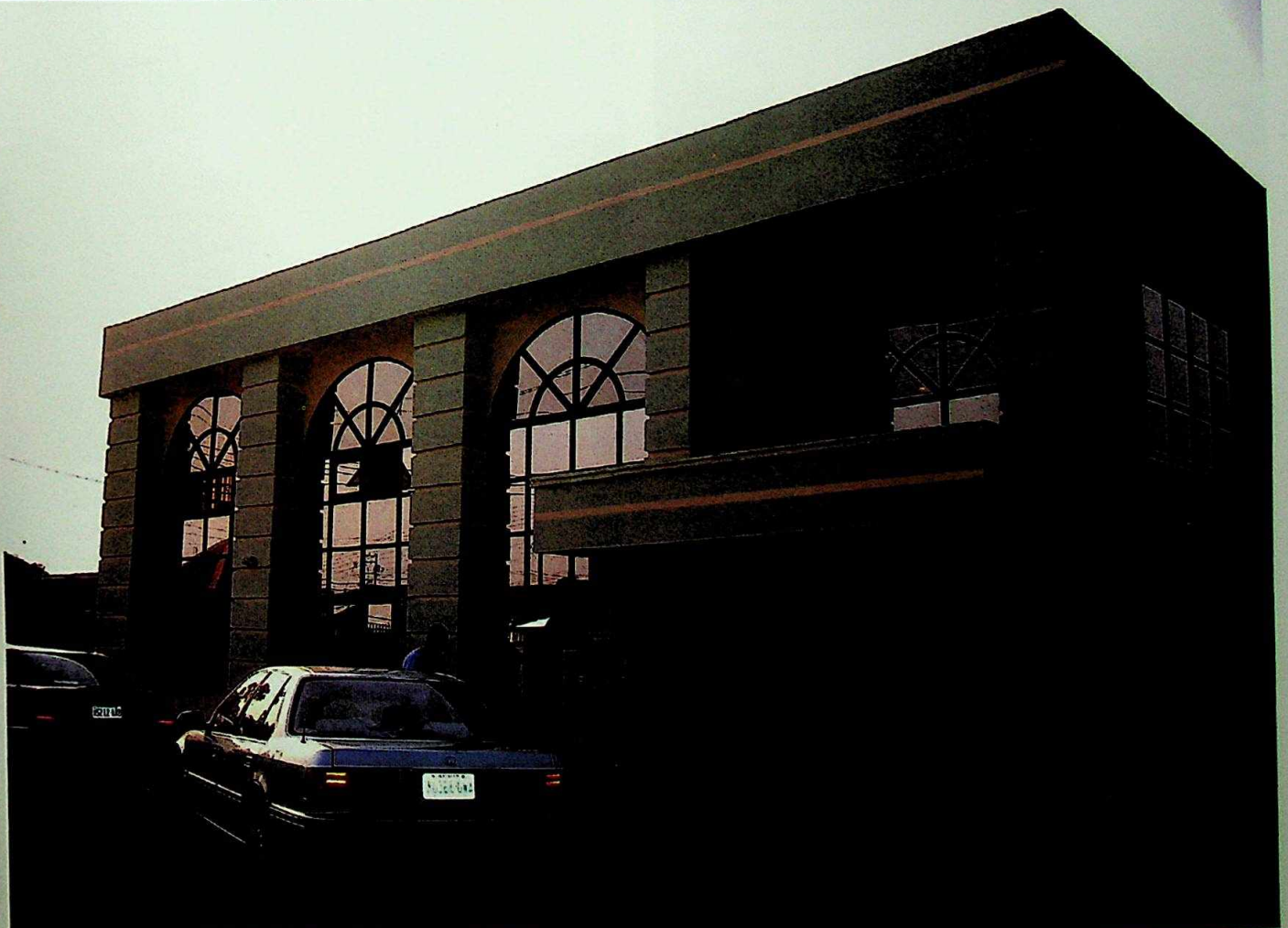
NEW GATEWAY SAVINGS AND LOANS...IN AID OF SHELTER FOR ALL
