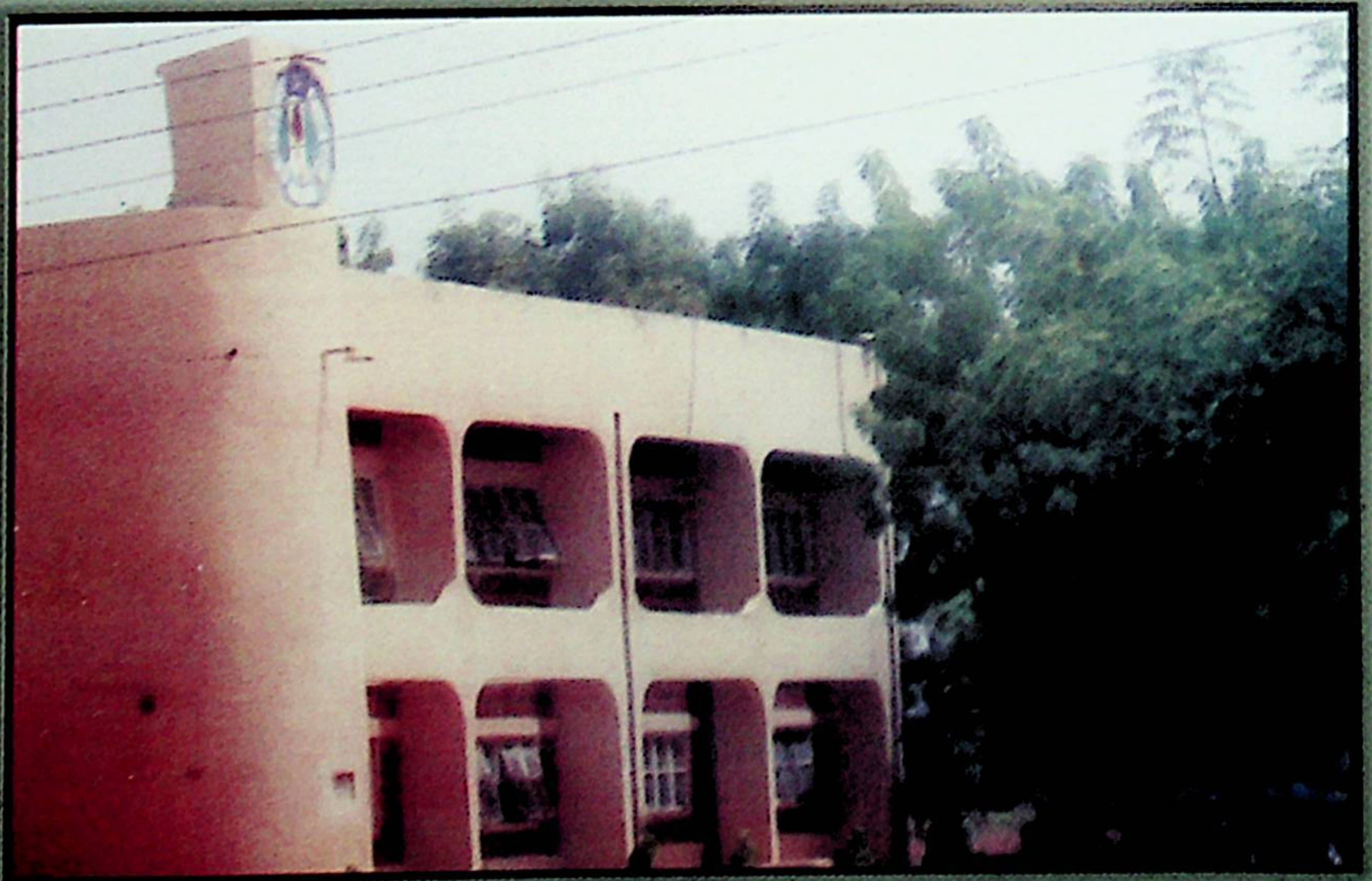
College of Education Azare fully renovated and upgraded by the Administration of Malam Isa Yuguda.
