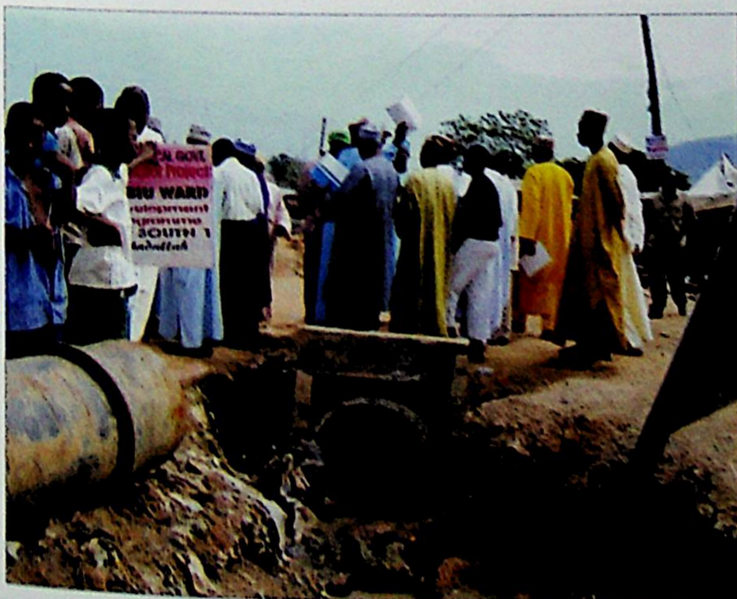
Completed Ring Culvert at Madalla in Iku South 1 Ward
