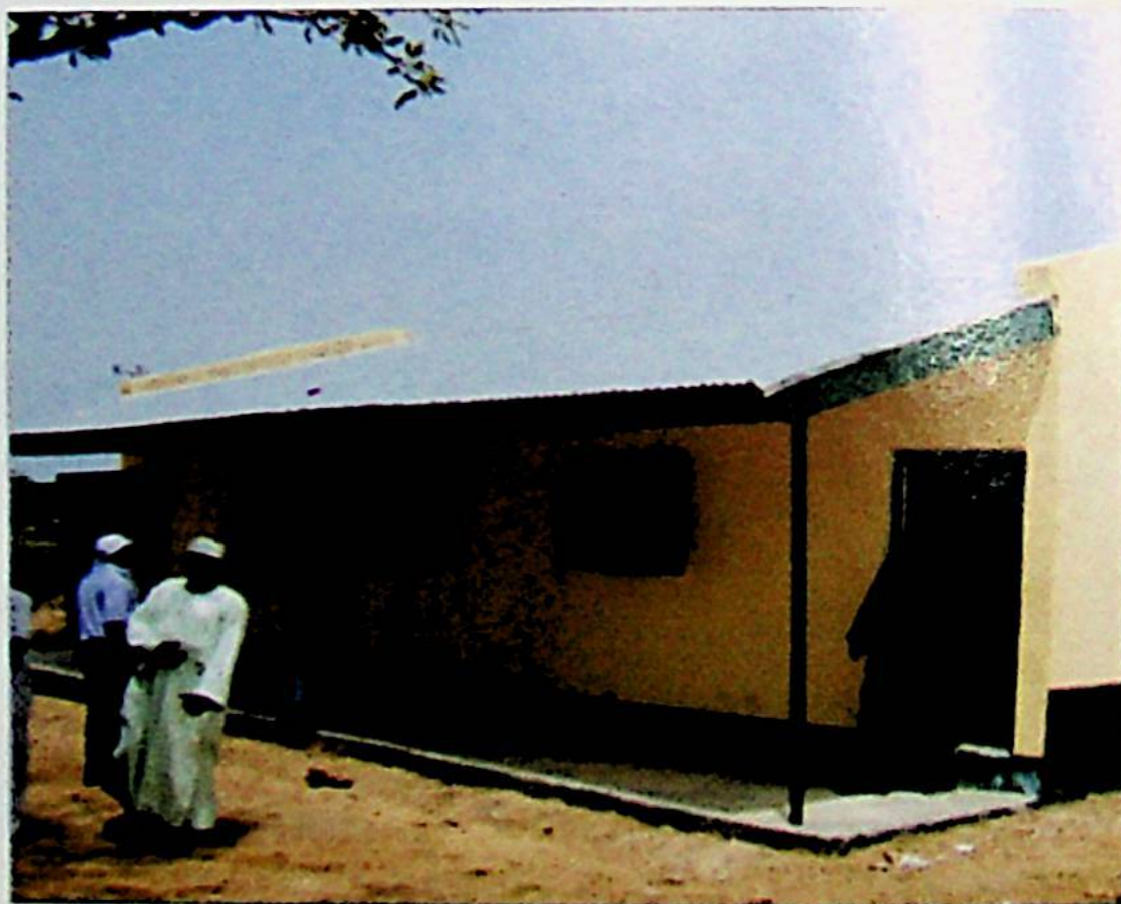
Constructed 1 Block of 2 Classrooms at Gallah Ward
