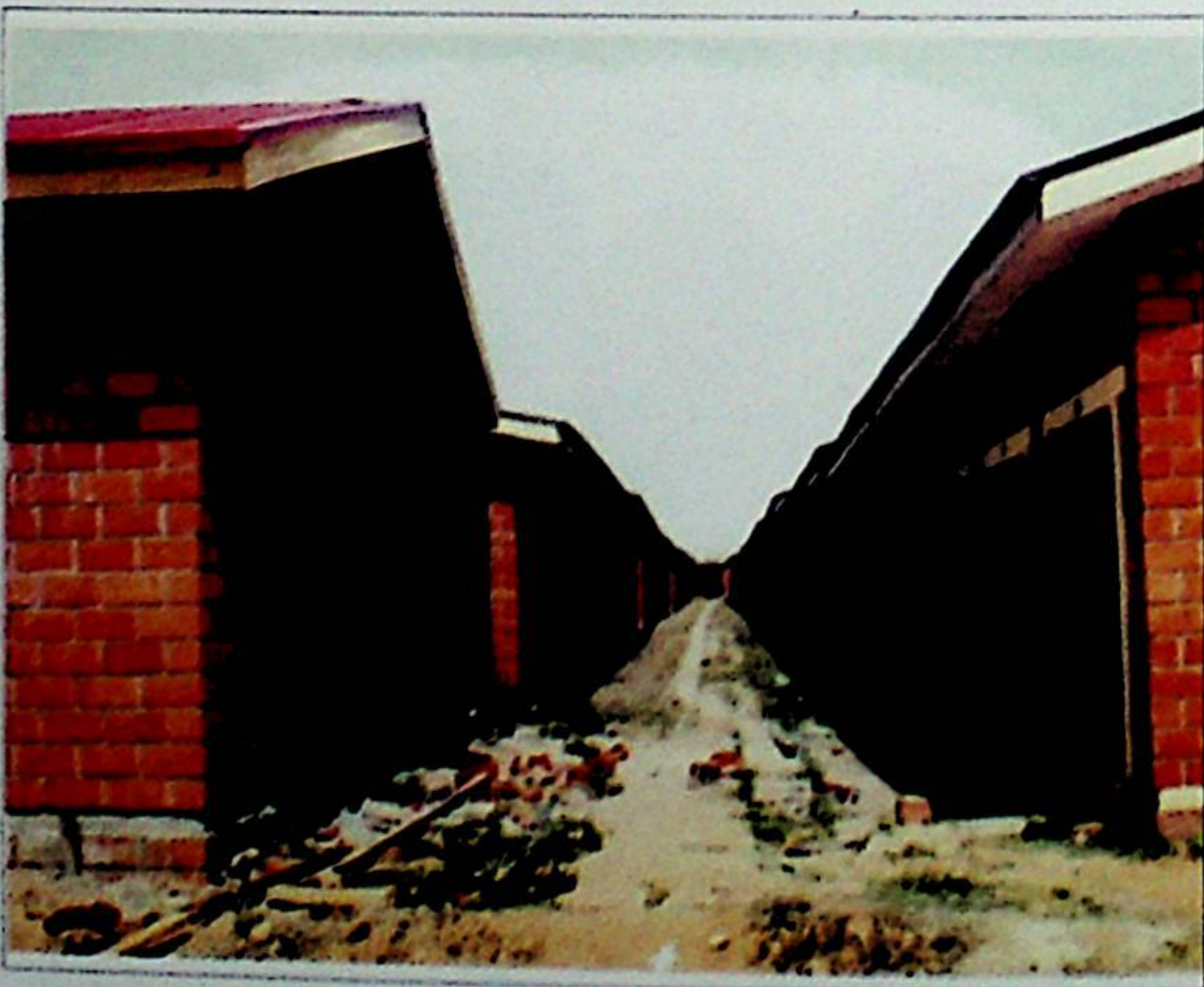
Ongoing construction work Ultra Modern Market
