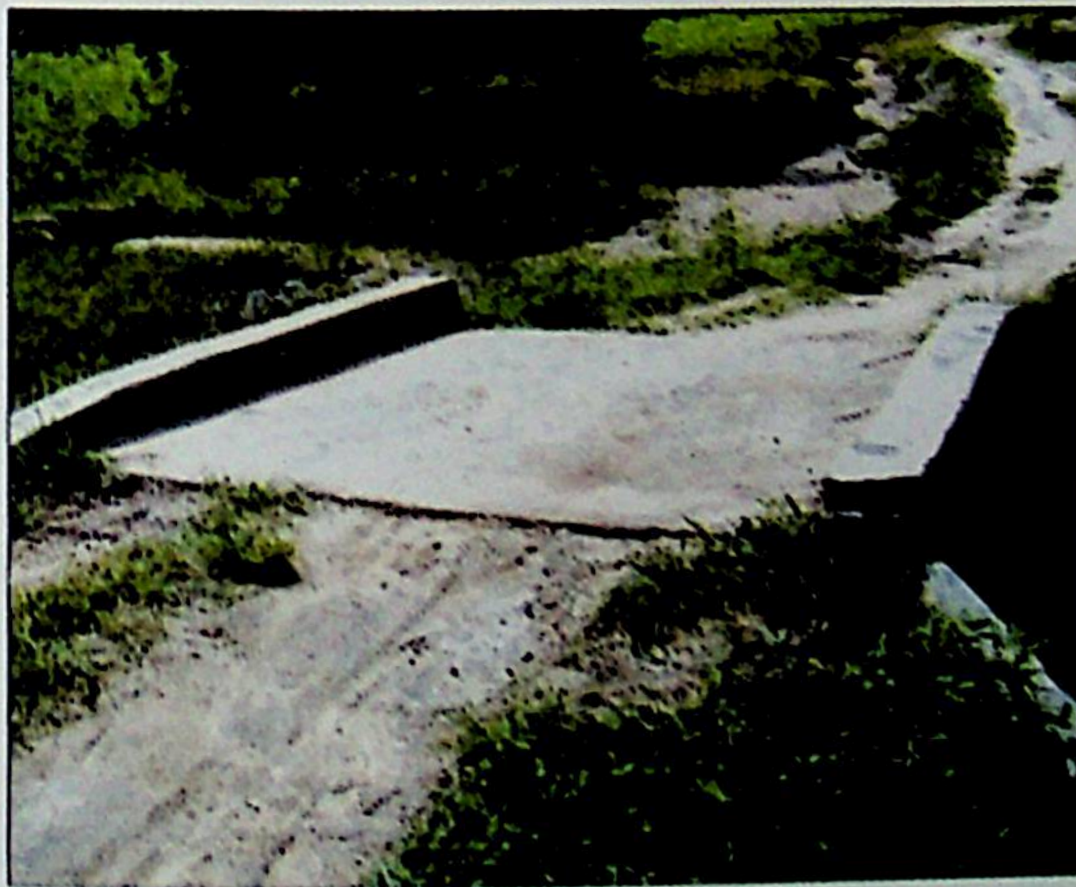
Constructed Culvert at Essa Village in Essa Ward
