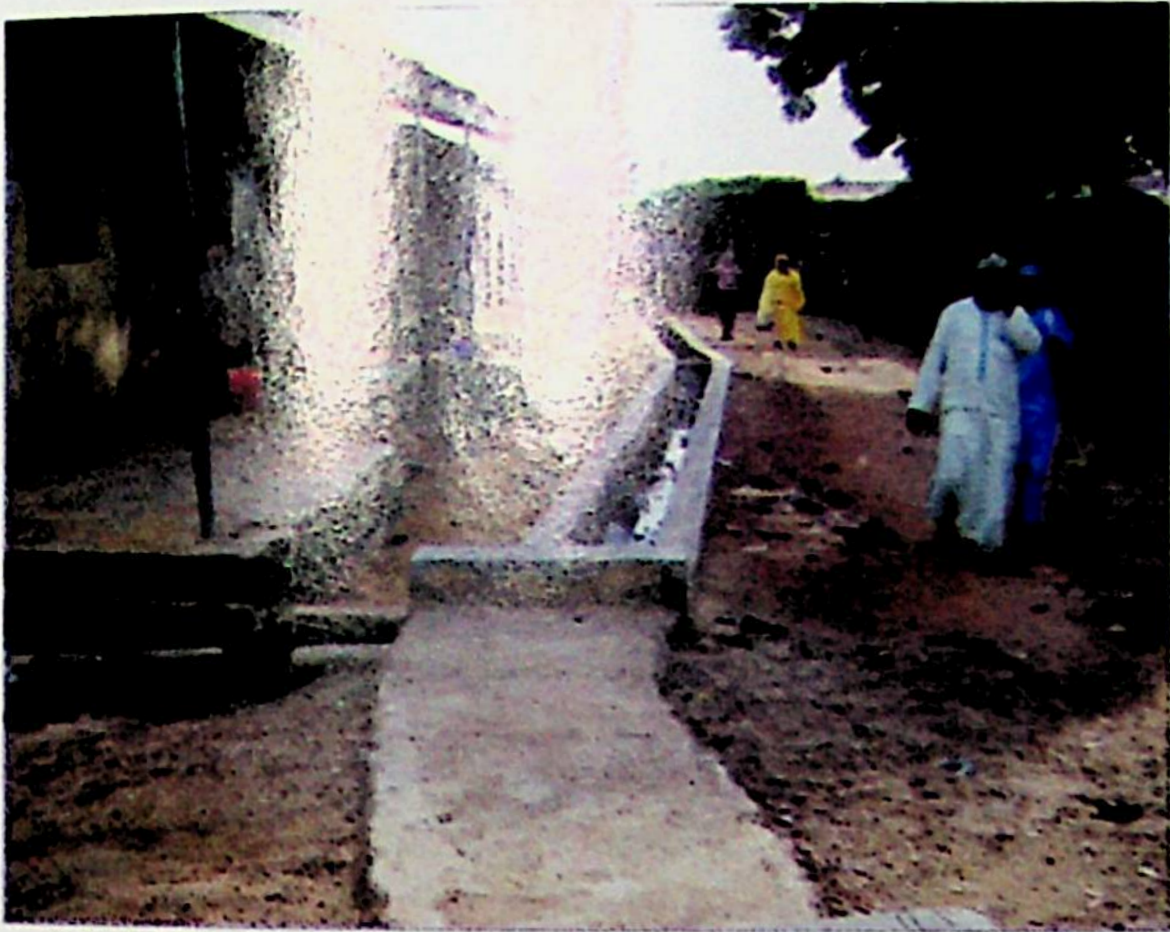
Construction of Culvert and drainage at Tunga in Tudun-Wada North Ward
