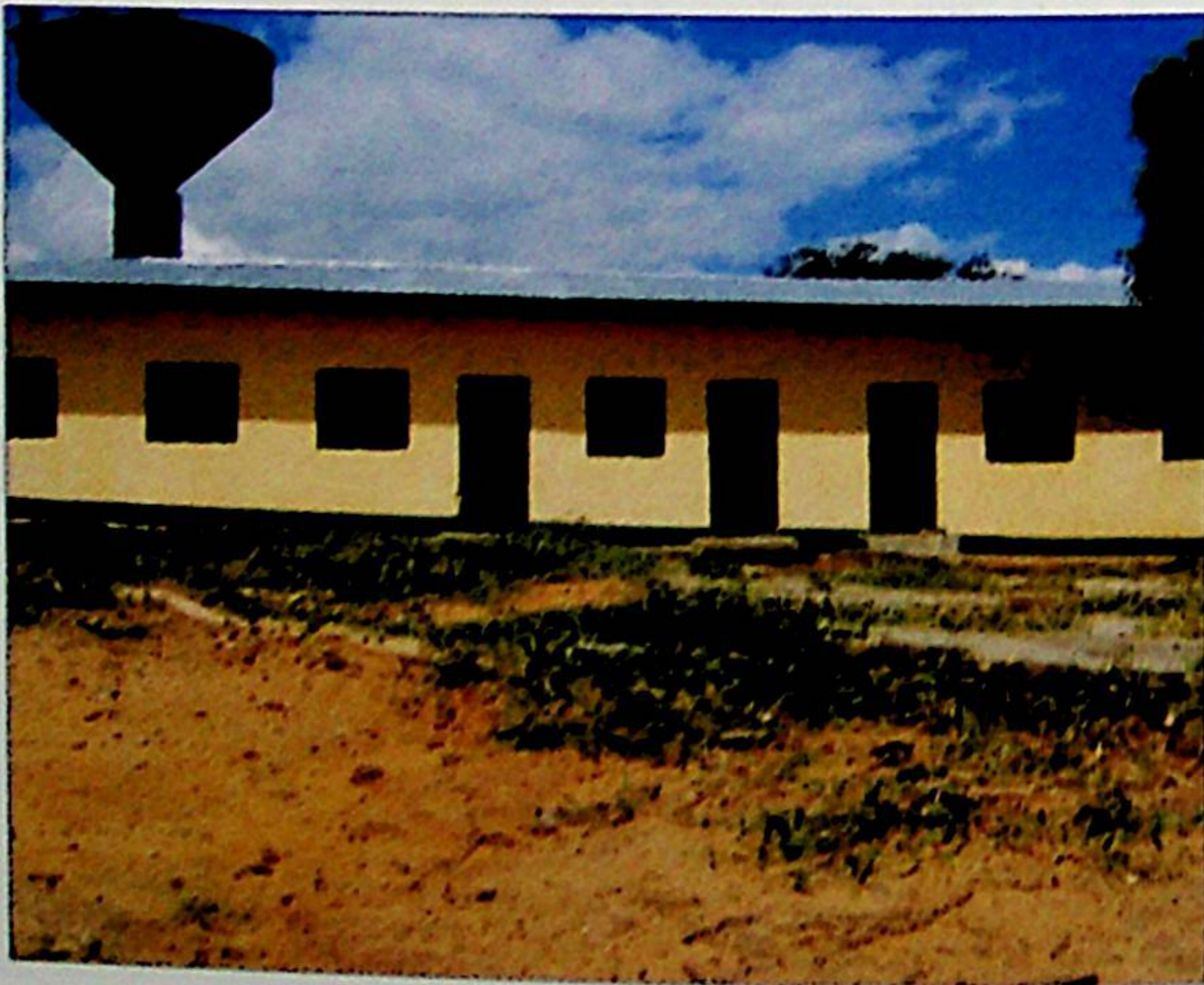
Renovated 1 Block of 2 Classrooms, office; and 7 stores at Enagi Central Primary School
