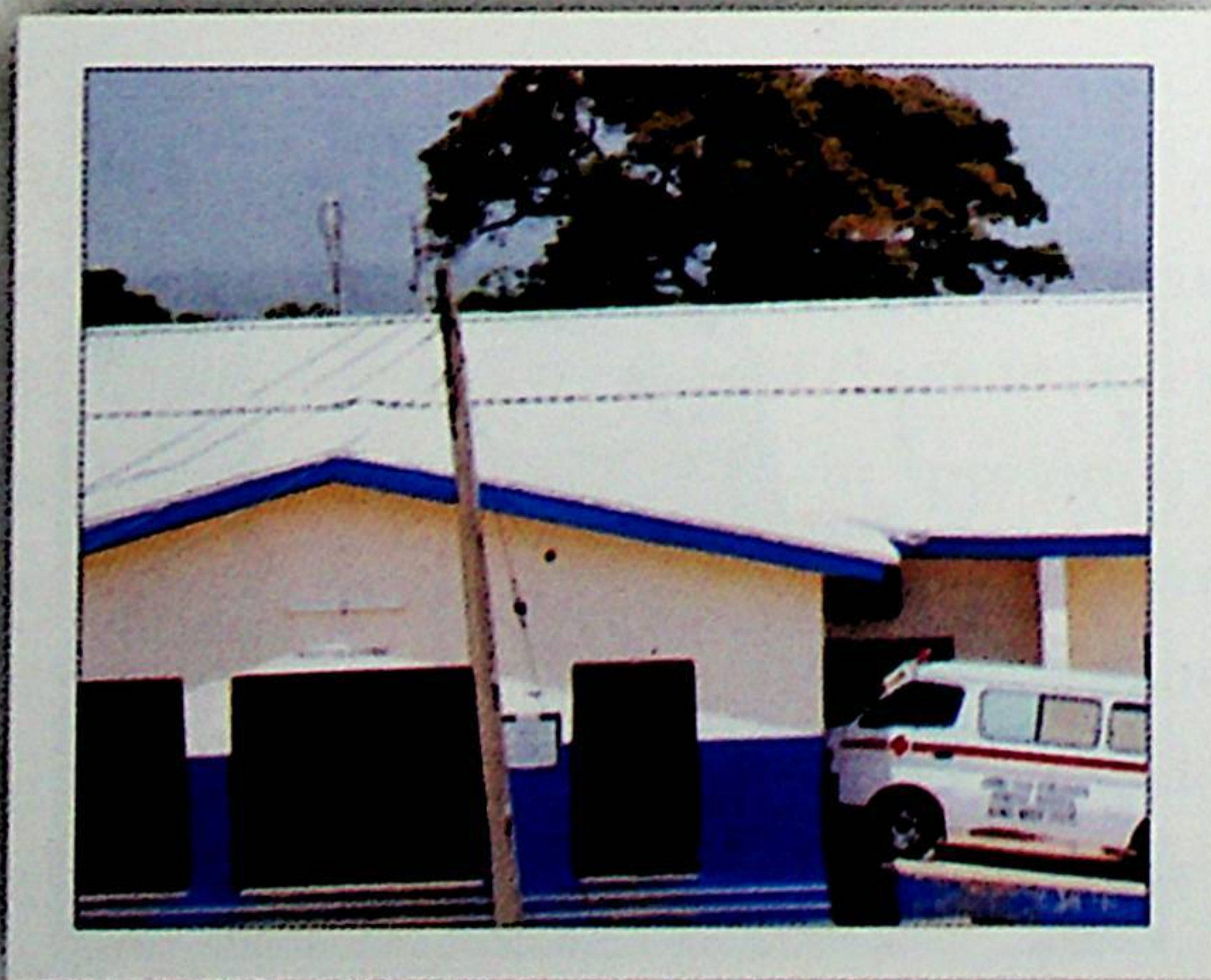
Rehabilitated rural health centre
