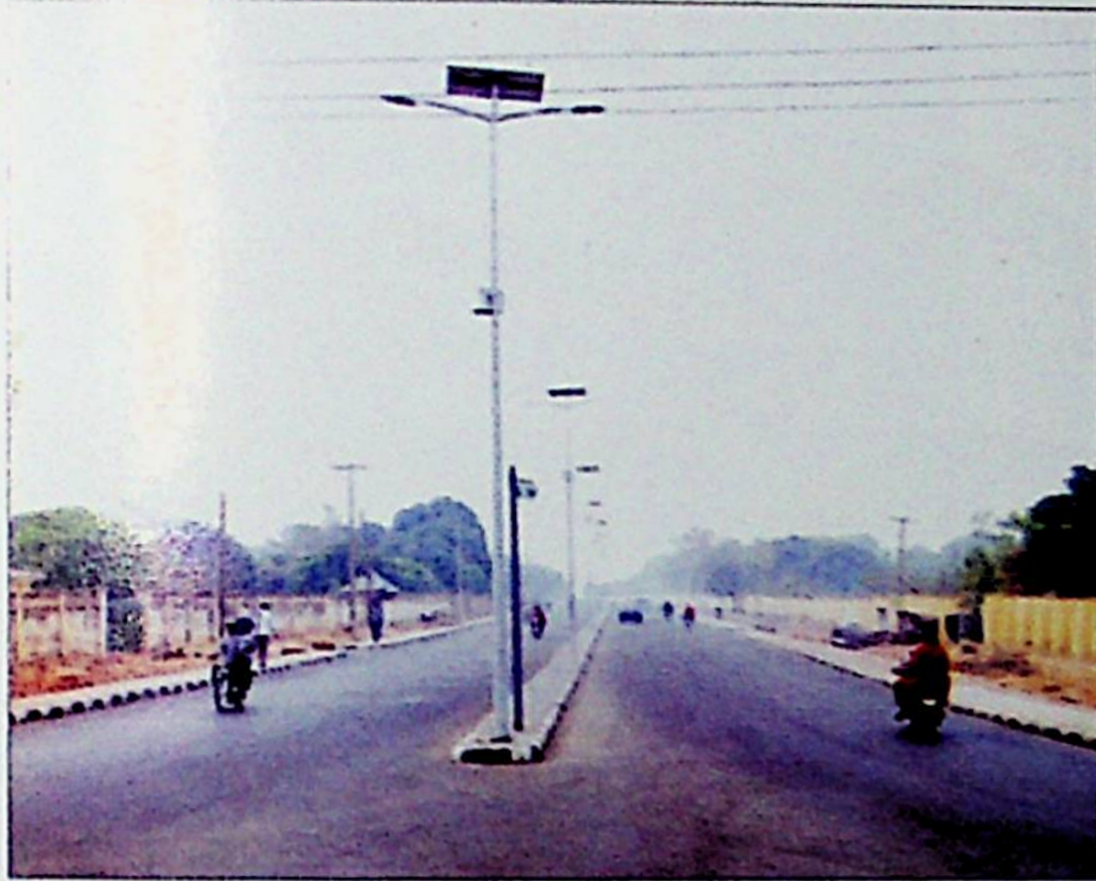
Road construction in Minna town
