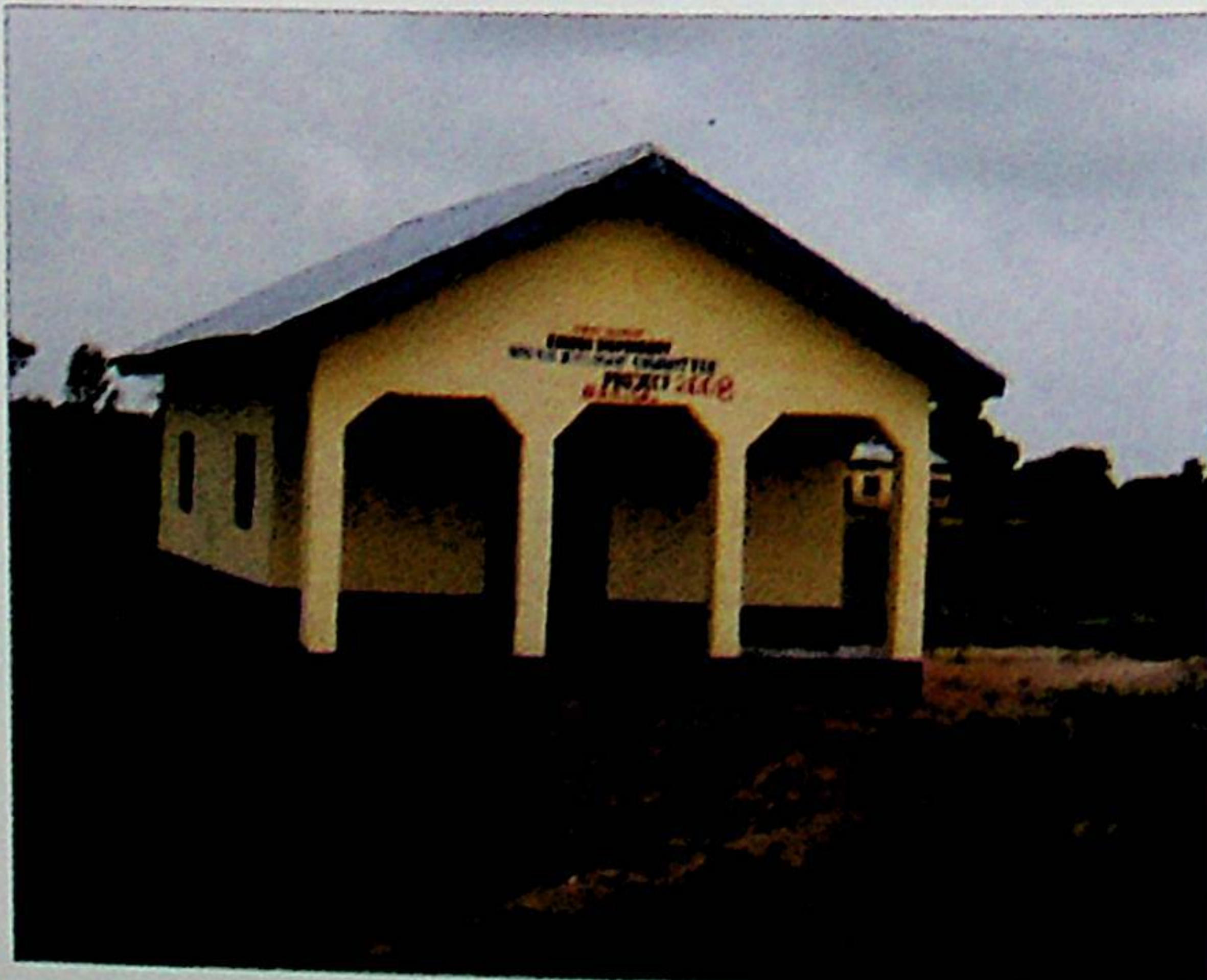
Construction of Kahigo Dispensary in Inkwai Ward
