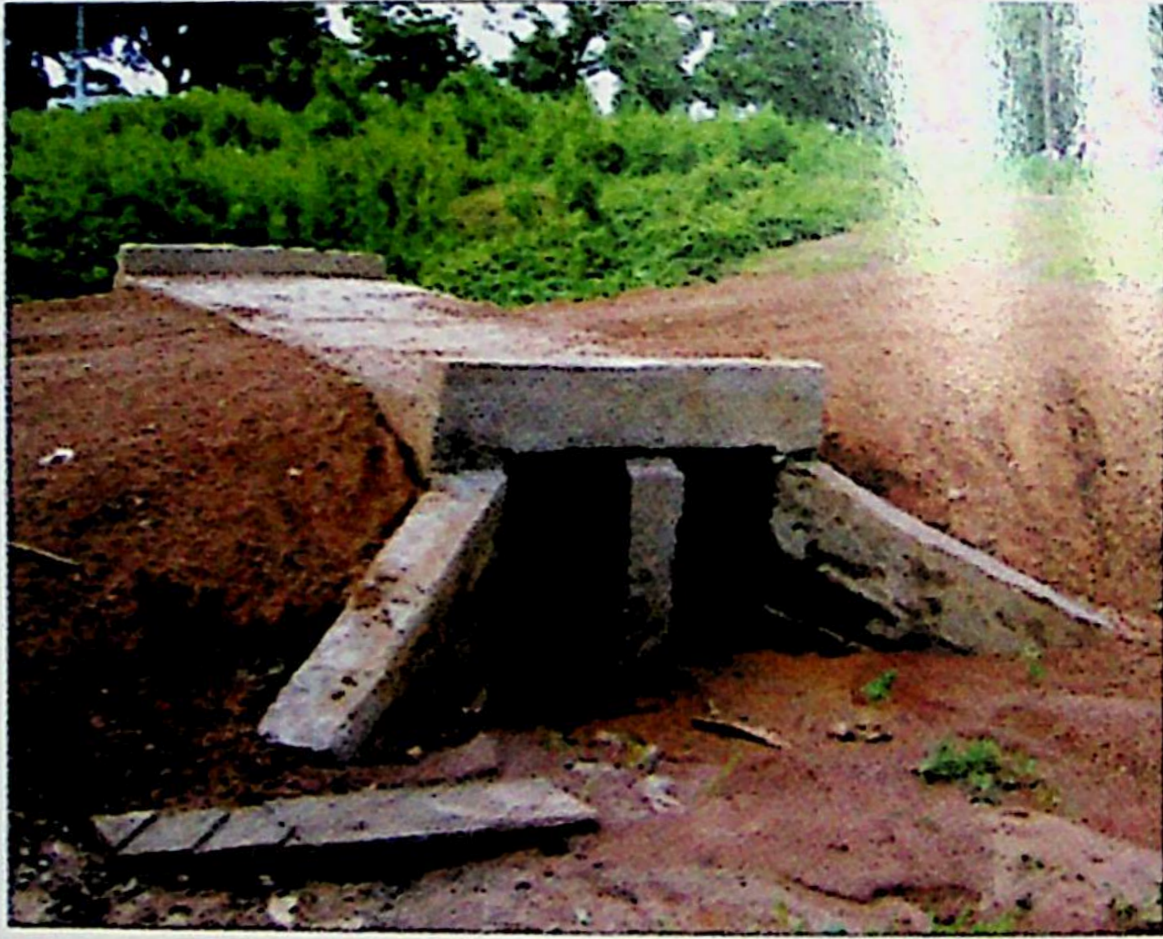
Constructed Culvert at Kata-Eregi Village
