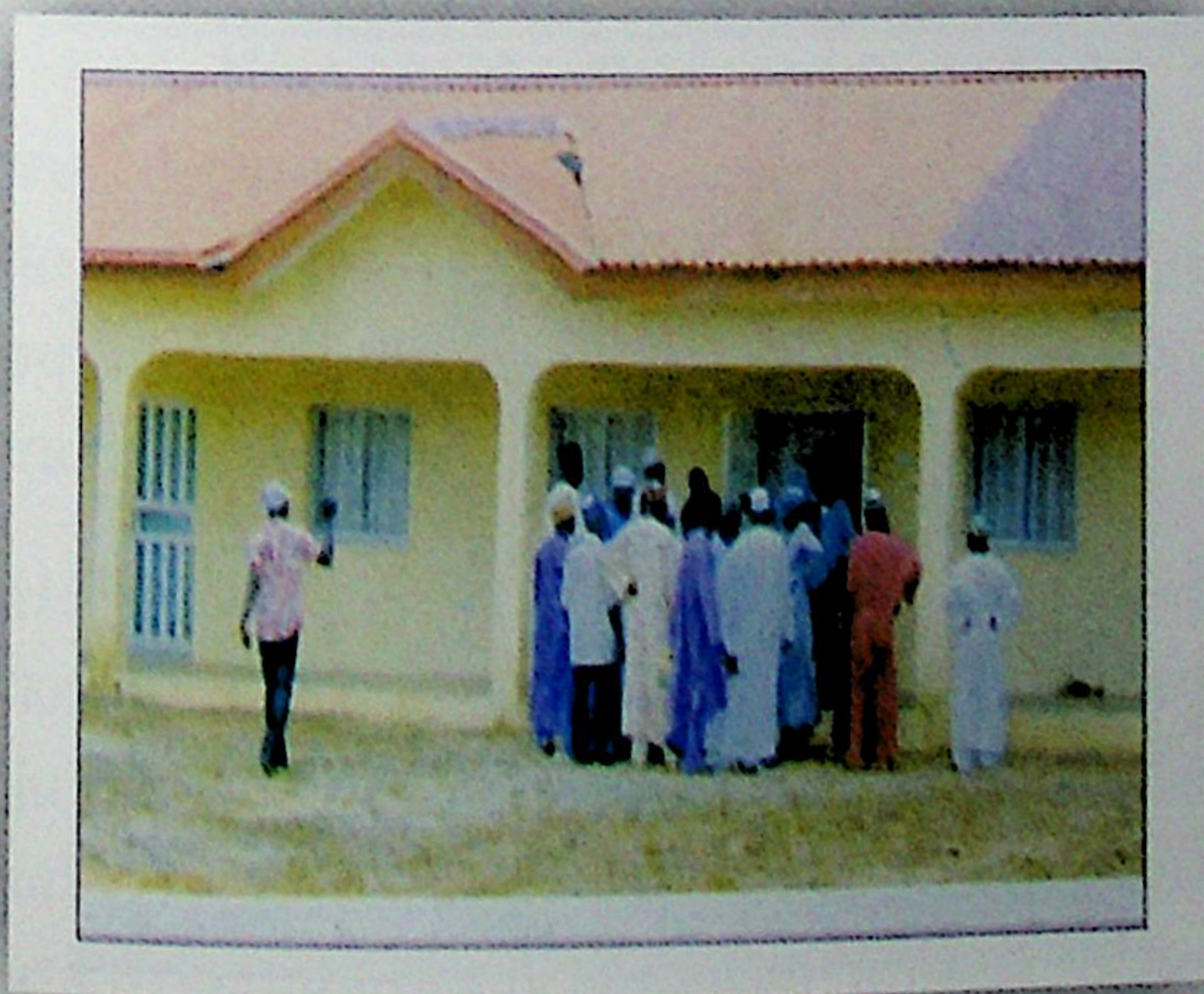
Completed Teachers' Resource Centre in Kontagora
