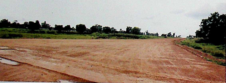
Funtua : Katsina road bye pass (on-going project)
