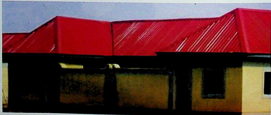
Cross section of the 252 Housing Units for Junior and middle cadre workers at Makera Village, Daura Road, Katsina State
