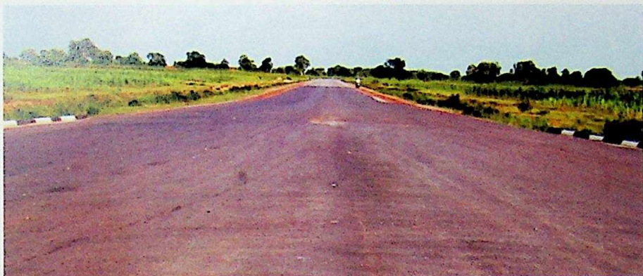
43km Karingafa-Tsiga-Yarkasuwa road
