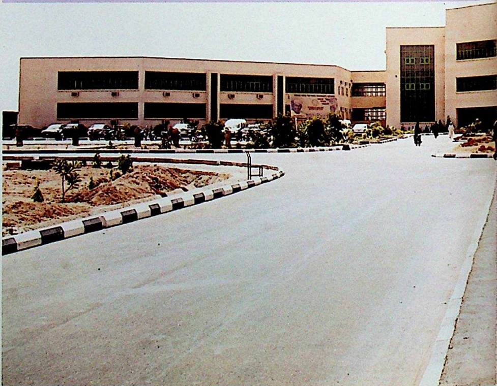
The senate building of the Umaru Musa Yar A'dua University, Katsina, inset the University library
