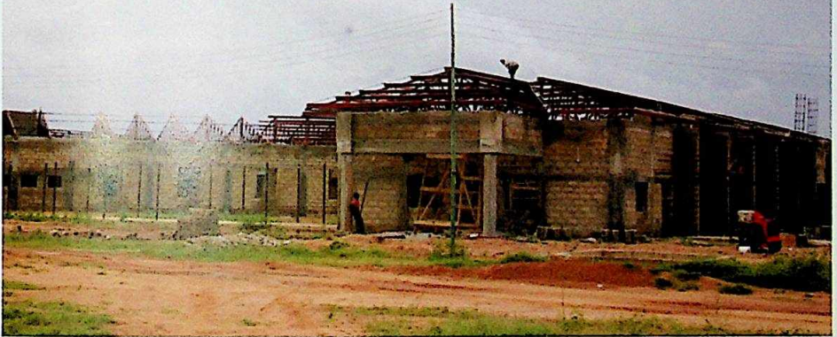
Orthopaedic Hospital, Katsina, nearing completion
