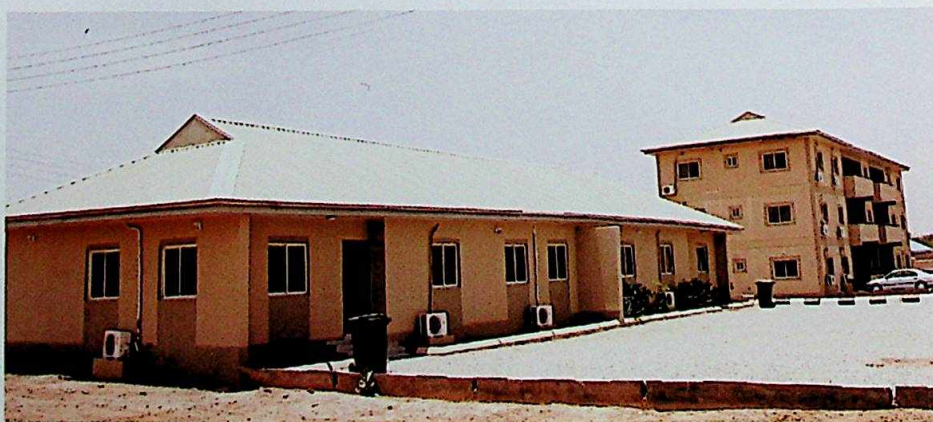
The Turai Yar'Adua Maternity and Children Hospital staff quarters
