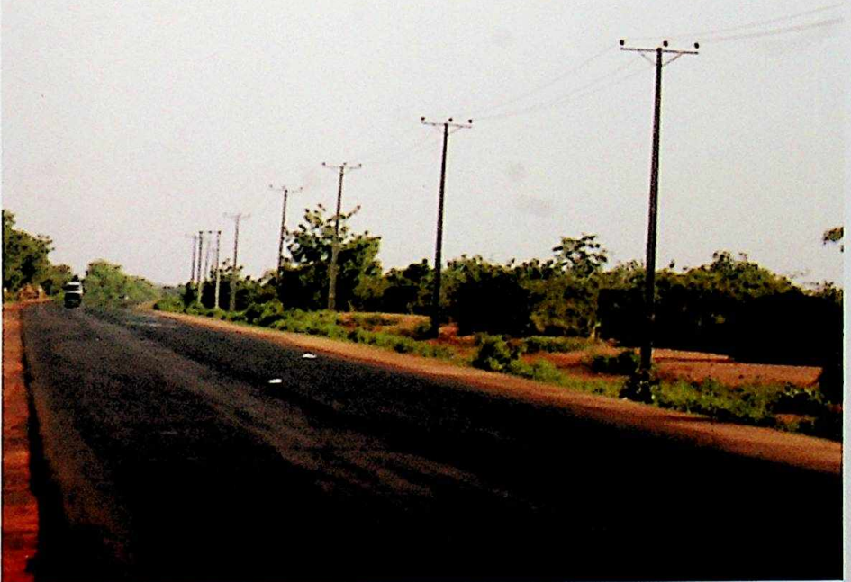
One of the extensive electrification projects, inset , some of the transformers
