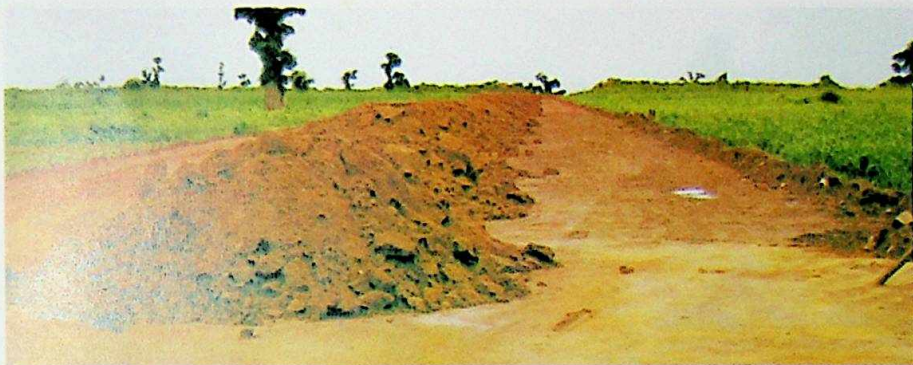
Musawa-Dangani-Mararraba Dan all road under construction
