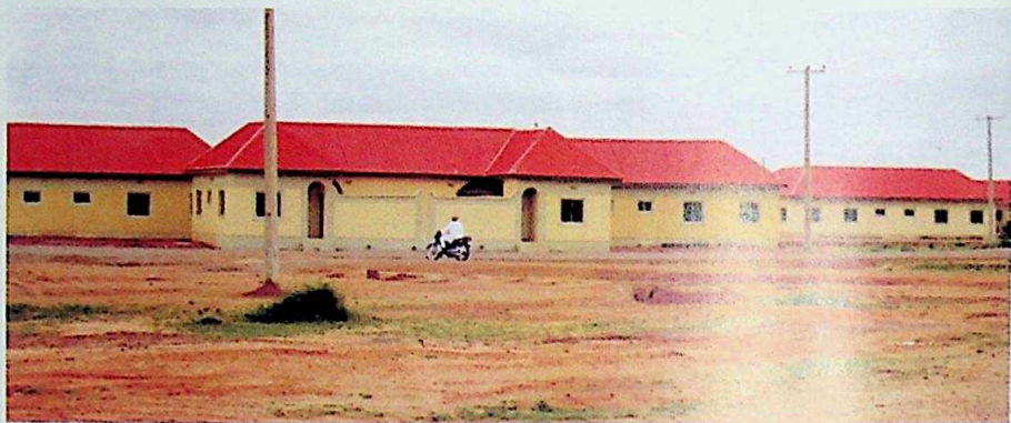
The 252 housing units at Makera, Daura Road, Katsina
