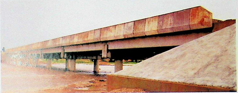
The 7 Span Karare Bridge on the Kurfi-Batsari
