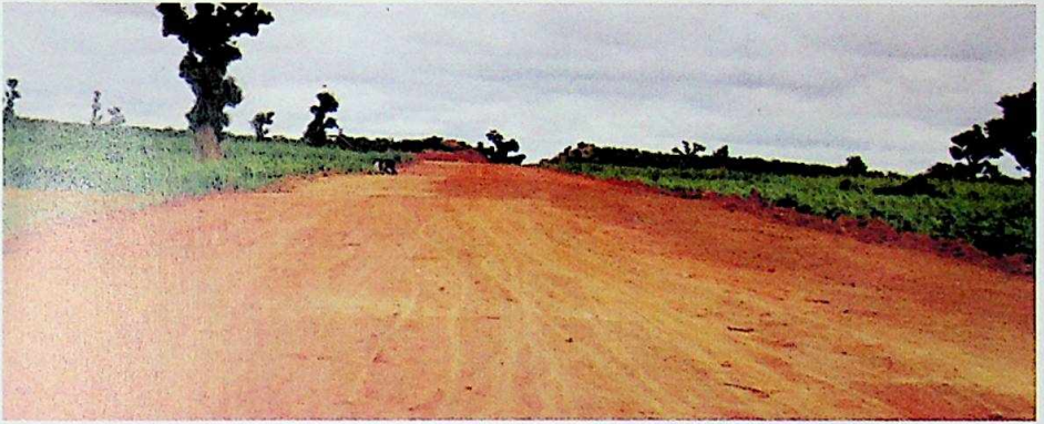
Maiadua-Gwajo Gwajo-Yaryandi-Tsabu road, under construction
