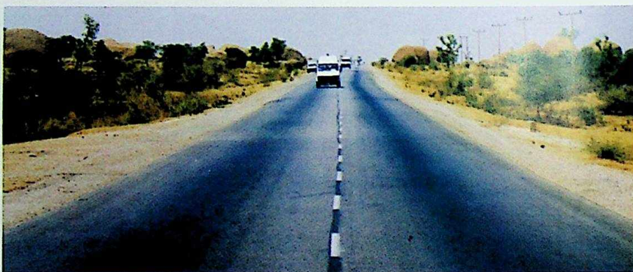
Yankara, Faskari, Maigora-Mando Junction. 45km road asphalted
