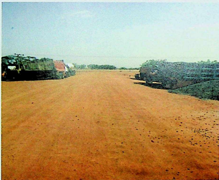
CONSTRUCTION OF KWANAR IDANDUNA – KADOWAWA - 22.4KM
