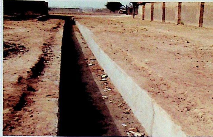
CONSTRUCTION OF DRAINAGES AND CULVERTS AT SABON GARI QUARTERS, BIRNIN KUDU TOWN, BIRNIN KUDU LOCAL GOVERNMENT AREA
