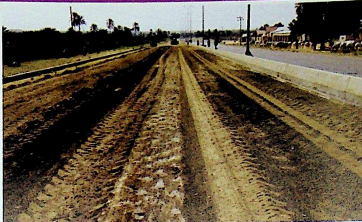
CONSTRUCTION RHS LINE DRAIN AND CARRIAGEWAY SCARIFICATION
