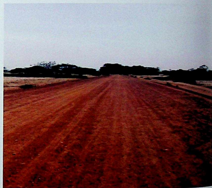
CONSTRUCTION OF TSAMIYA KWANCE – JAMUS – RATAYE - LAMINTANI - 15,1KM
