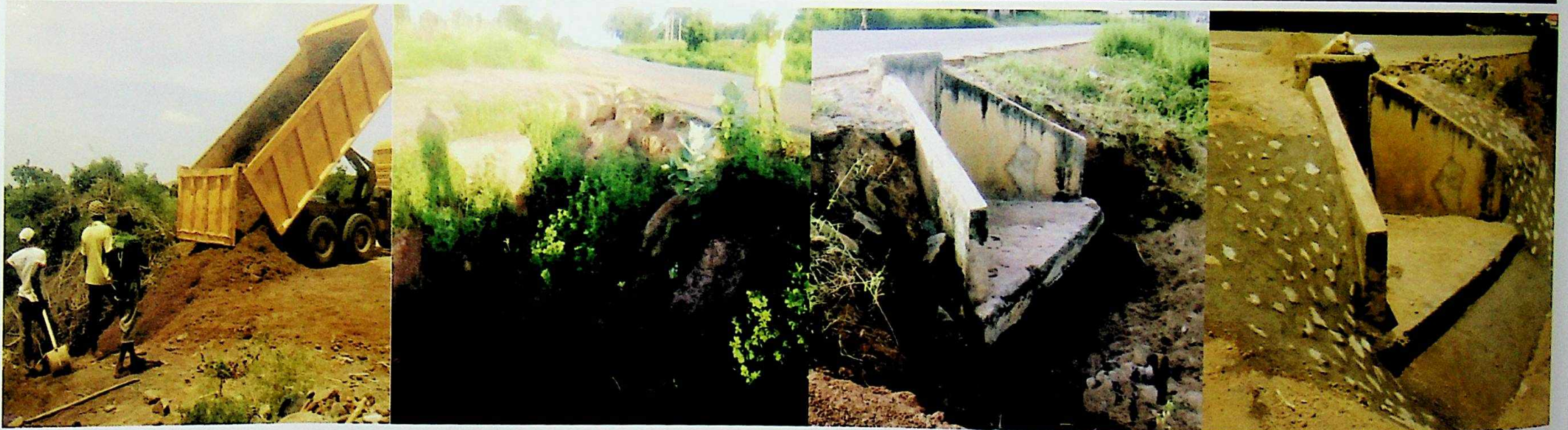
BEFORE AND AFTER THE INTERVENTION WORK
