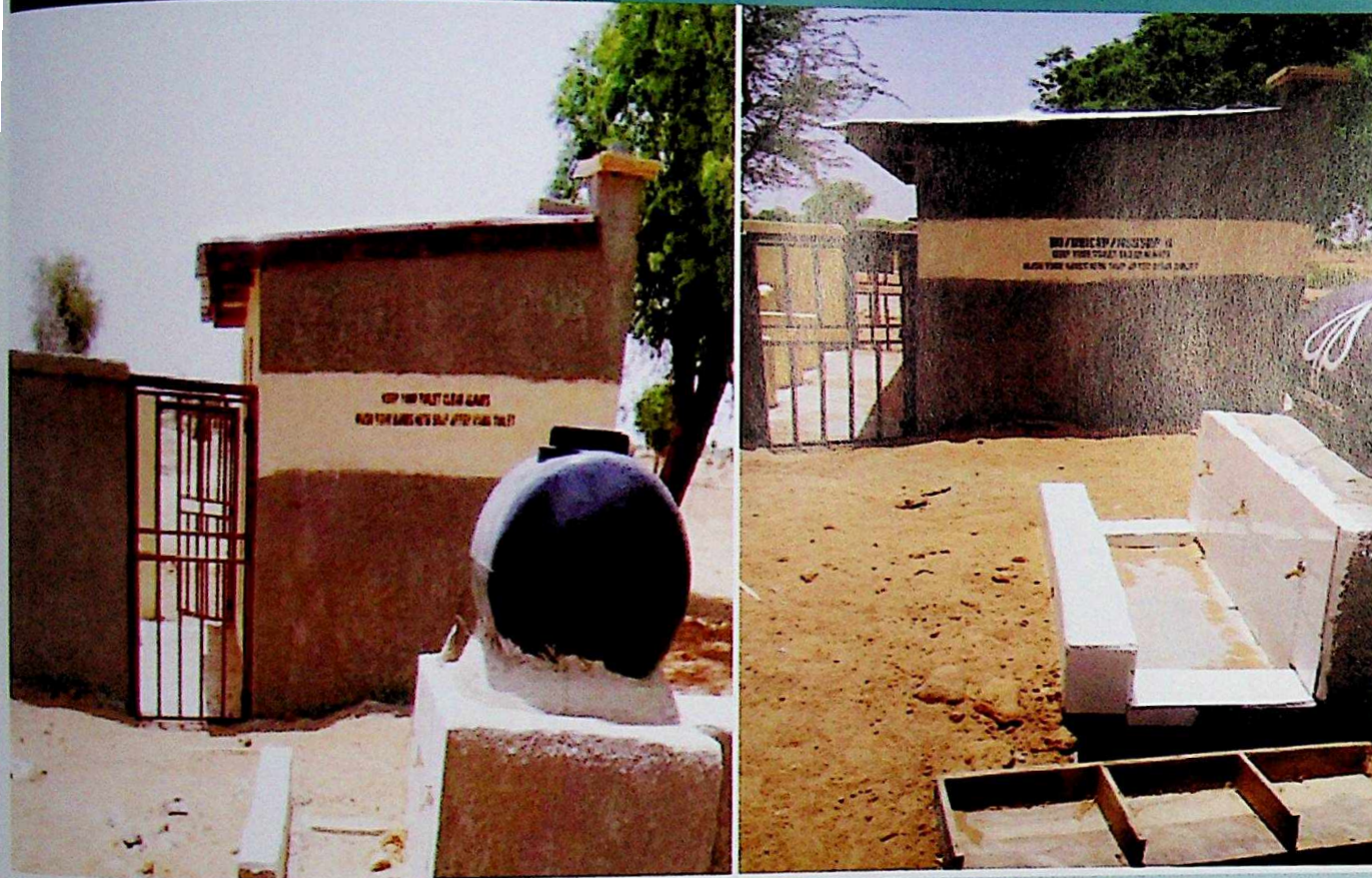
Newly constructed VIP Latrine at Babuwa Primary School M/Madori
