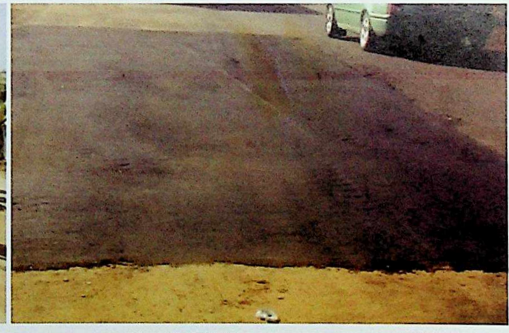
COMPLETED SECTION OF GWARAM- BASIRKA ROAD AFTER THE INTERVENTION WORK
