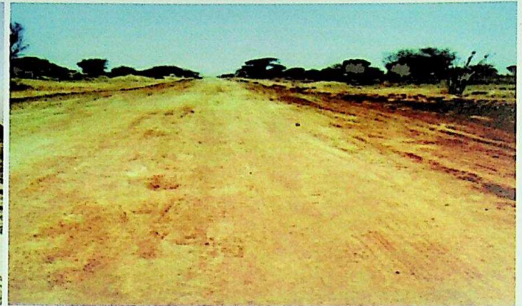
SPREADING AND SHAPING
