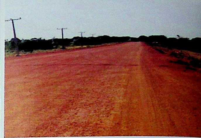
BASE COURSE APPLICATION
