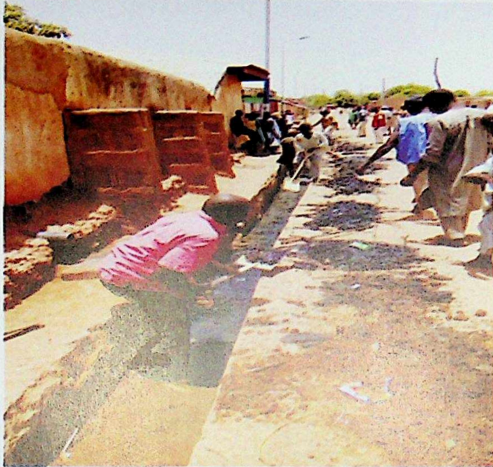
A self help group desilting drainages
