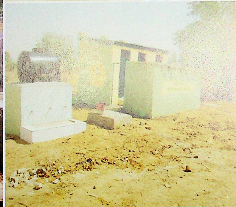
One of the 300 constructed VIP Latrine in Schools across the State
