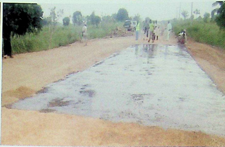
PRIMING AT GADAMA CULVERT
