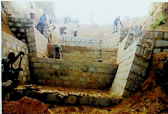
CONSTRUCTION OF RETAINING WALL
