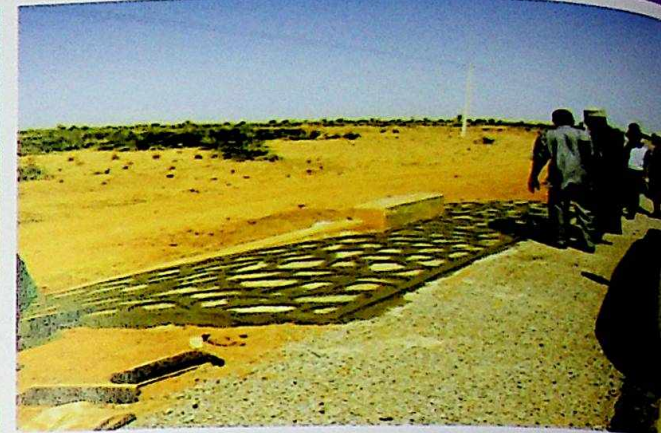
STONE PITCHING (PROTECTION OF EMBANKMENT)
