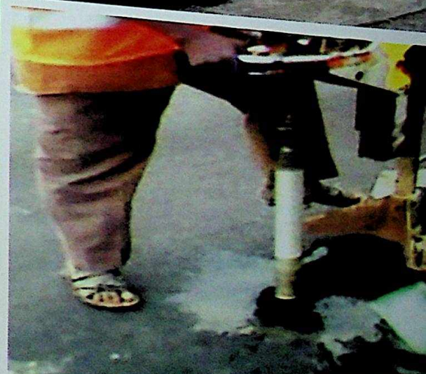
PRIMING IN PROGRESS AND CORING TEST
