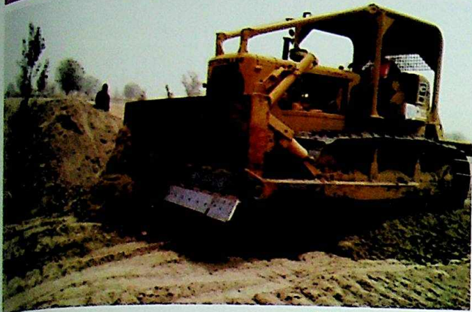
DUMPING AND SPREADING OF FILL MATERIAL
