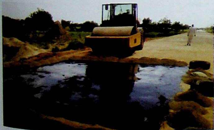
SURFACE DRESSING WORK AT GADAMA CULVERT 1 ST SECTION
