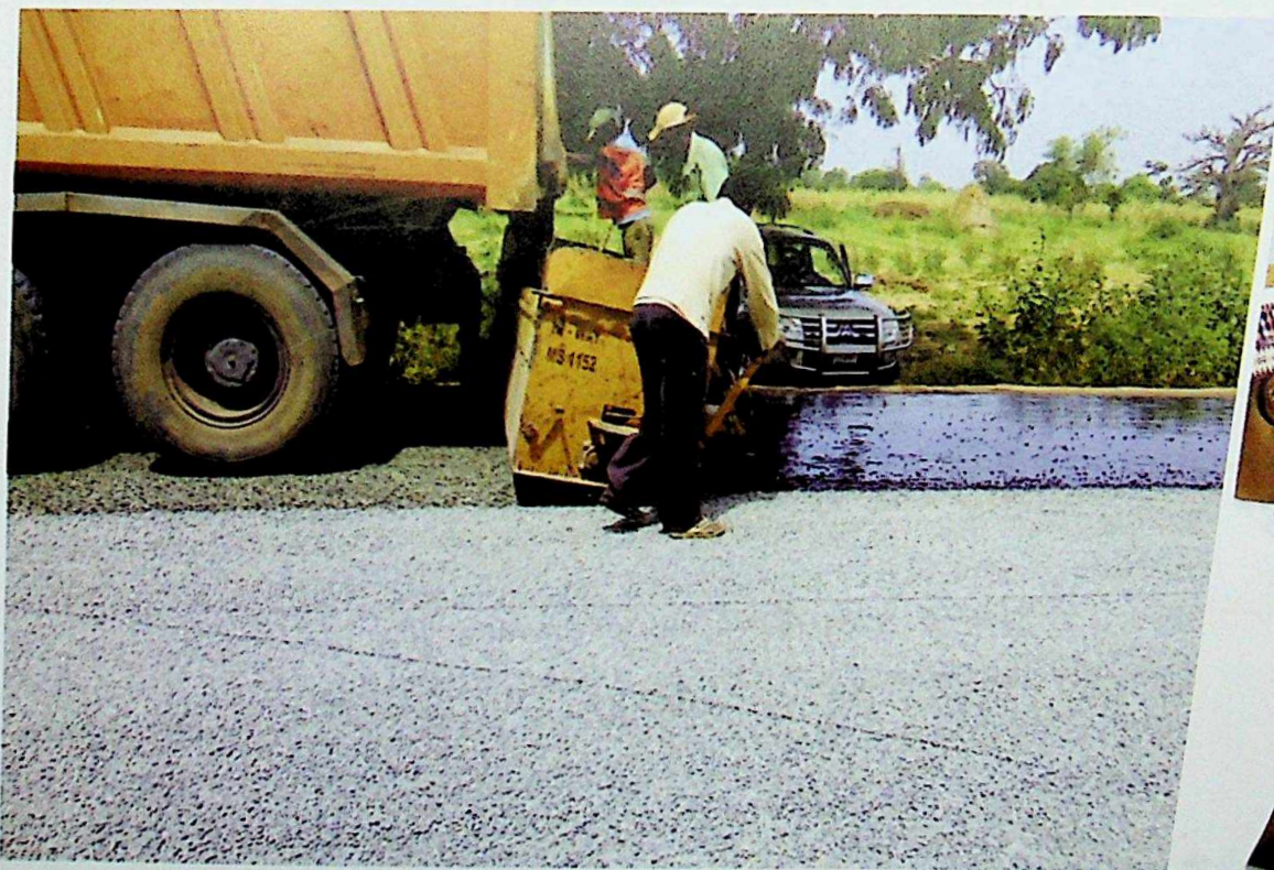
SURFACE DRESSING IN PROGRESS
