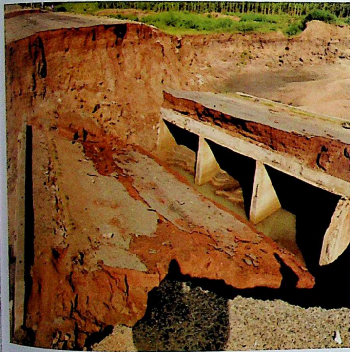
DAMAGED 6 CELL BOX CULVERT
