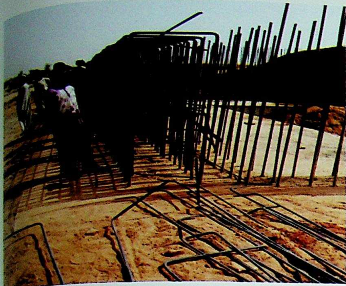
ARRANGEMENT OF REINFORCEMENT FOR ABUTMENT
