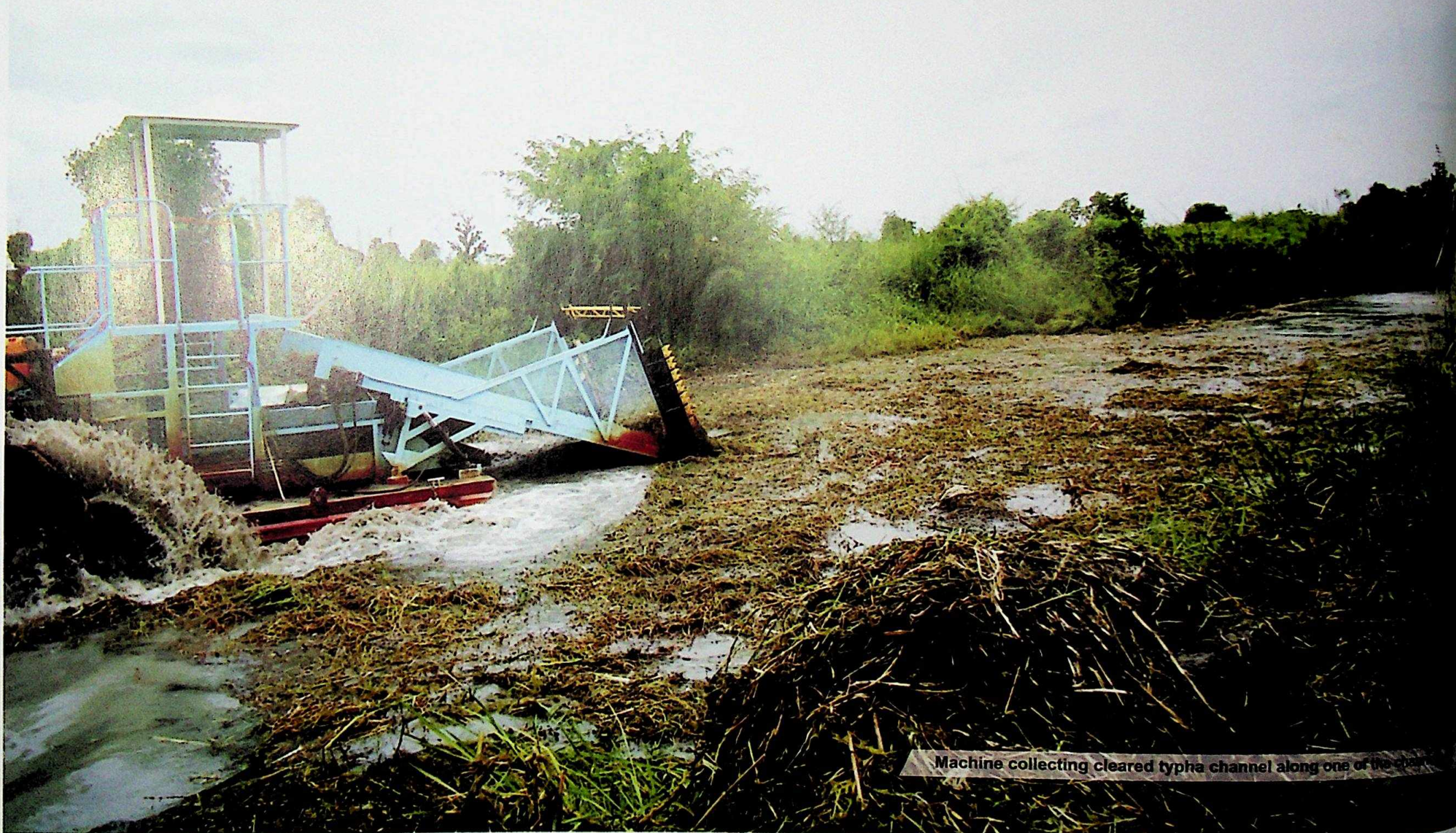
Clearing of the Guri Bridge Channel
