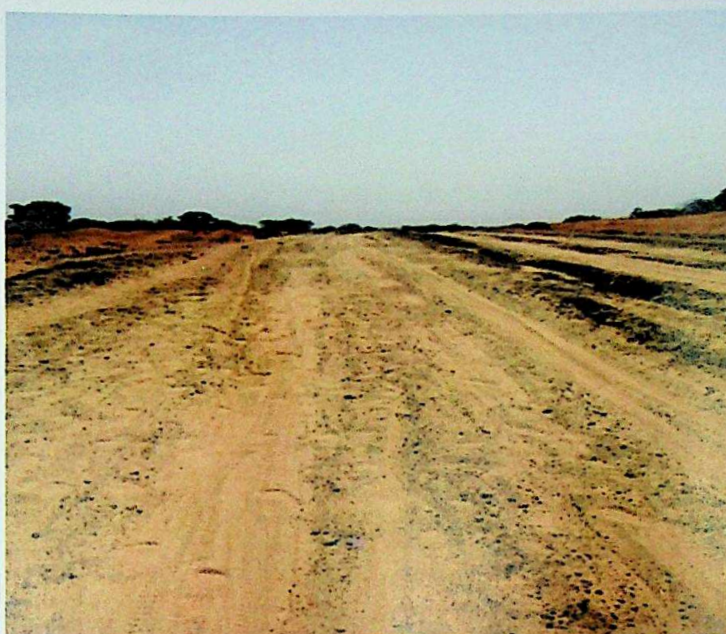
CONSTRUCTION OF SHAFAR – GIDAN SANI – DAGUZAU ROAD - 17.4KM
