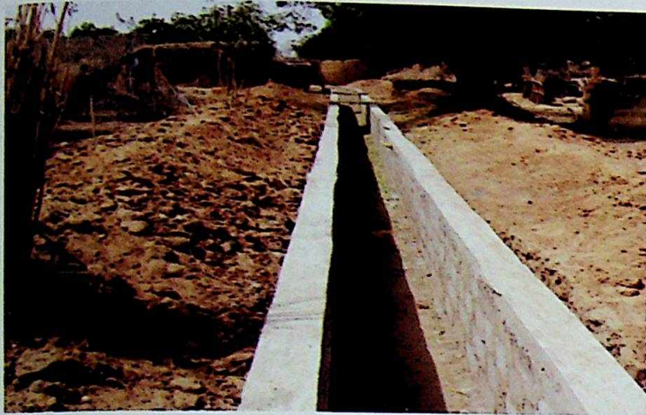
CONSTRUCTION OF DRAINAGES AND CULVERTS AT CHAMO TOWN, DUTSE LOCAL GOVERNMENT AREA
