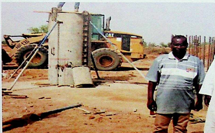
CASTING OF PILE STRUCTURE
