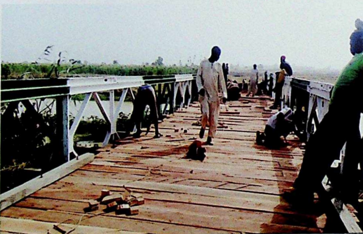
INSTALLATION OF NEW TIMBER DECKING
