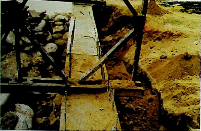
CONSTRUCTION OF ABUTMENT
