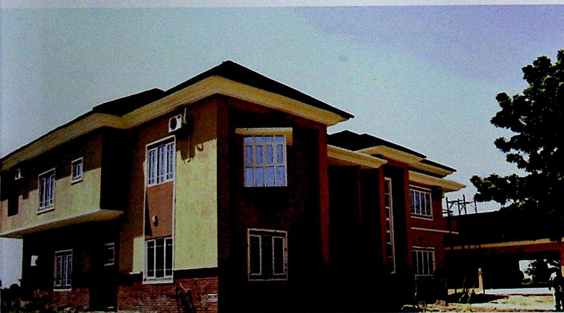
Side view of the completed VC lodge
