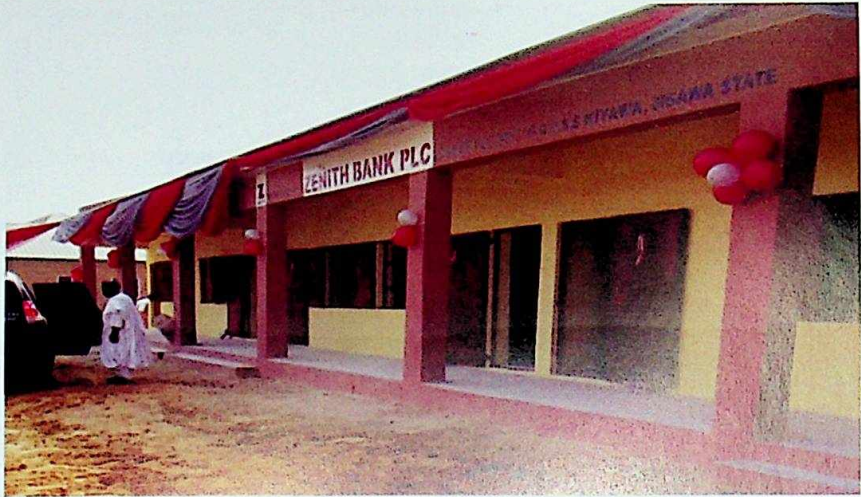
CSR Projects -Commissioning of Zenith Bank project at Kiyawa
