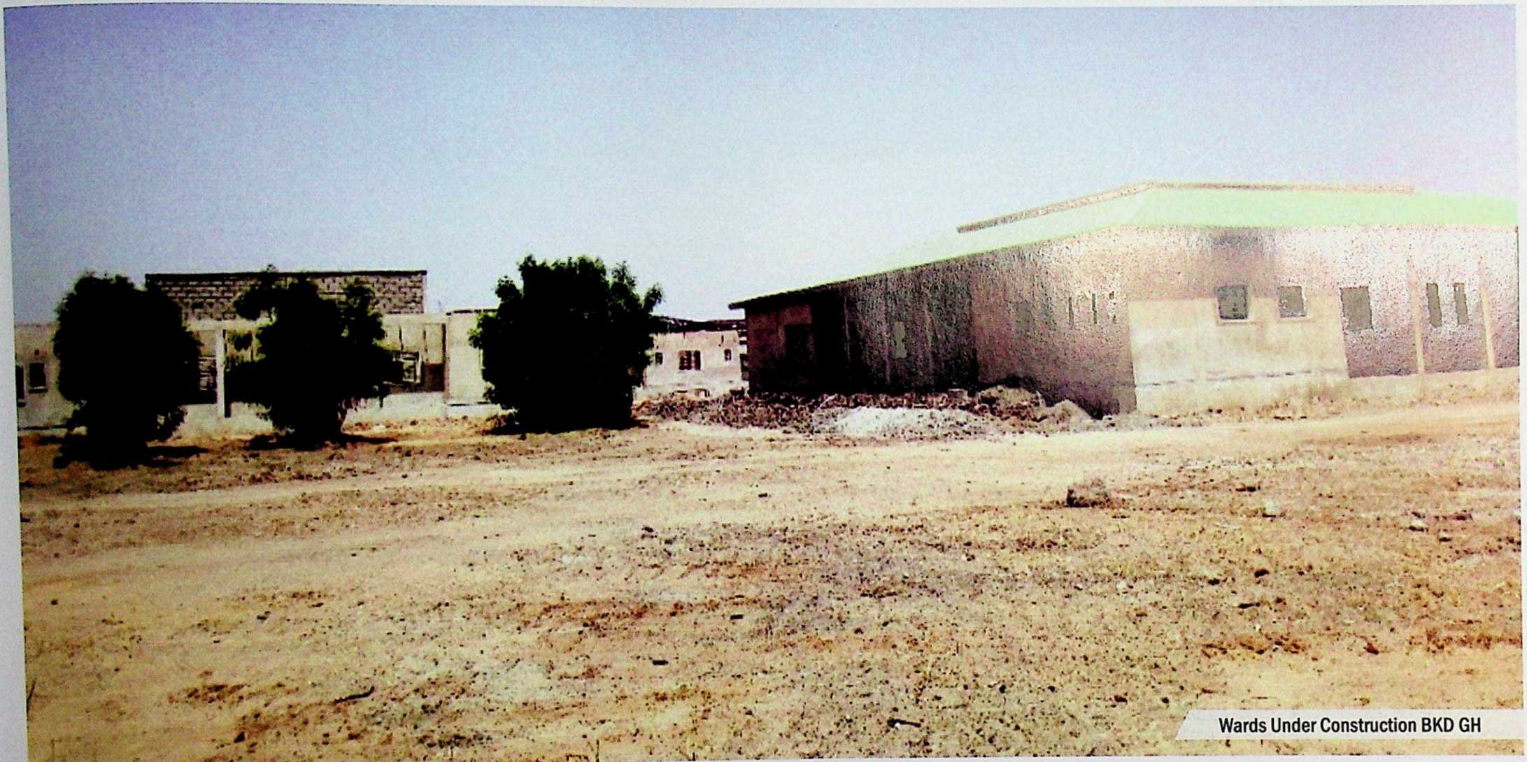
New Birnin Kudu General Hospital-Gate and Gate House
