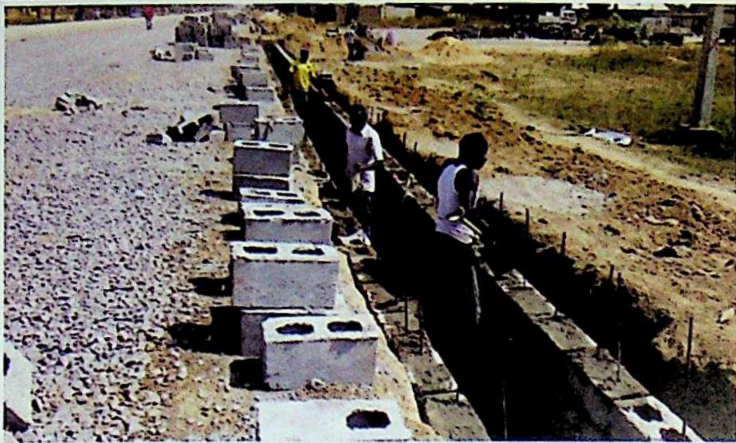
CONSTRUCTION RHS LINE DRAIN AND CARRIAGEWAY SCARIFICATION
