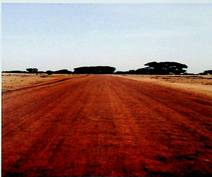
CONSTRUCTION OF MALLAM MADORI- DAKIDO - 5.4KM
