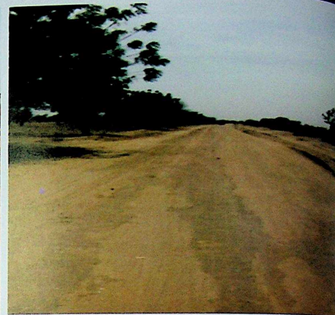
CONSTRUCTION OF GUMEL – GARIN GAMBO ROAD - 7KM
