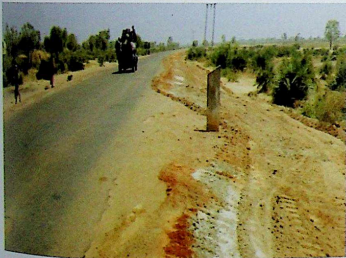
SCARIFICATION OF SHOULDER AND DUMPING OF BASE MATERIAL
