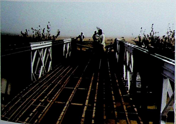
REPAINTING AND REPAIR OF STRINGERS
