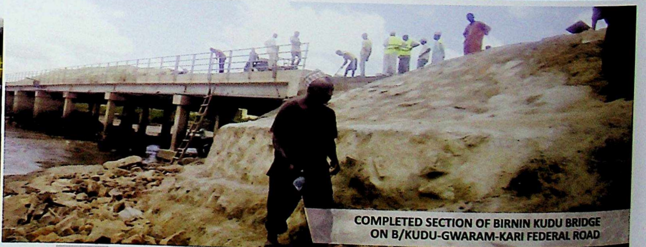
STONE PITCHING WORK AT BIRNIN KUDU BRIDGE
