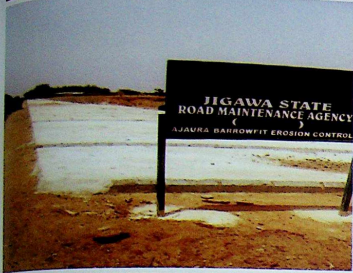
COMPLETED EROSION CONTROL SITE
