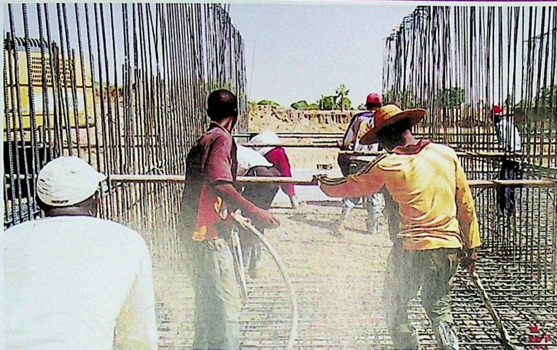
RECONSTRUCTION WORK ON PROGRESS
