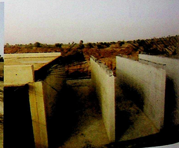
3 CELL BOX CULVERT UNDER CONSTRUCTION
