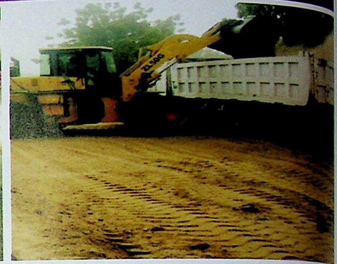
REMOVAL OF UNSUITABLE
