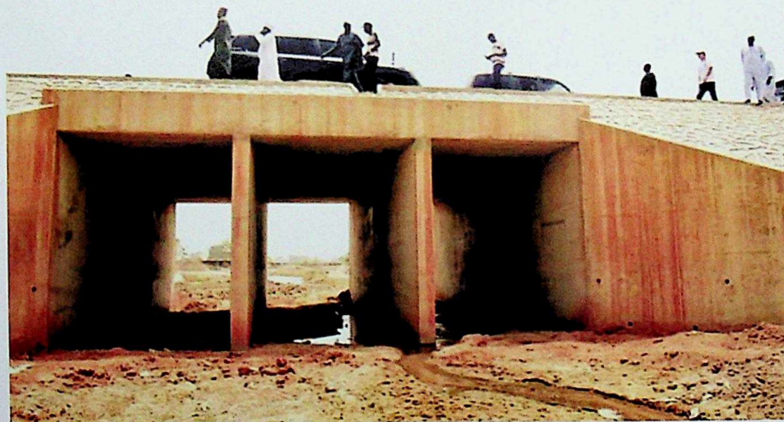
COMPLETED CULVERT
