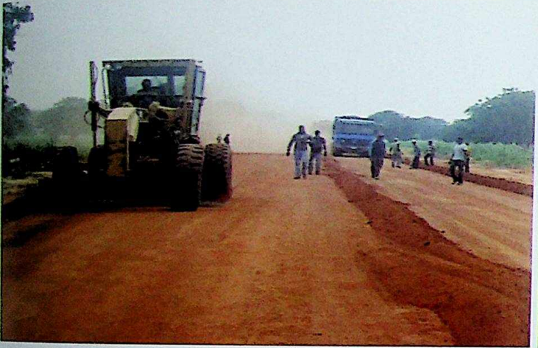
CLEARANCE AND GRADING OF SUBBASE
