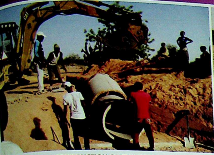
CONSTRUCTION OF CULVERT
