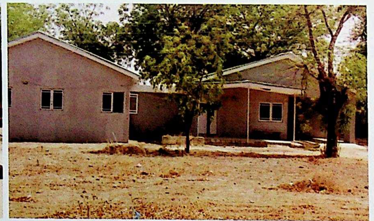
Babura GH Renovated Staff Quarters
