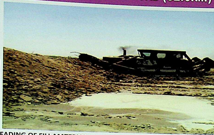
SPREADING AND SHAPING
