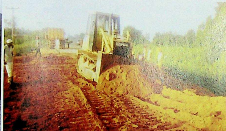
EARTH WORKS IN PROGRESS AT GADAMA CULVERT
