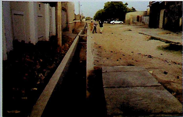
CONSTRUCTION OF DRAINAGES AND CULVERTS AT FANISAU QUARTERS HADEJIA TOWN, HADEJIA LOCAL GOVERNMENT AREA
