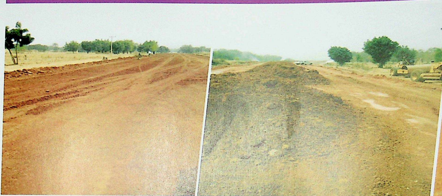
SPREADING OF LATERITE SUBBASE MATERIAL AND DUMPING OF BASE MATERIAL
