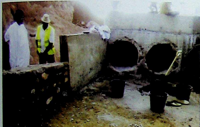
DIRECTOR ENGINEERING JIRMA INSPECTING PROTECTION WORK GADAMA CULVERT
