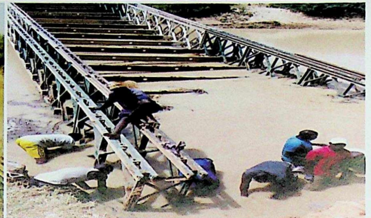
JACKING IN PROGRESS
