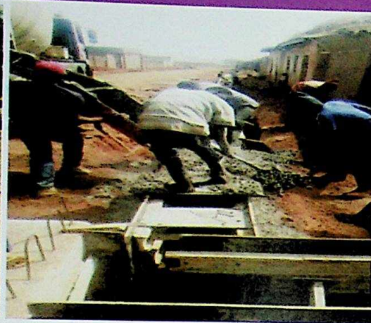
CONCRETE DRAINAGE WORKS
