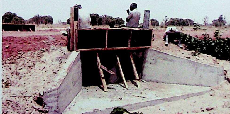
ON GOING CONSTRUCTION OF CULVERT AND CARRIAGEWAY
