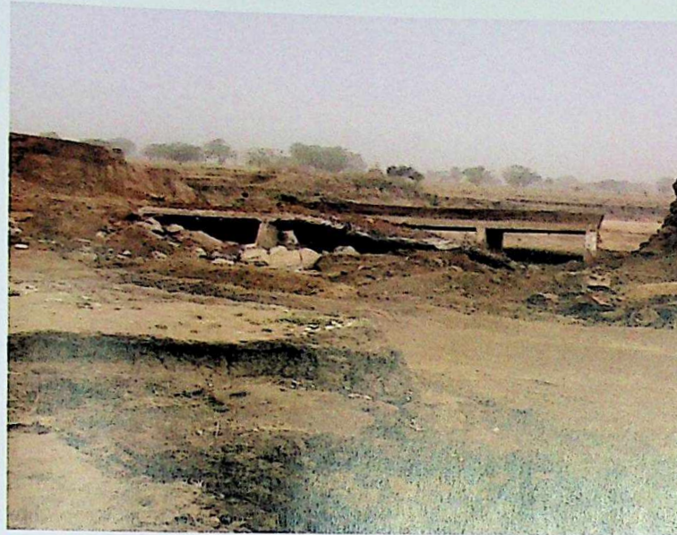
DEMOLITION OF THE FAILED CULVERTS
