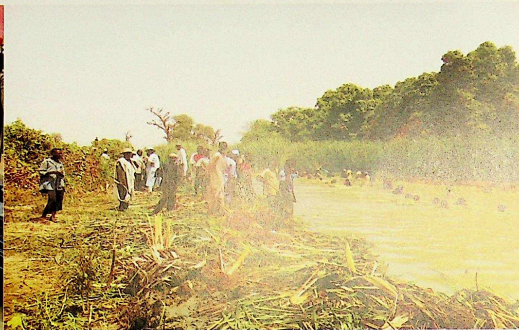
Manual Removal of Typha Grass at Burungana river channel
