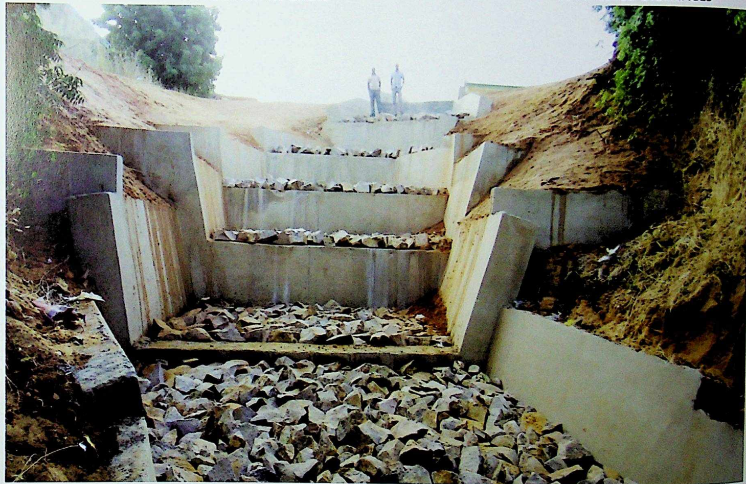
COMPLETED RETAINING WALL
