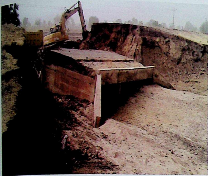
DEMOLITION OF THE FAILED CULVERTS
