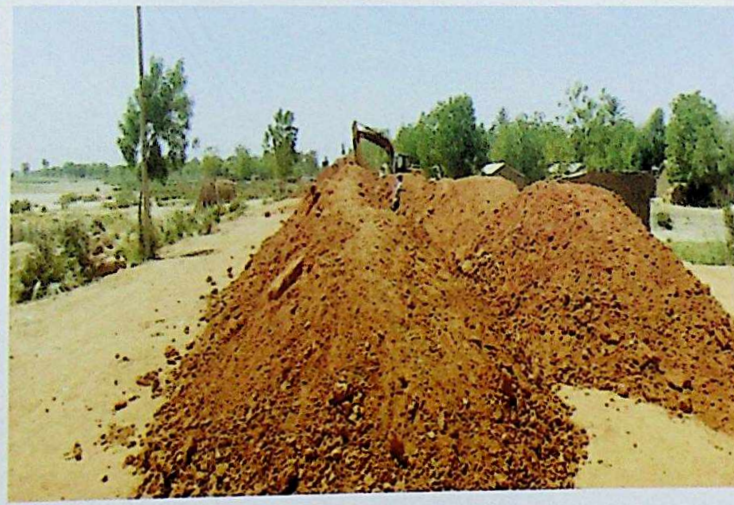
SCARIFICATION OF SHOULDER AND DUMPING OF BASE MATERIAL
