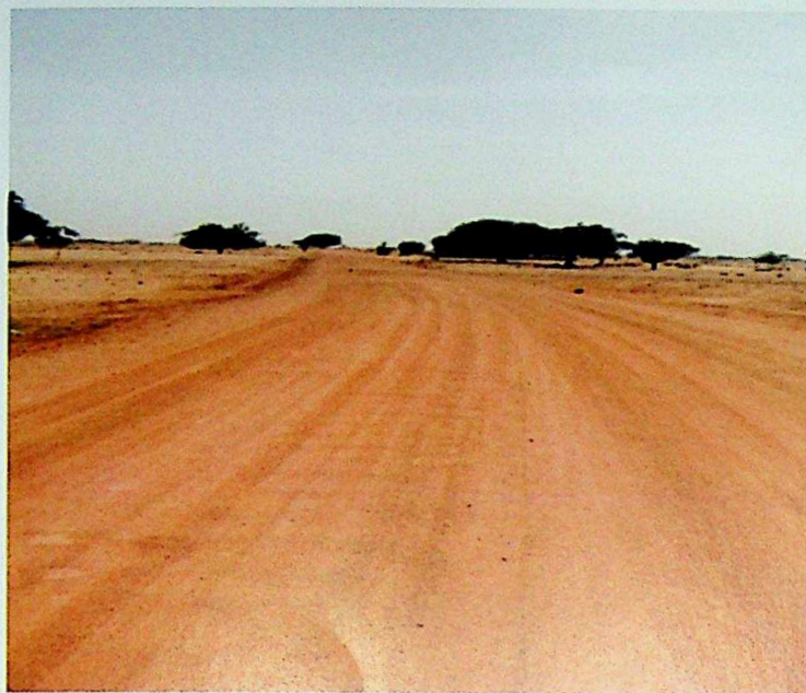
CONSTRUCTION OF LAMBAR ZAUMAR MAHAUTA – DUWIGI – GWIWA ROAD - 15KM
