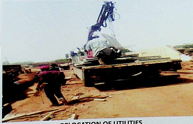
RELOCATION OF UTILITIES
