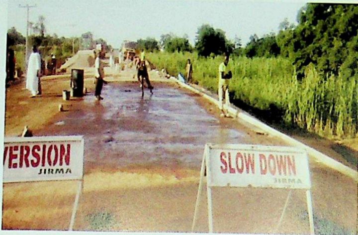
PRIMING AT GADAMA CULVERT
