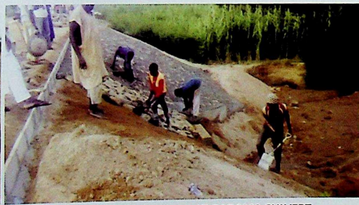
STONE PITCHING WORK AT GADAMA CULVERT
