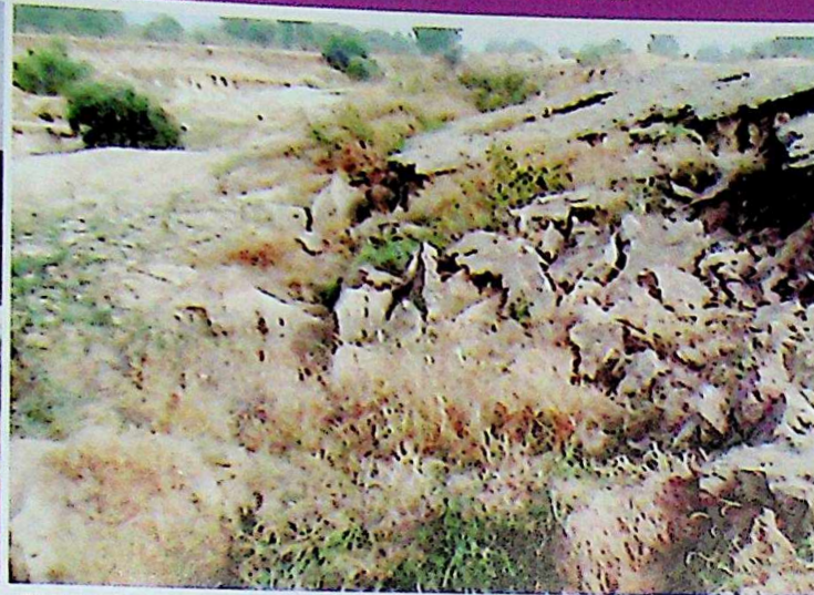
FAILED EMBANKMENT THREATENING THE PAVEMENT AT KADAITA
