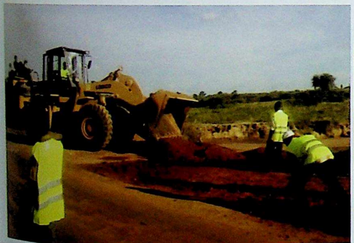
WORKS IN PROGRESS AT GWARAM – BASIRKA ROAD
