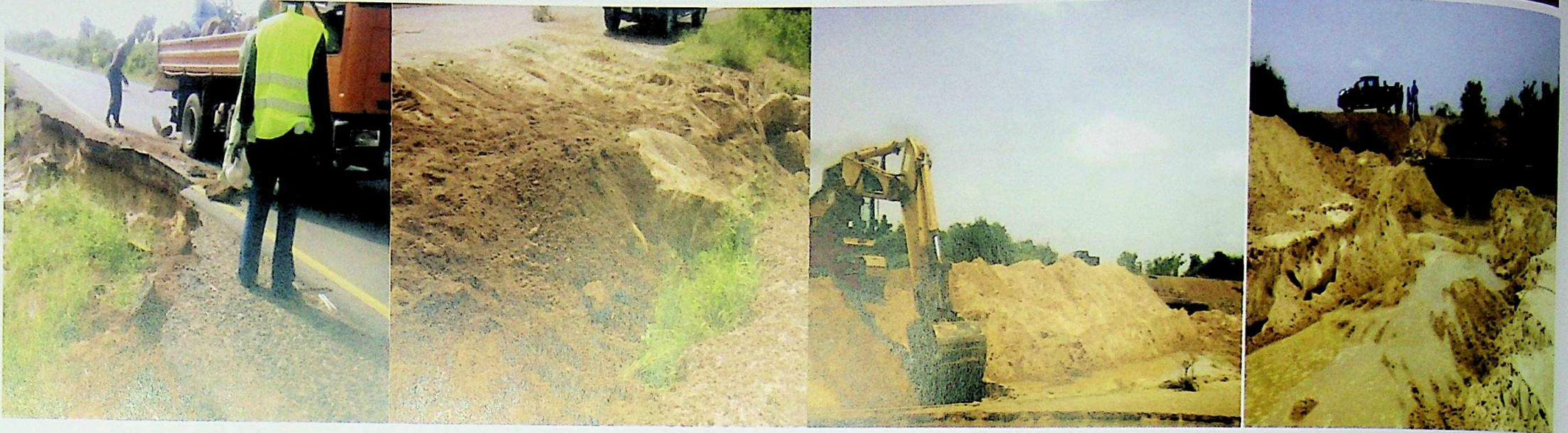
BEFORE AND AFTER THE INTERVENTION WORK
