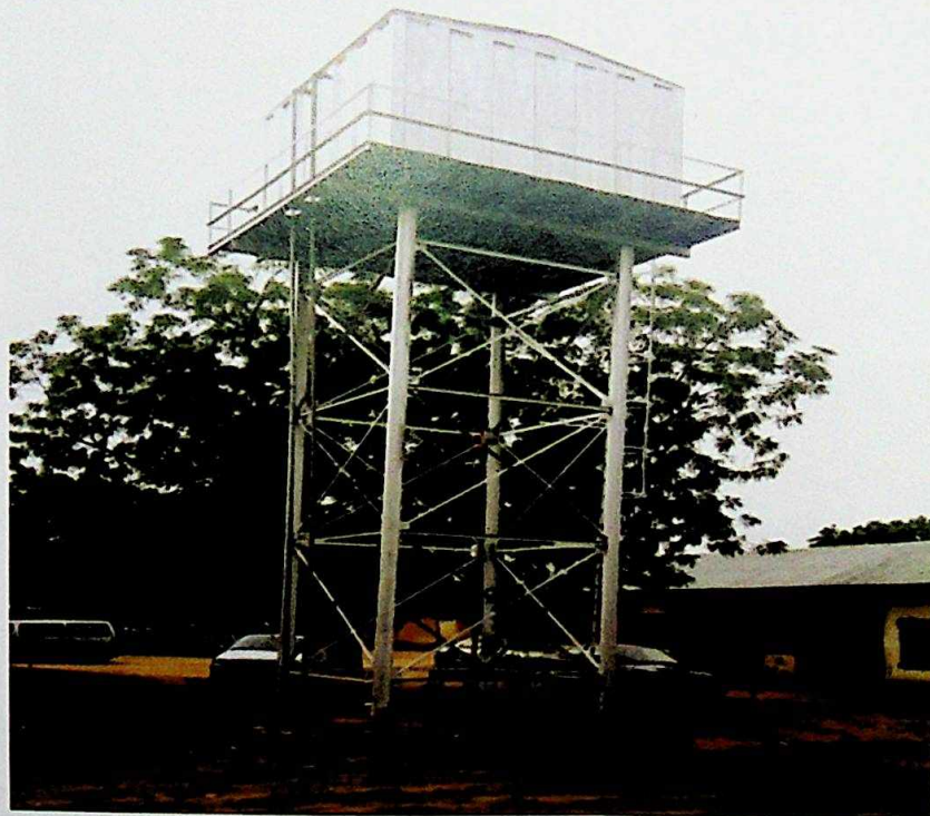
Improved Garki water scheme
