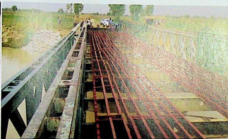
RE ASSEMBLING STRINGERS
