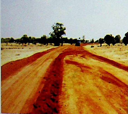
SPREADING OF SUB BASE MATERIAL
