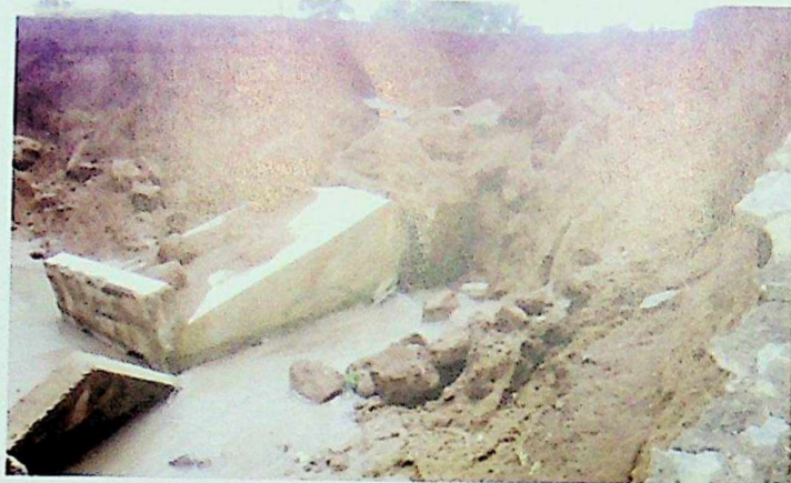
FAILED CULVERT AT GADAMA (NO.2) ON GWARAM - FAGAM ROAD
