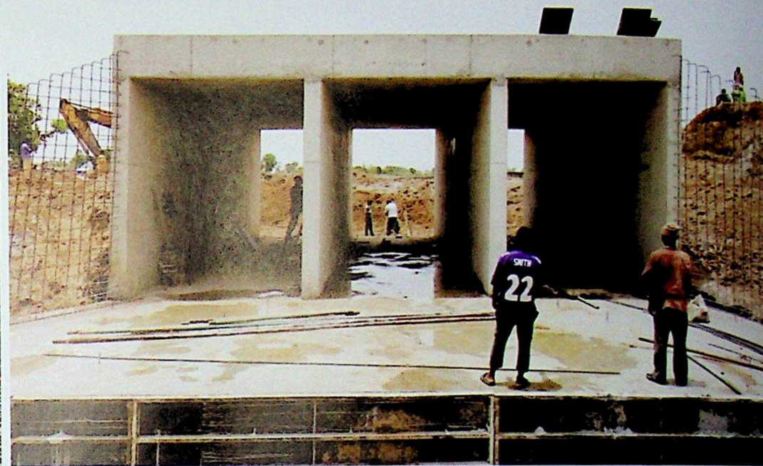
TSAMIYA - YALWANDAMAI- BIRNIN KUDU ROAD WORK IN PROGRESS
