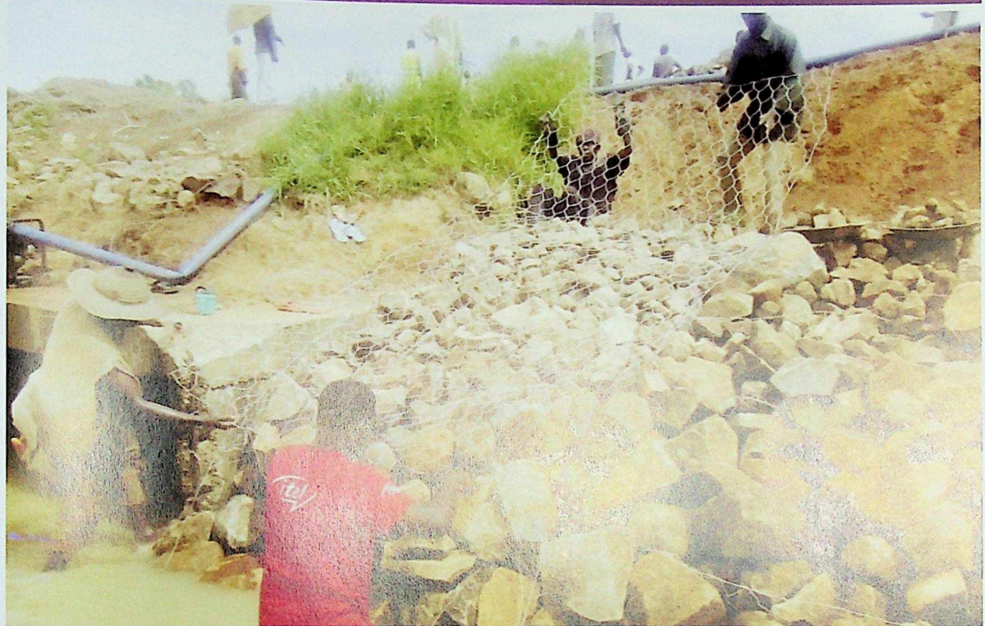
WORKS IN PROGRESS AT GWARAM – BASIRKA ROAD
