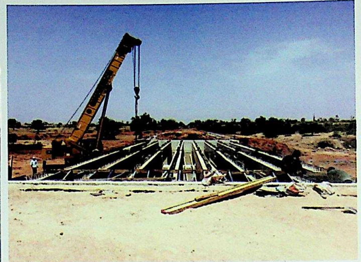
INSTALLATION OF BEAM GIRLERS
