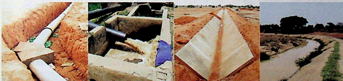
New Irrigation canals being Constructed across the State
