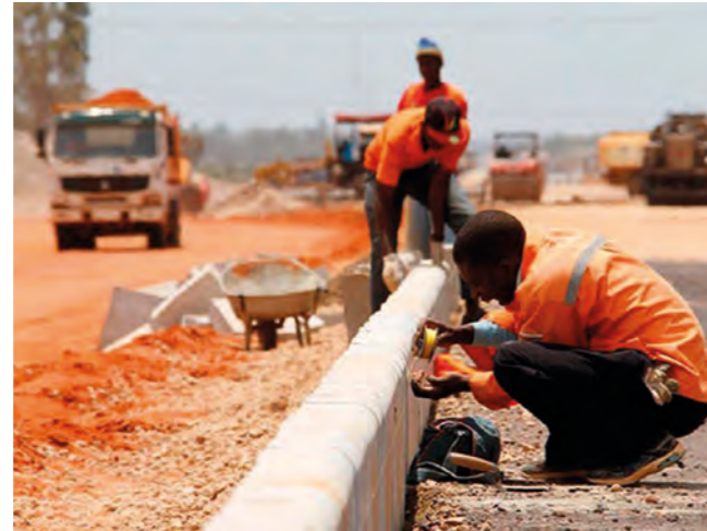
Connecting Nigeria by increasing network of roads.
