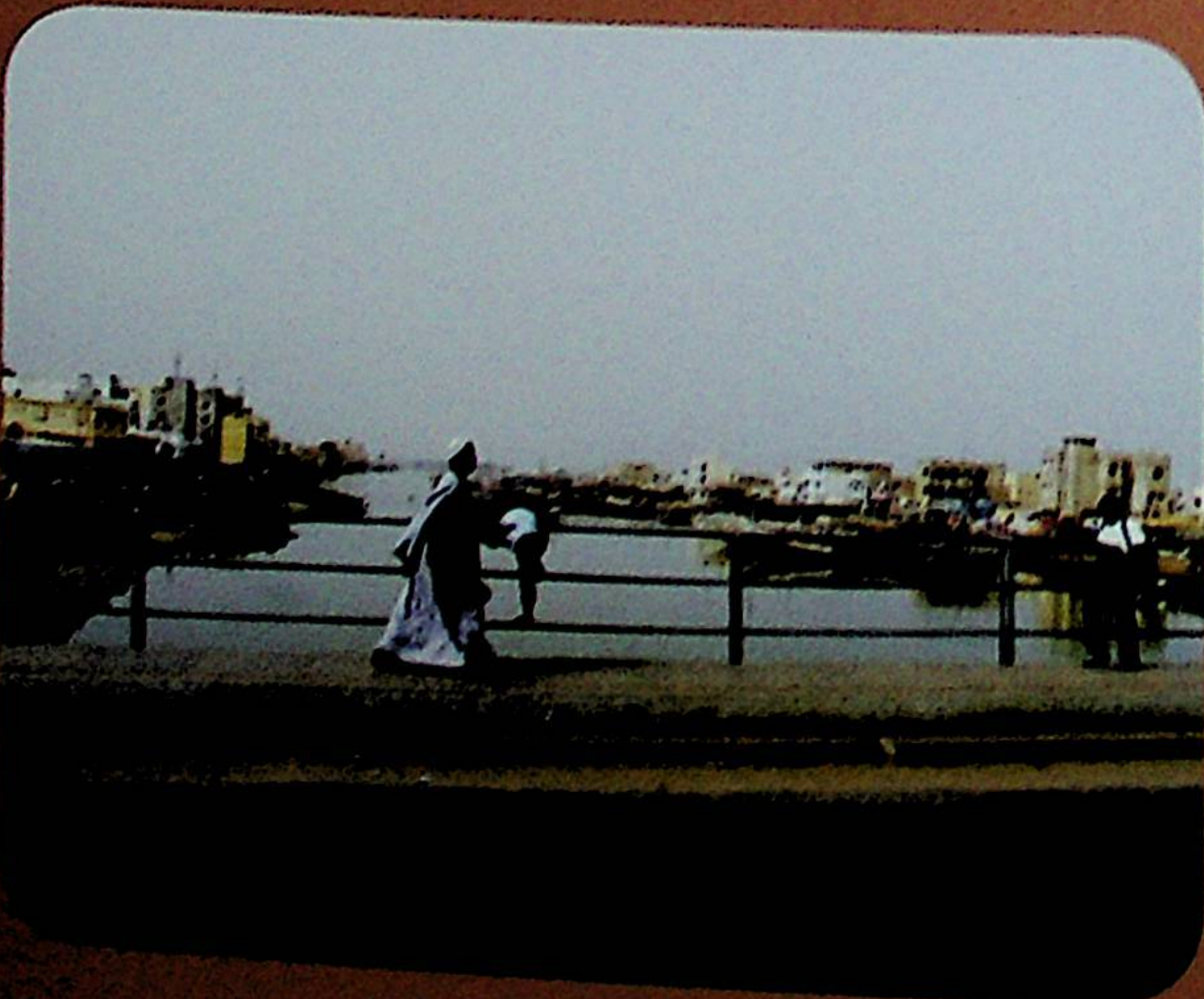
Malick Gaye Bridge, Saint-Louis
