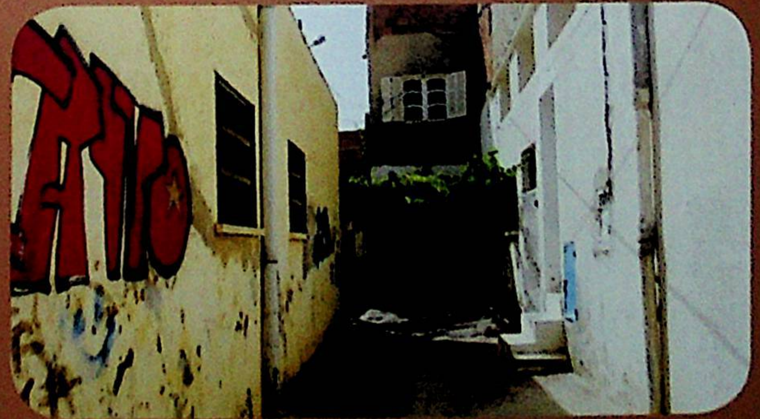
Rehabilitation of a working-class neighborhood in the suburbs of Sfax
