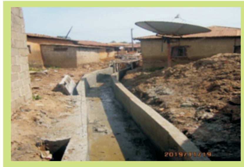
ON- GOING REHABILITATION OF ZUNGERU TOWNSHIP ROADS
