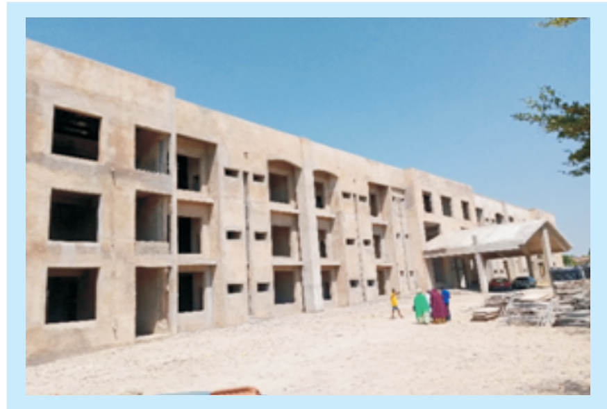
ON-GOING EXTENSION OF HOUSE OF ASSEMBLY COMPLEX
