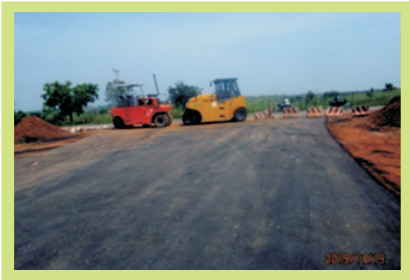
ON- GOING REHABILITATION OF ZUNGERU TOWNSHIP ROADS
