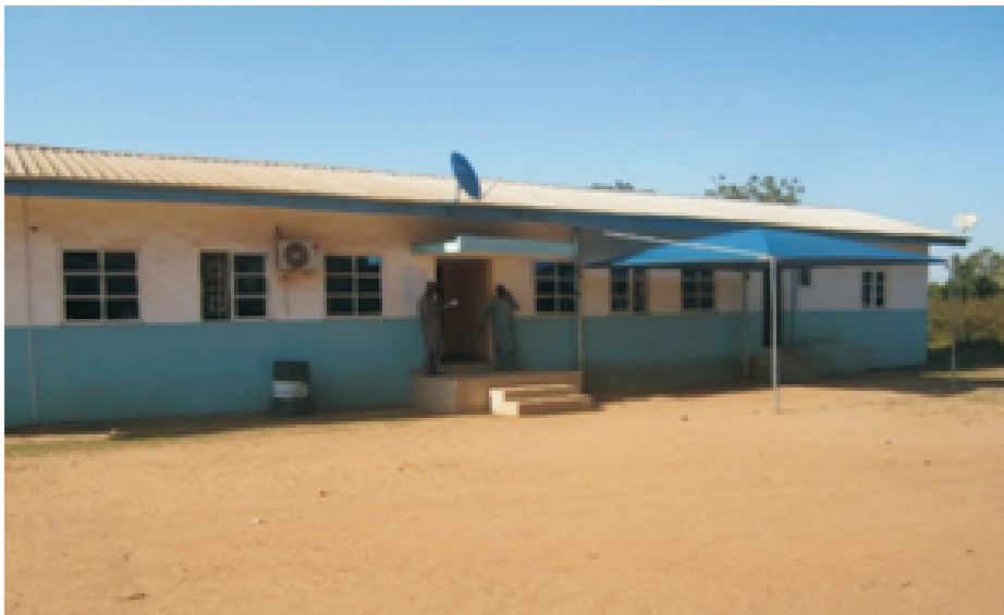
RENOVATION OF HIGH COURT OF JUSTICE, KONTAGORA
