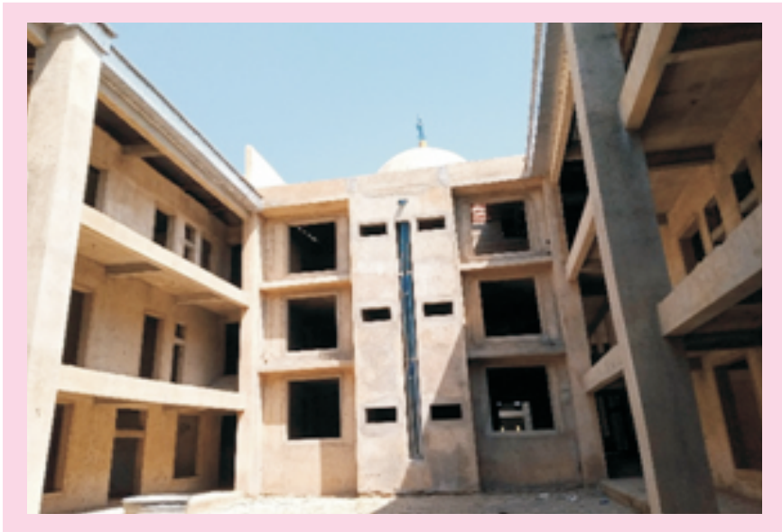
ON-GOING EXTENSION OF HOUSE OF ASSEMBLY COMPLEX
