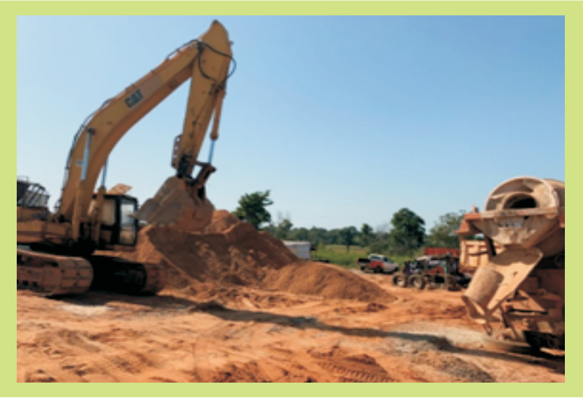
ON-GOING CONSTRUCTION/REHABILITATION OF FELLIGI-SHAFIN ROAD (12.7KM)
