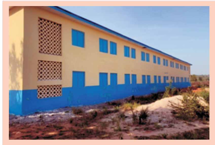
CONSTRUCTION OF HIGH RISE BUILDING AT MOHAMMED KOBO PRIMARY SCHOOL, LAPAI
