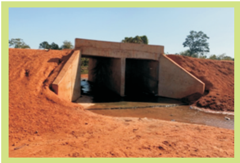
ON-GOING CONSTRUCTION/REHABILITATION OF FELLIGI-SHAFIN ROAD (12.7KM)
