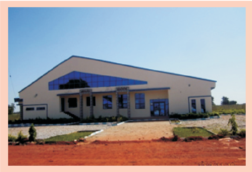
CONSTRUCTION OF AUDITORIUM AND A BLOCK OF 3 CLASSROOM AT COLLEGE OF NURSING KONTAGORA
