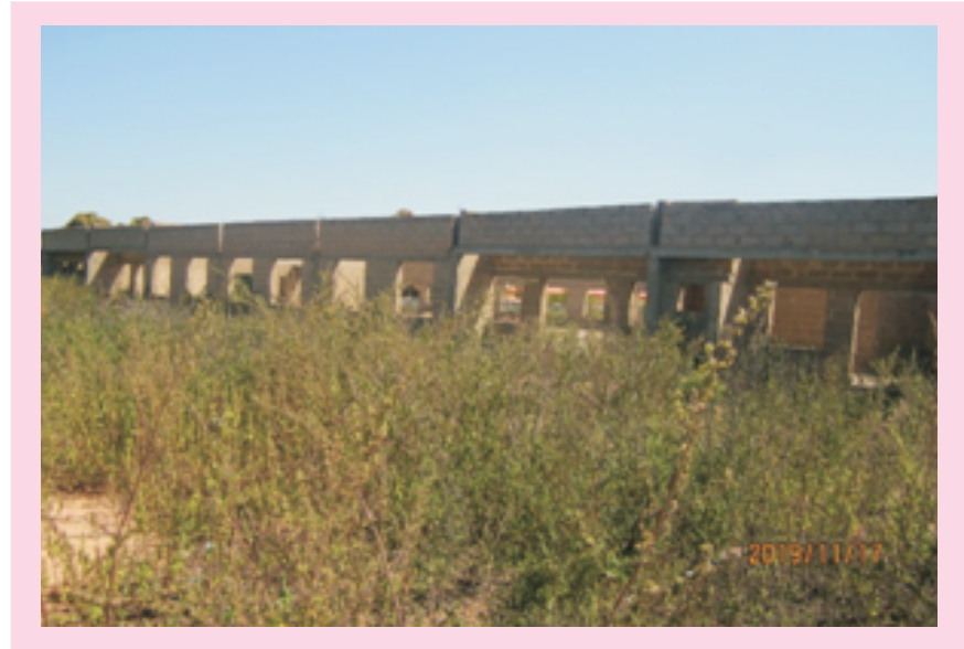
CONSTRUCTION OF ADDITIONAL STRUCTURES AT GOVERNMENT LODGE, KONTAGORA
