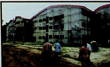
Construction Site at 80 percent completion
