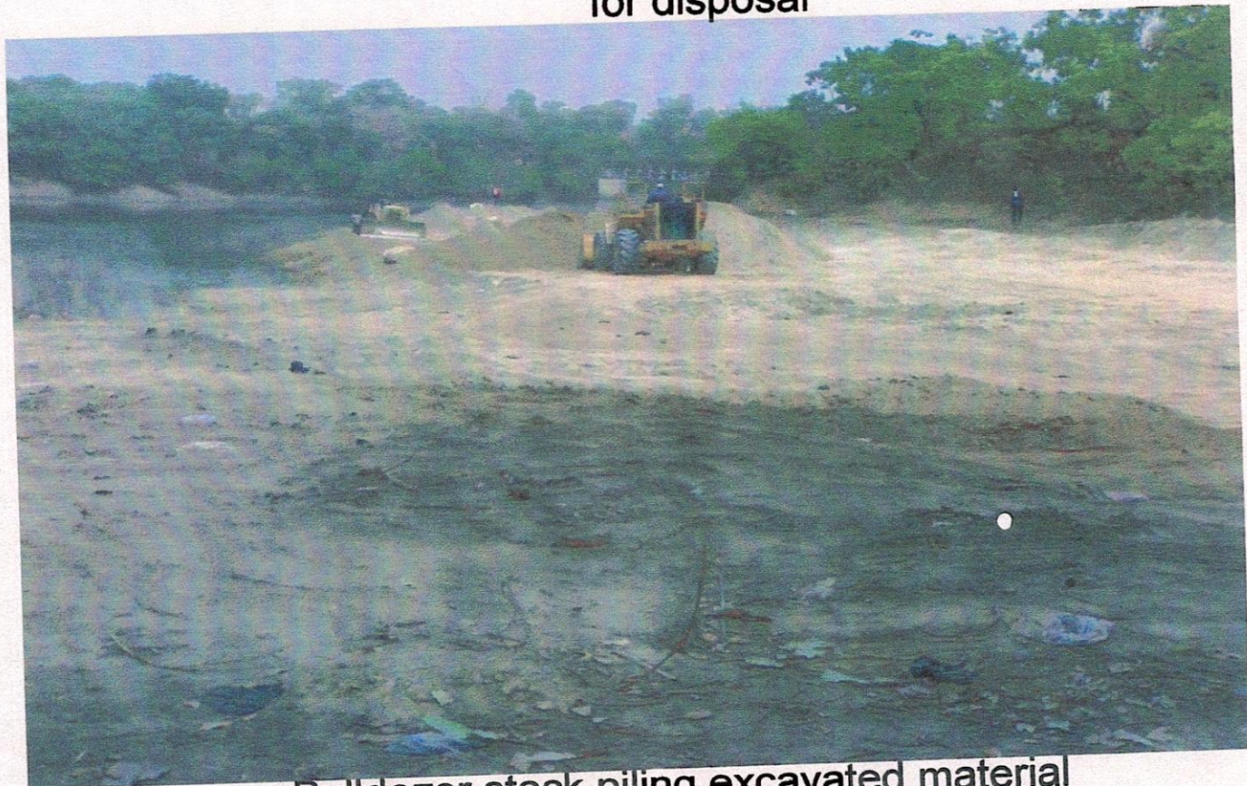
Pay loader loading tipper with excavated materials for disposal
