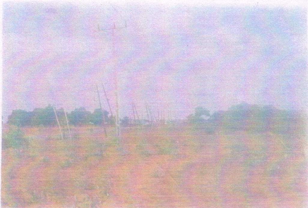
REPLACEMENT OF WOODEN ELECTRIC POLES WITH CONCRETE POLES FROM CITY GATE TO CHANCHAGA WATER WORKS
