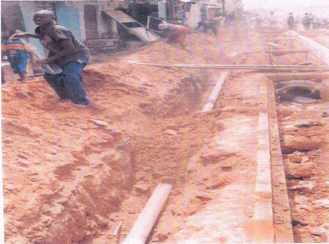
LAYING OF 160/100mm Dia. uPVC PIPES
