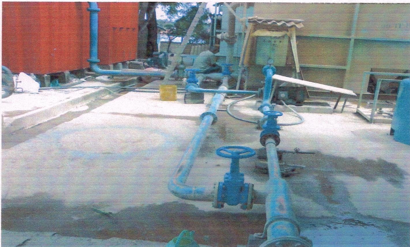
Picture showing pipe connection to the distribution lines
