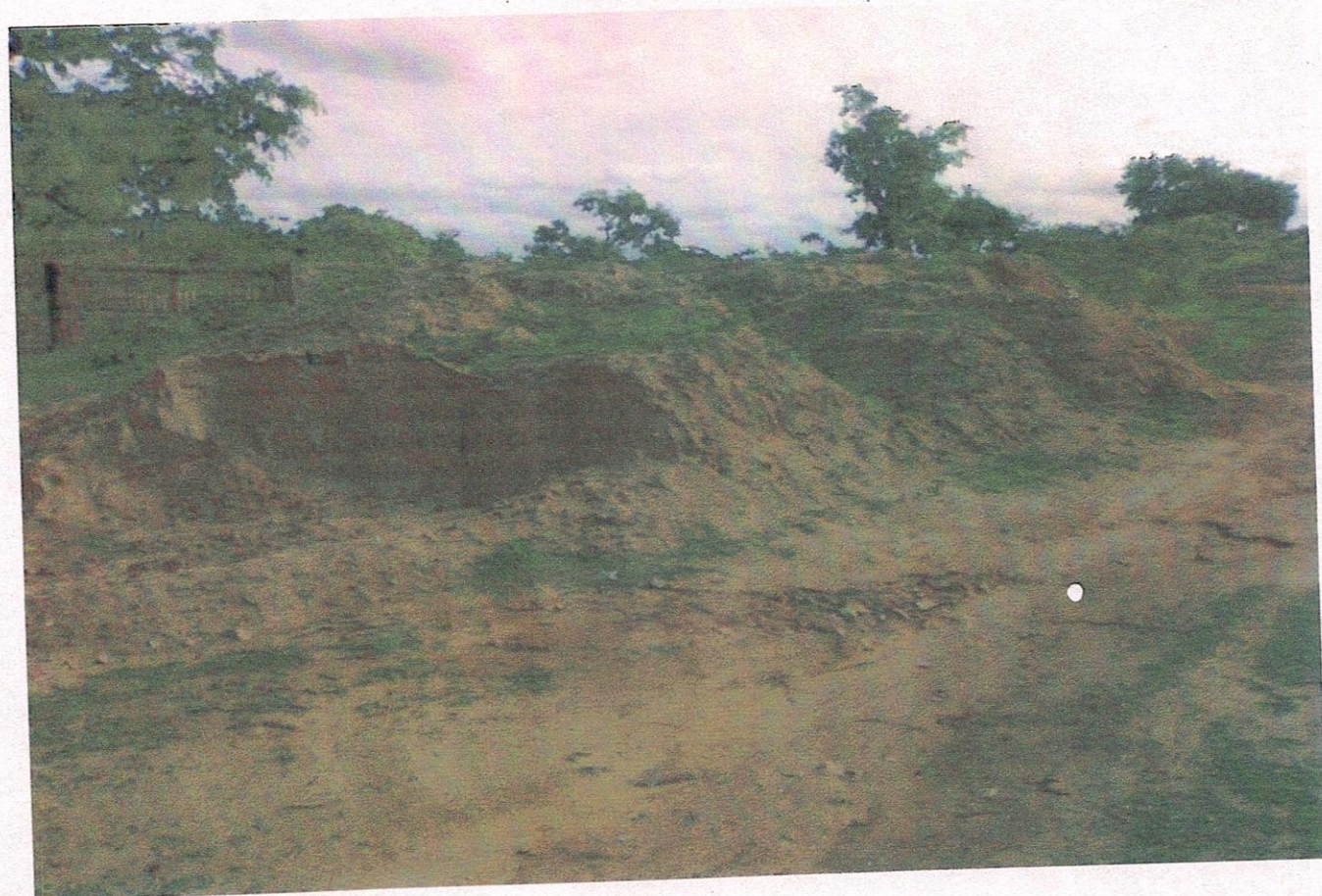
Pictures showing deposited De-silted materials from dam area
