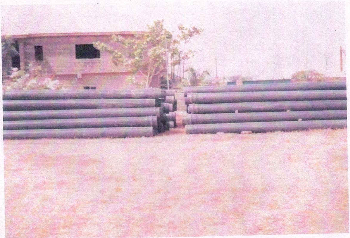
400mm PIPES FOR RELOCATION WORKS
