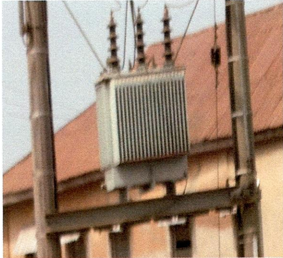
Oye LG- Siemens Transformer 33/0.415KV In front of St. John's Anglican Church, Ilupeju.
