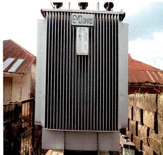
Ise-Orun LG-200KVA 33/0.415KV Emo-Ohrid Transformer, S.N.338490. Beside Kingdom Hall Obada, Ekiti
