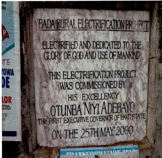
Ise-Orun LG-200KVA 33/0.415KV A Plague for Emo-Ohrid Transformer, S.N.338490. Beside Kingdom Hall Obada, Ekiti
