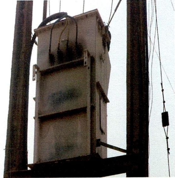
Oye LG ...KVA 33/0.415KV Simens Transformer S.N., In front of Onirare Palace
