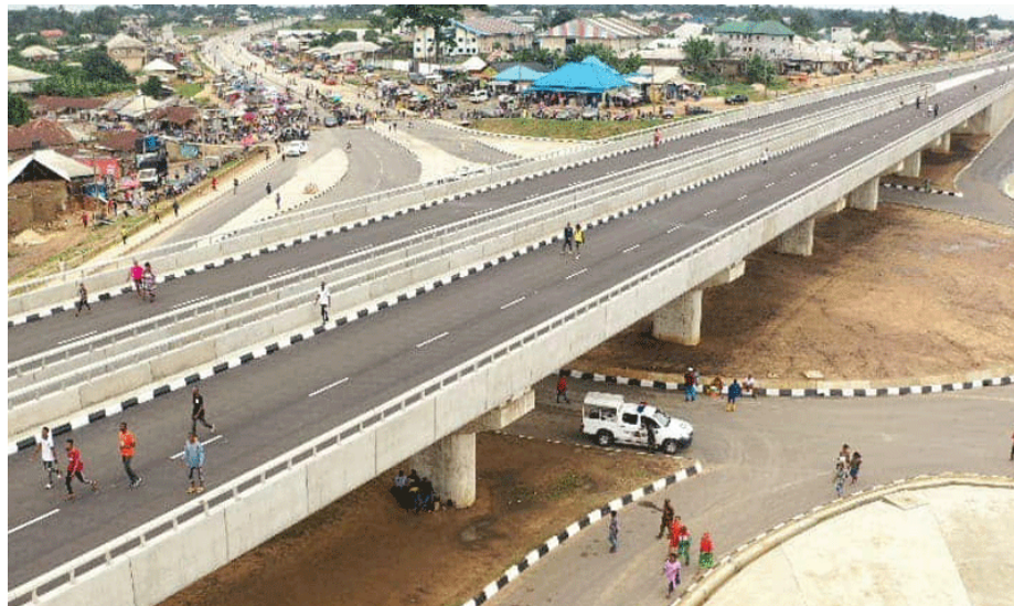
The new Oku Iboku flyover
