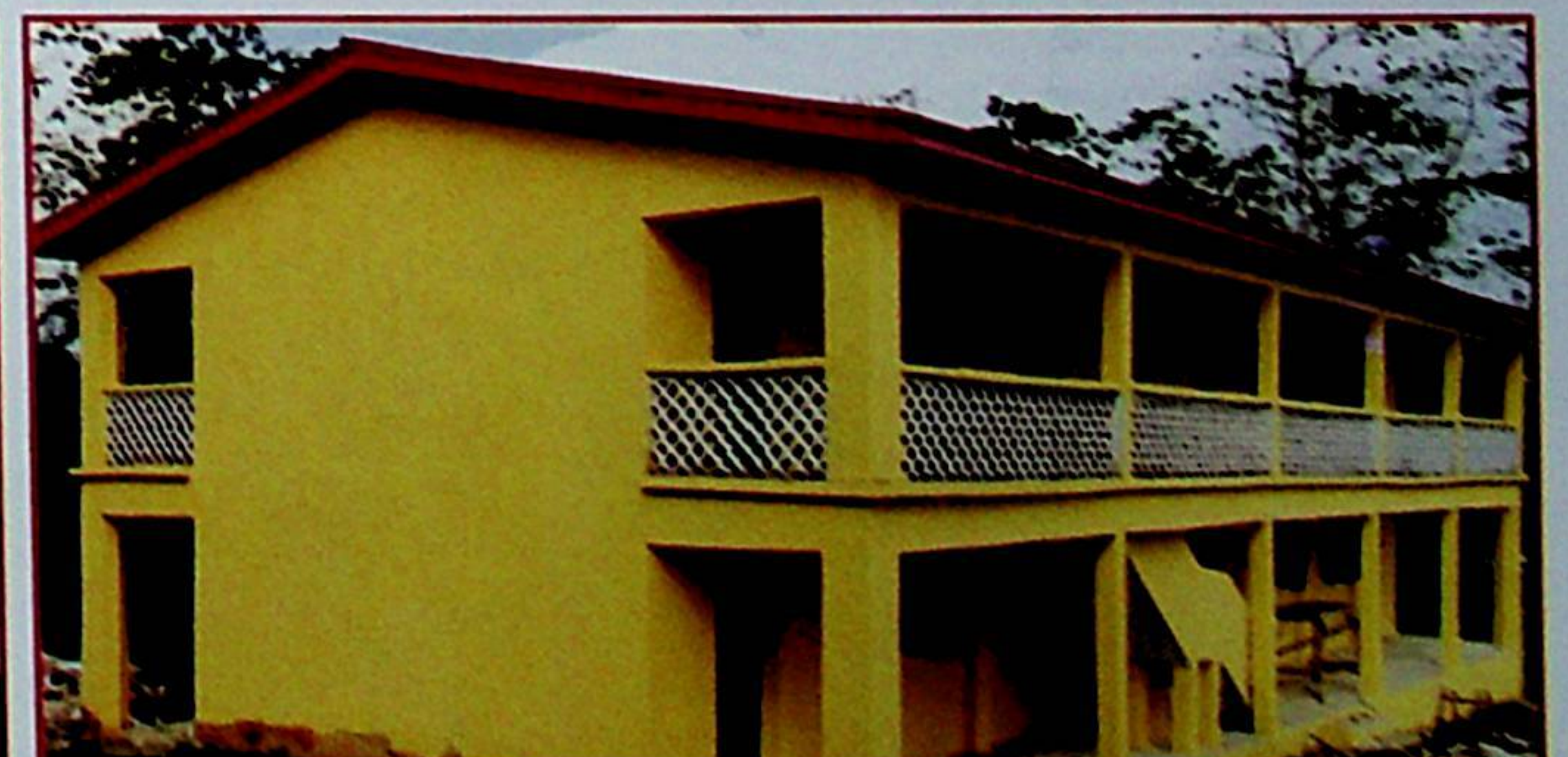
Corpus Christi, Ilawe-Ekiti, one of the one hundred Secondary Schools renovated by the present administration
