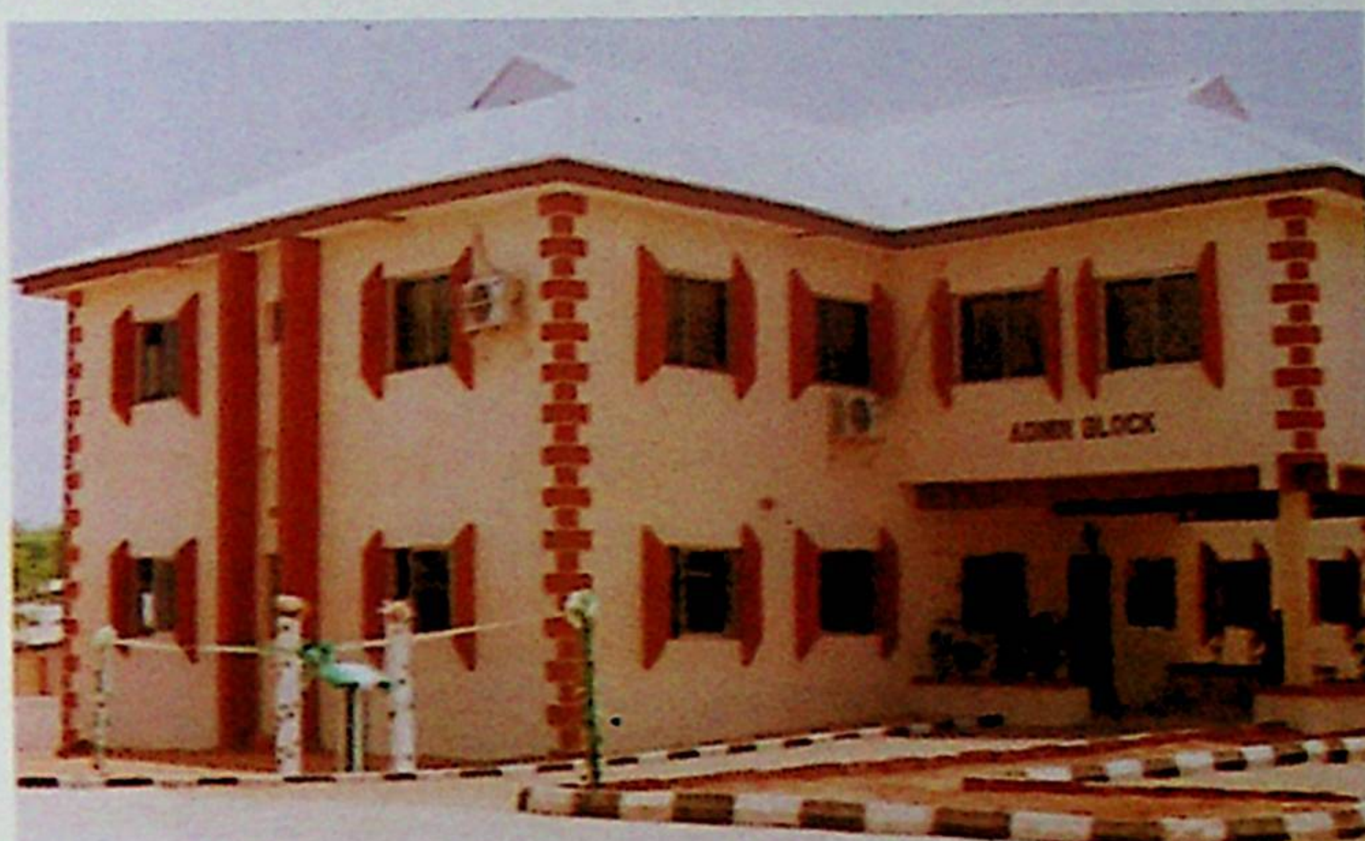
ETF Funded Gombe Community Education Resource Centre, Gombe
