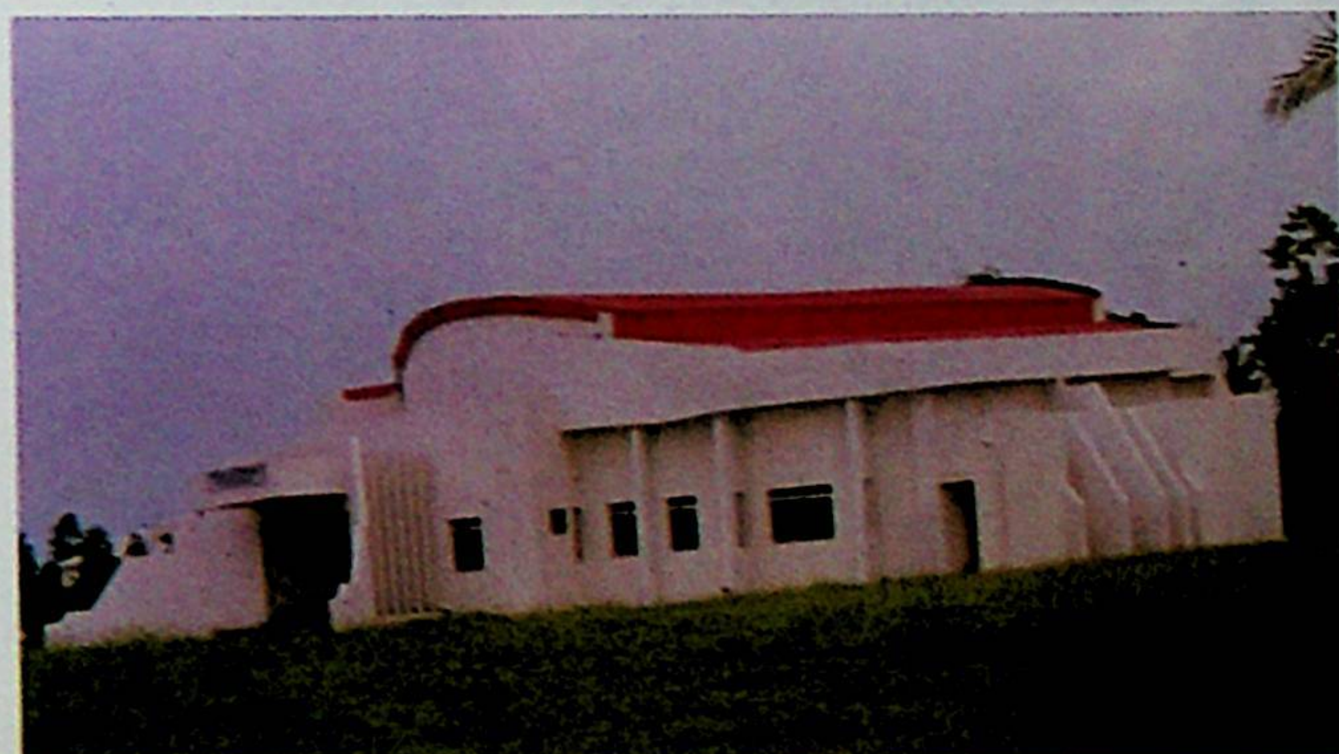
Multi Purpose Hall, Federal Polytechnic Ado Ekiti, Ekiti State.
