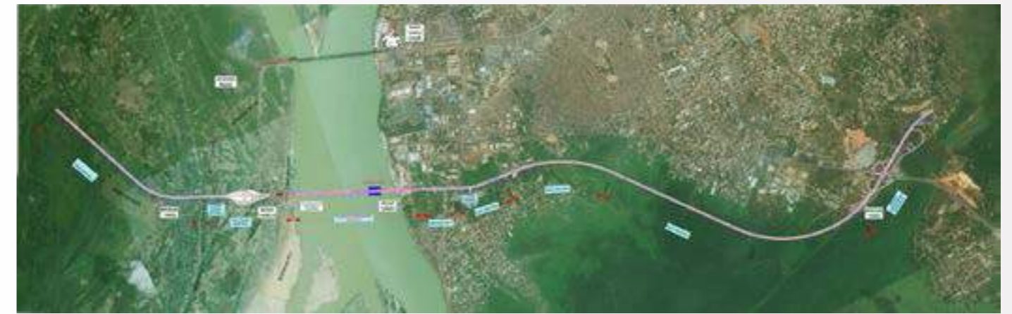
Second Niger bridge
