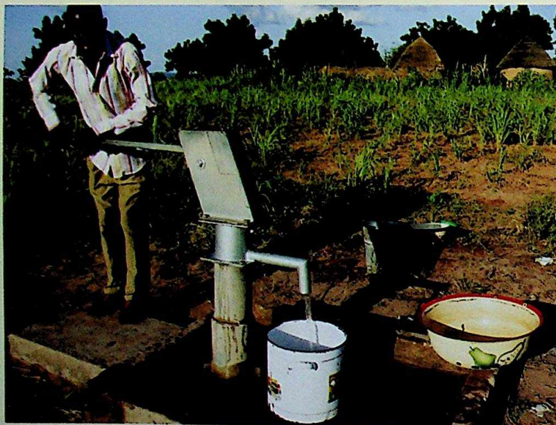
Rehabilitation of water pumps and boreholes supported by the TY Danjuma Foundation in Taraba State'.
