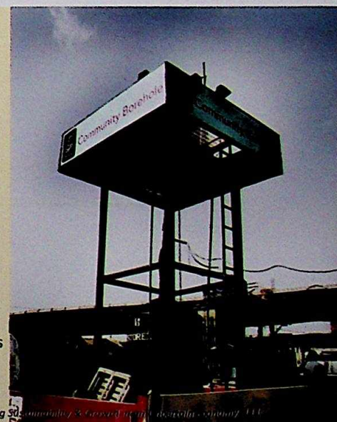
Zain water project in Iponri Market, Lagos
