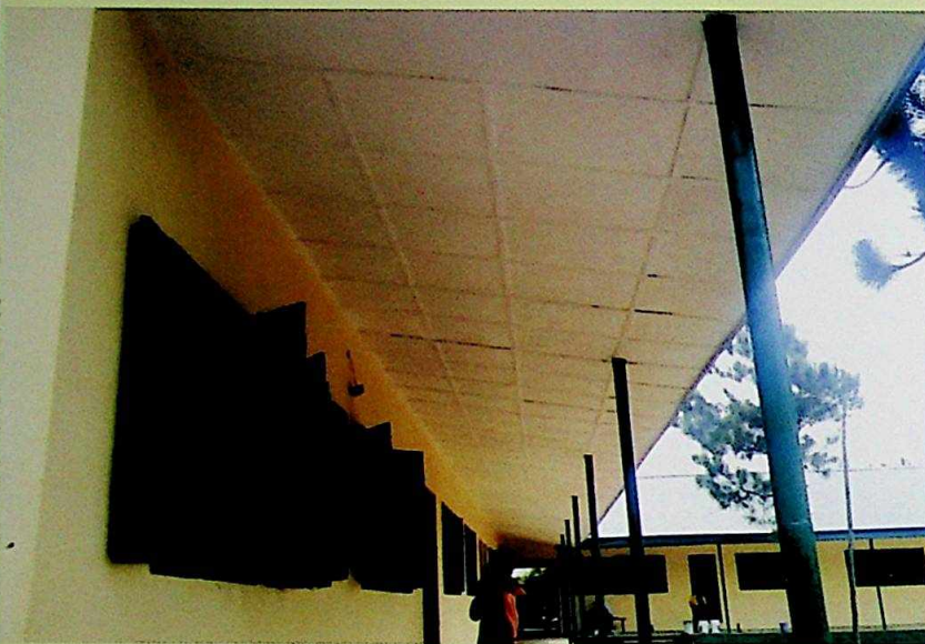
Painting of verandah completed
