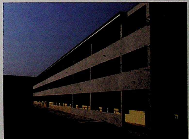
Completed blocks of residential accommodation for officers in Abuja
