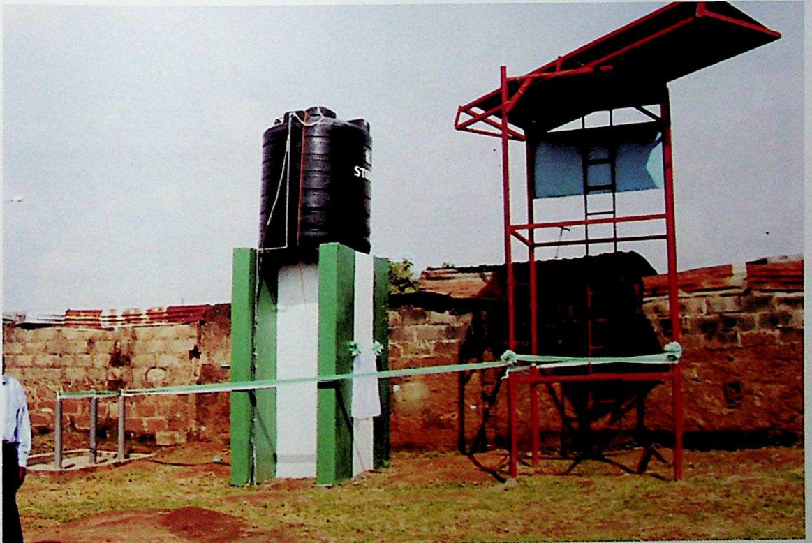
The Solar Water borehole system
