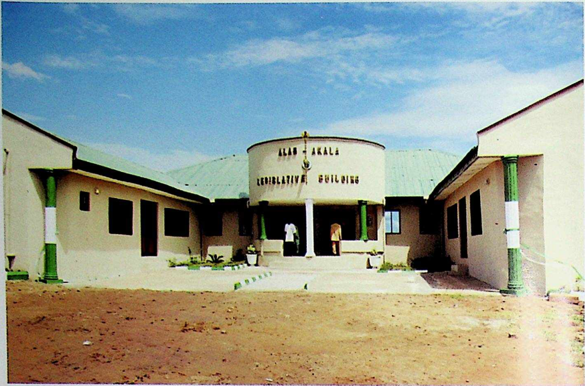
Alao-Akala Legislative Building: A magnificent edifice in honour of a worthy son of the soil at the Ogbomosho South Local Government Secretariat.
