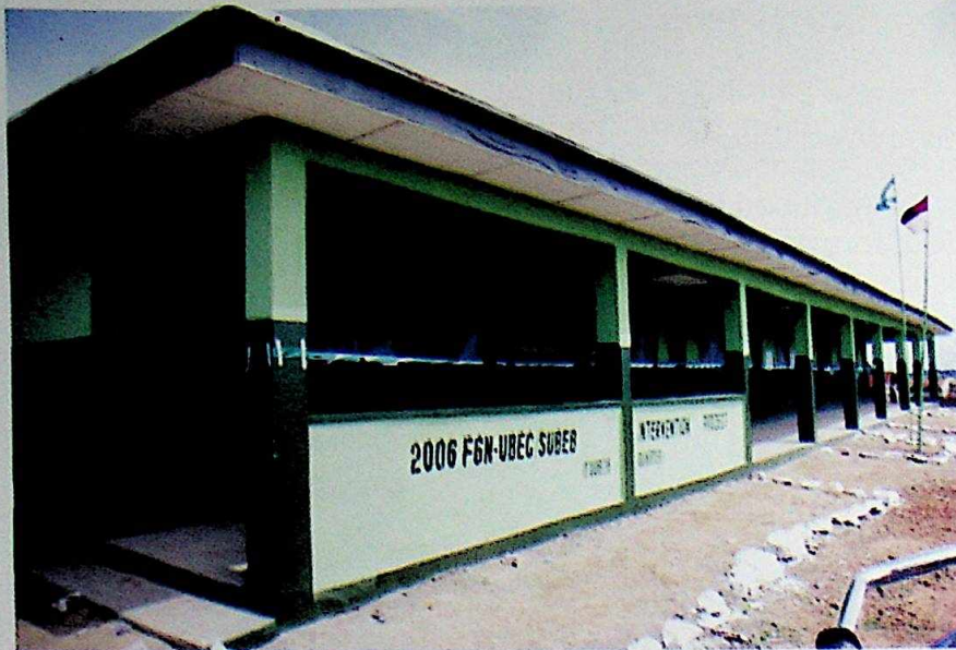
FGN-UBEC/SUBEB project at Osupa Baptist Primary School, Ogbomoso
