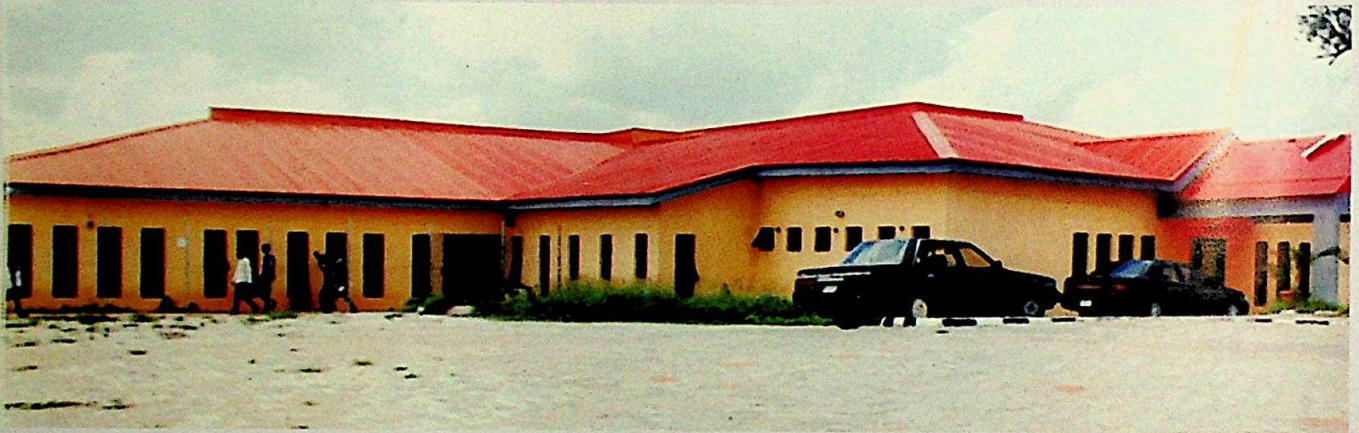
Centre of Excellence in software engineering building at Osun State Polytechnic, Iree.
