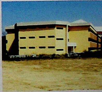
College Building at the UNIOSUN, Ikire Campus
