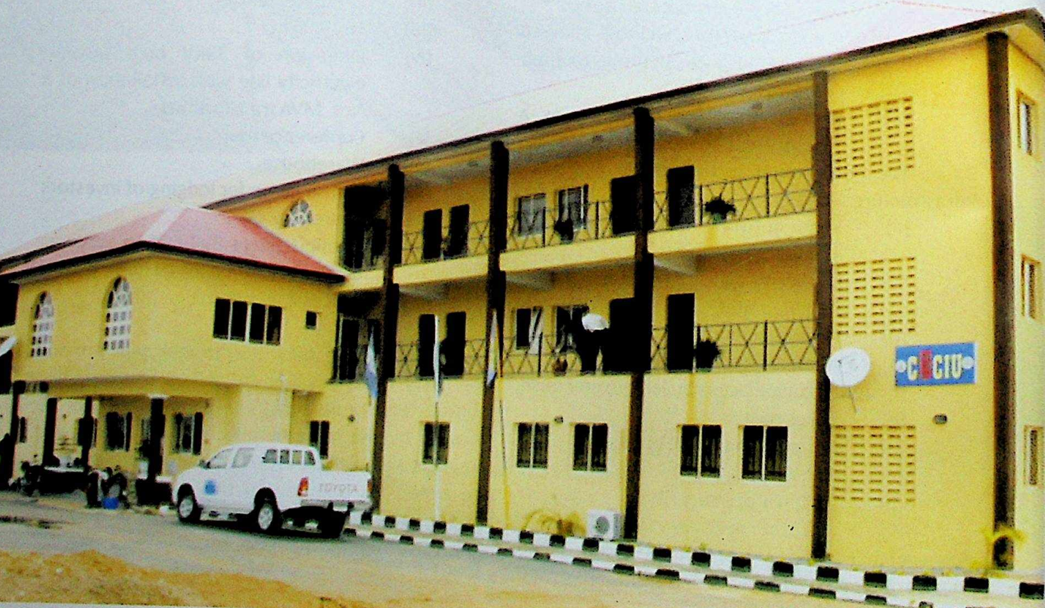
Newly constructed Centre for Black Culture and International Understanding, Osogbo.
