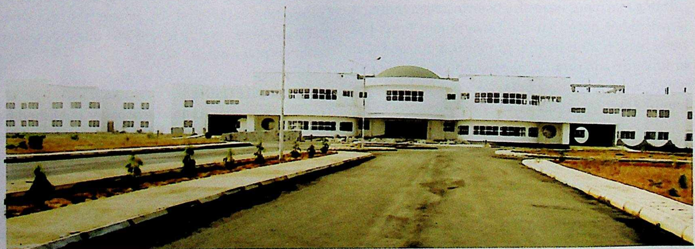
Newly completed and equipped REALITY TV Station at Iwo
