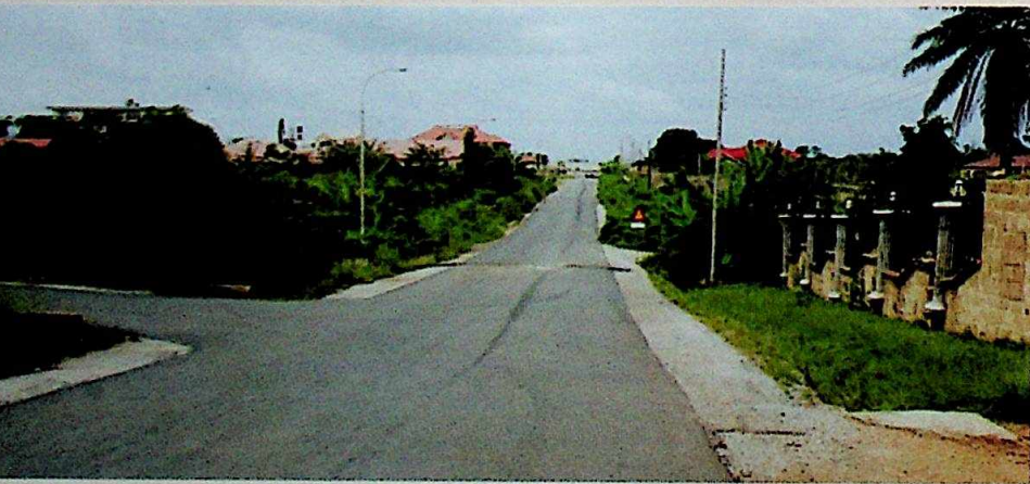
Construction of Road Network within G.R.A., Osogbo
