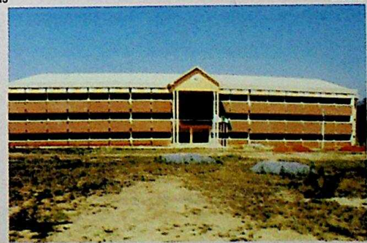
College Building at the UNIOSUN, Ejigbo Campus
