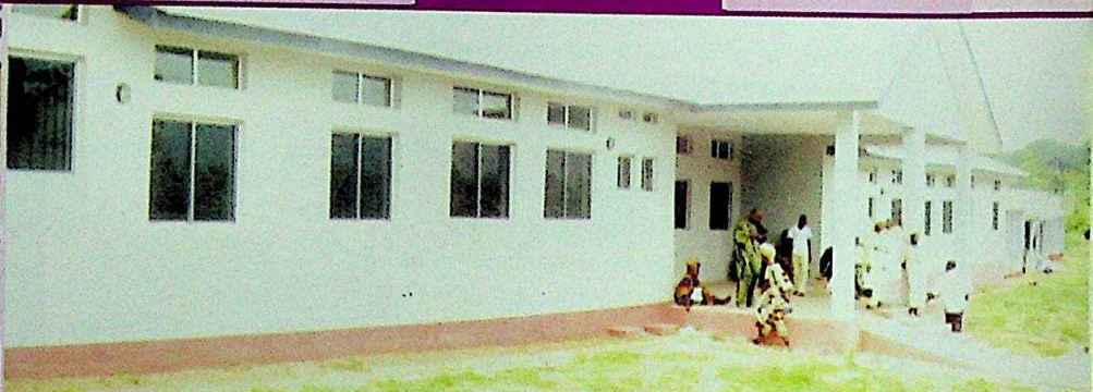
Maternity Complex at State Hospital, Asubiaro, Osogbo
