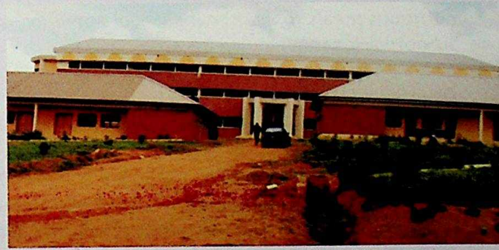
Blocks of lecture rooms at the UNIOSUN
