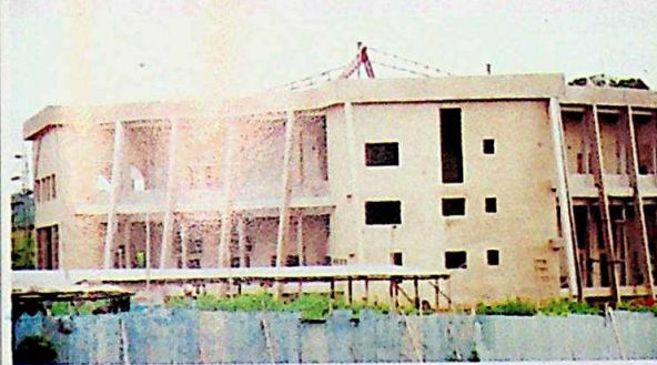
UNIOSUN Auditorium under construction
