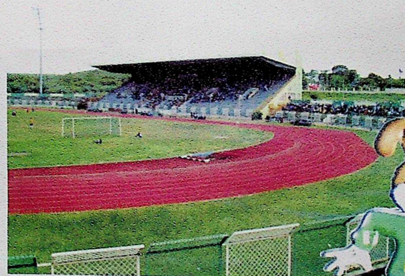
MKO Abiola Stadium, Abeokuta
