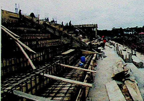
VIP Stand under construction
