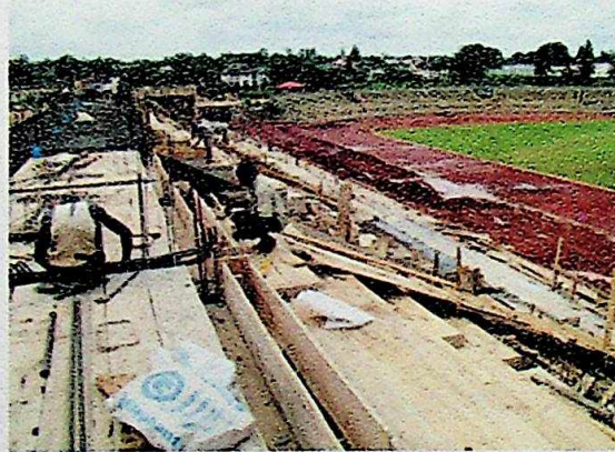
VIP Stand under construction
