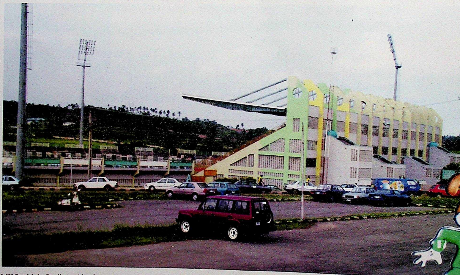
MKO Abiola Stadium, Abeokuta
