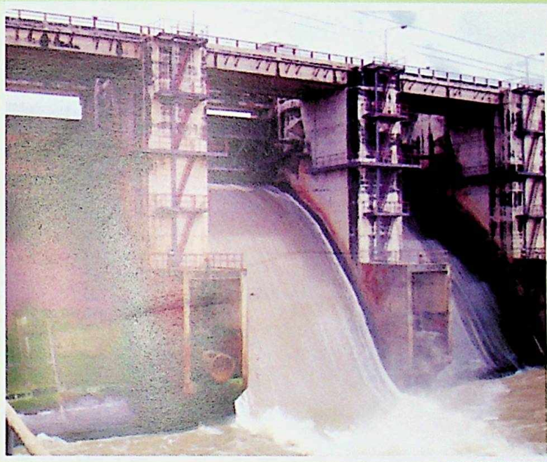
▲ Oyan Dam @ Sokoto Road
