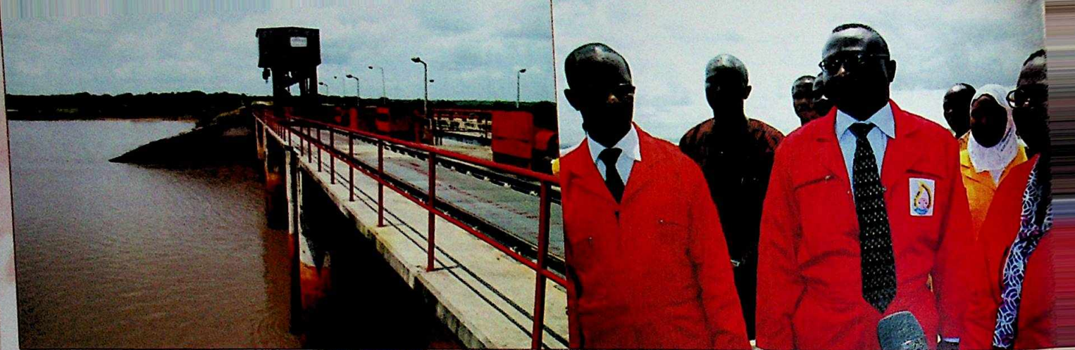
Special duties commissioner Akogun Koa Onadipe (middle) Engineer Mrs. C. Babajide (right) and an Official of the Ministry inspecting Oyan Dam
