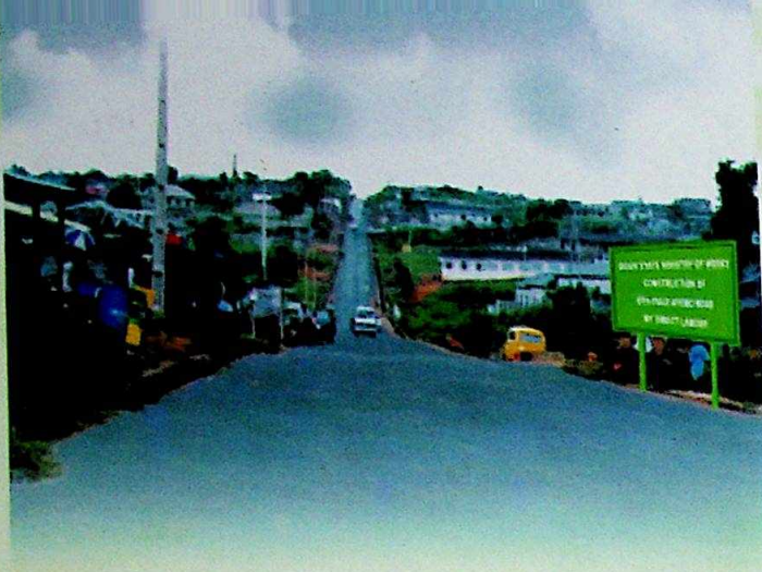
The newly constructed Sam Ewang Road, Idi-Aba, Abeokuta
