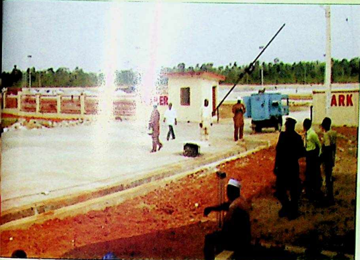
Construction of Sagamu Trailer Park
