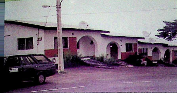
OGD Quadrangle, Abeokuta: Blocks of Studio constructed to provide accommodation for government functionaries
