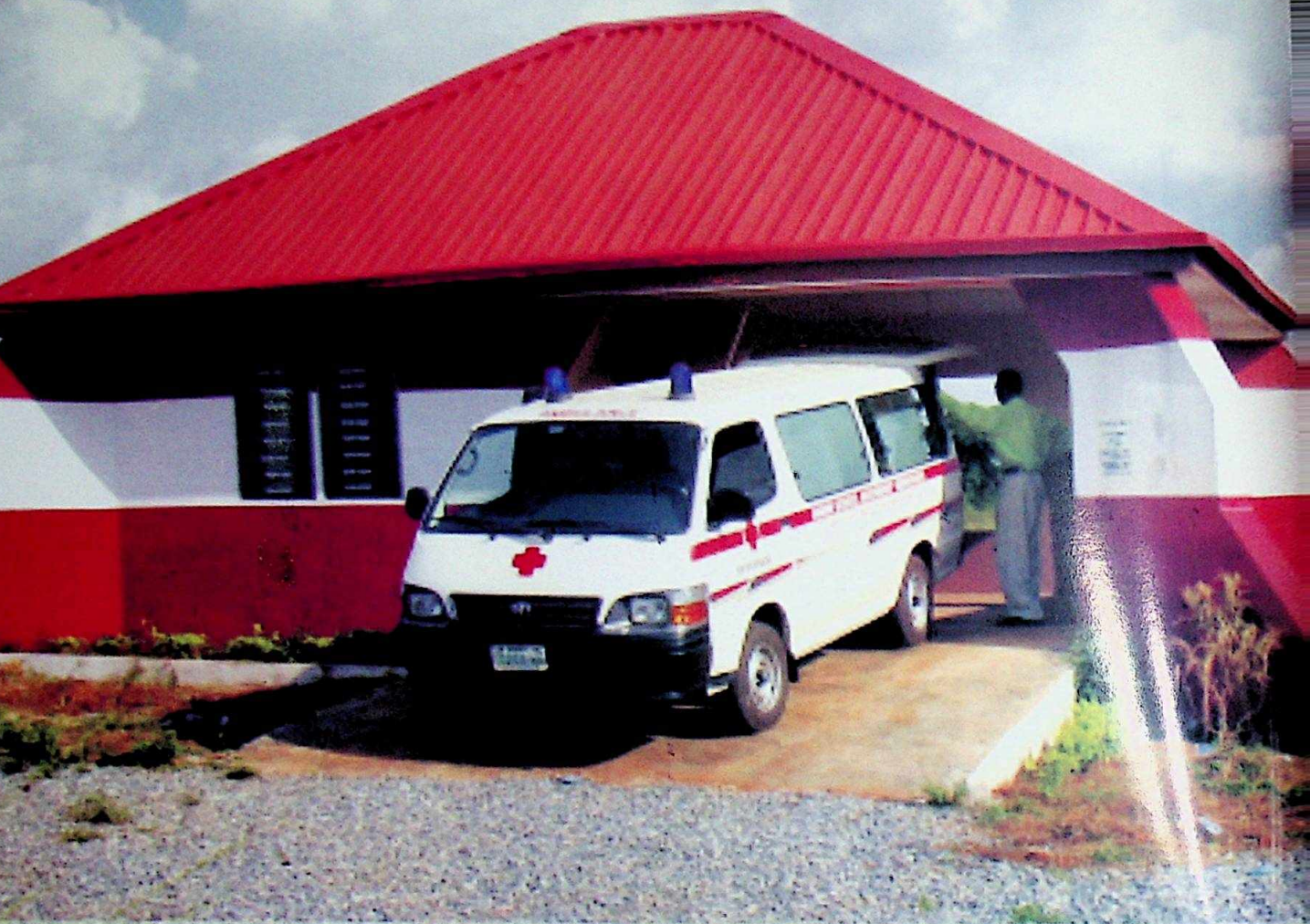
OGSAS point at Shagamu Roundabout
