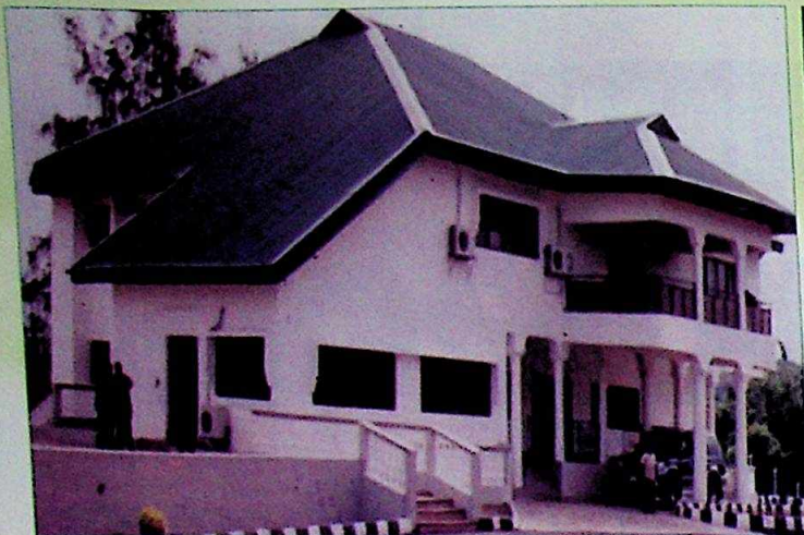
The completed Deputy Governor's Lodge at GRA Abeokuta
