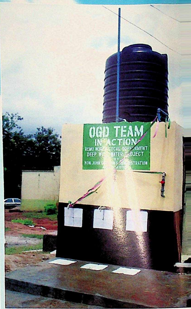
A community borehole project ready for commissioning at Isara
