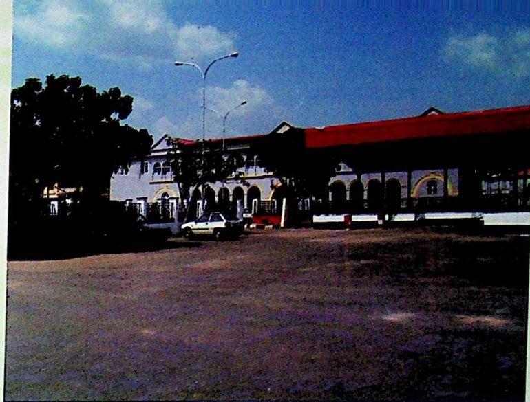
Complete Rehabilitation of Ake Palace Ground
