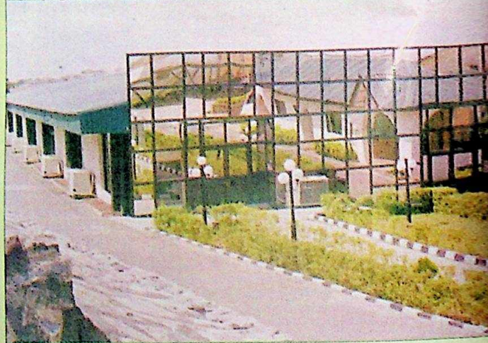
The Valley View Auditorium built within eight (8) weeks
