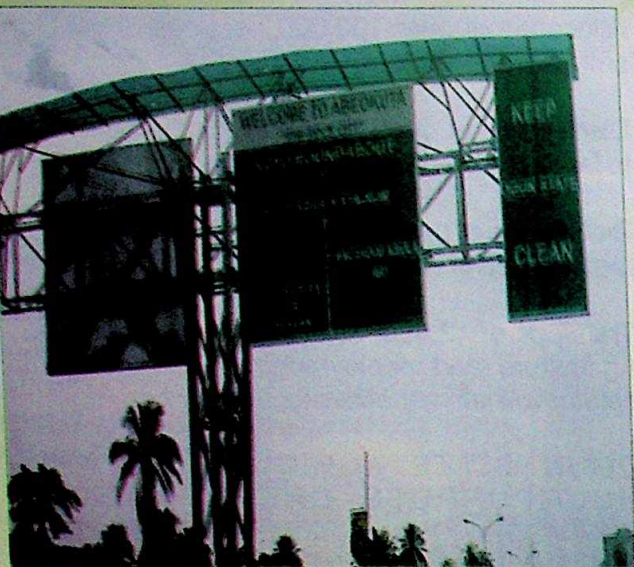
Strategic road signs on Abeokuta/Shagamu Expressway.
