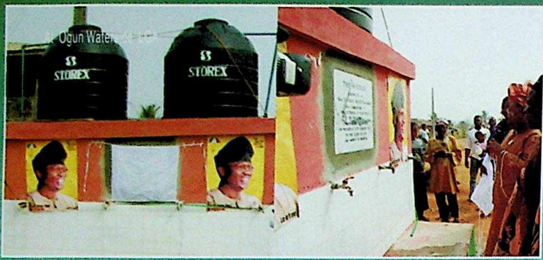
Water project set for commissioning.
