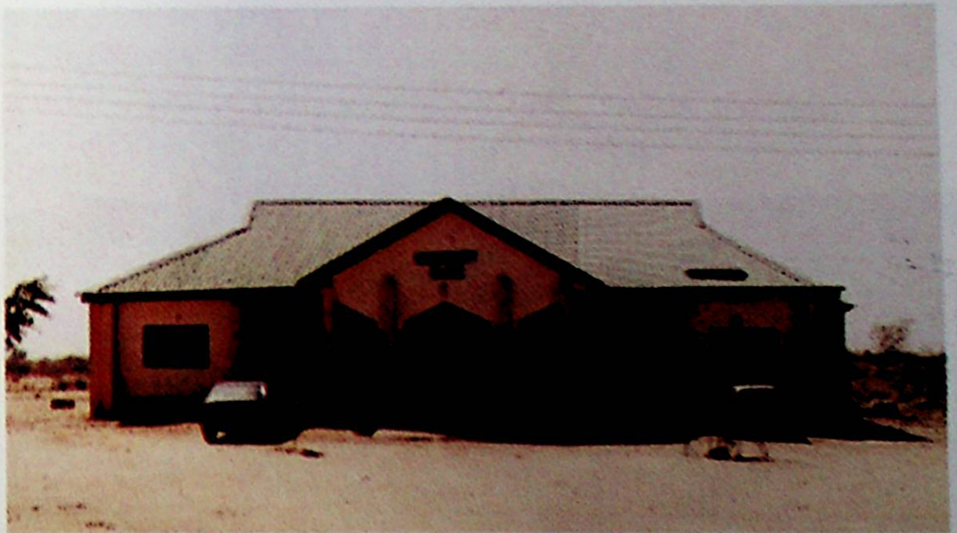
University clinic situated a few metres away from student hostels
