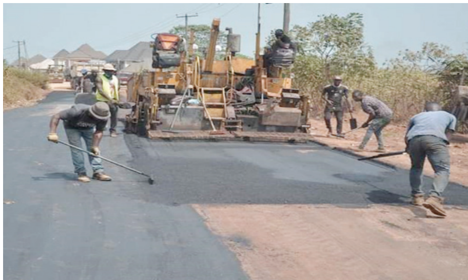
One of the multiple road projects in Amuzukwu
