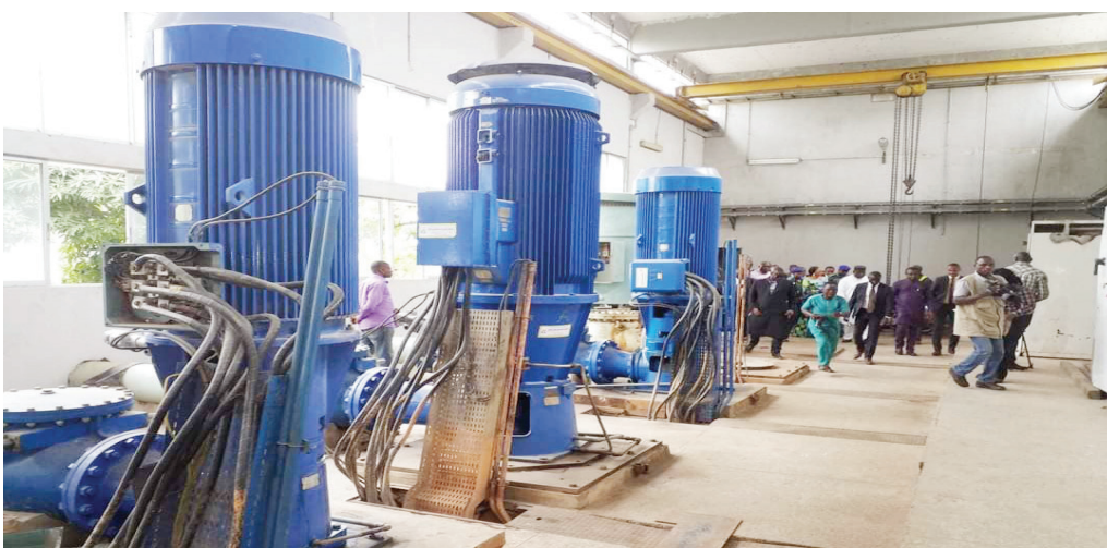
Enugu Solar powered Boreholes
