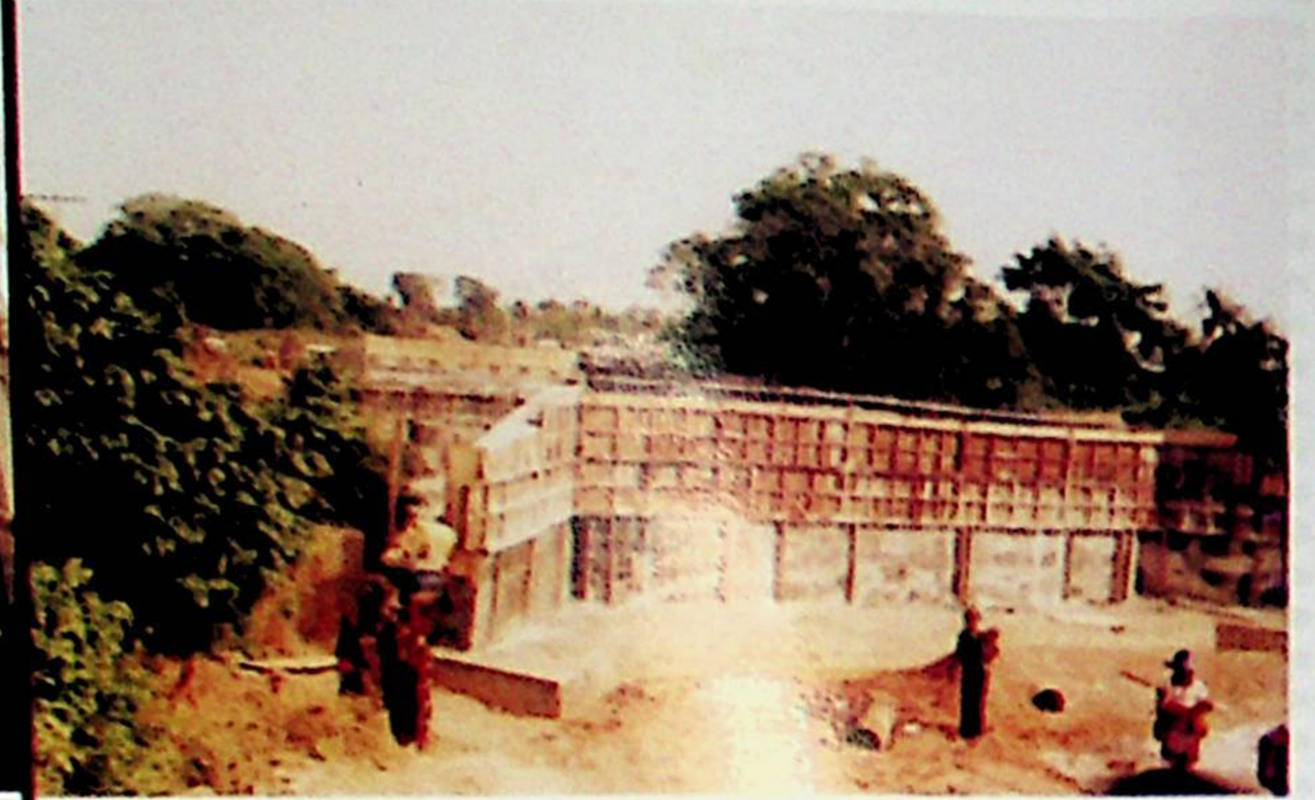
One of the new unity bridge in Ivo LGA
