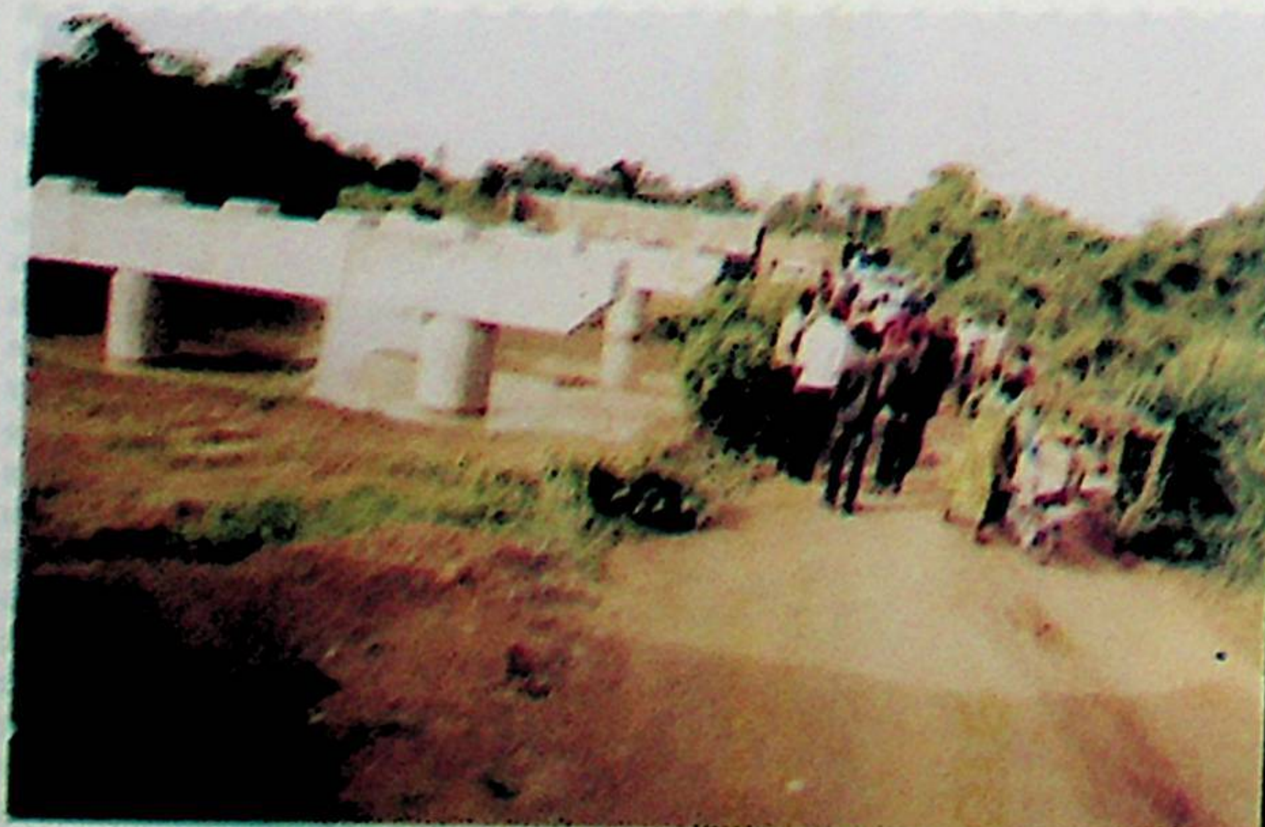
One of the new unity bridge at Odomowo Ivo LGA
