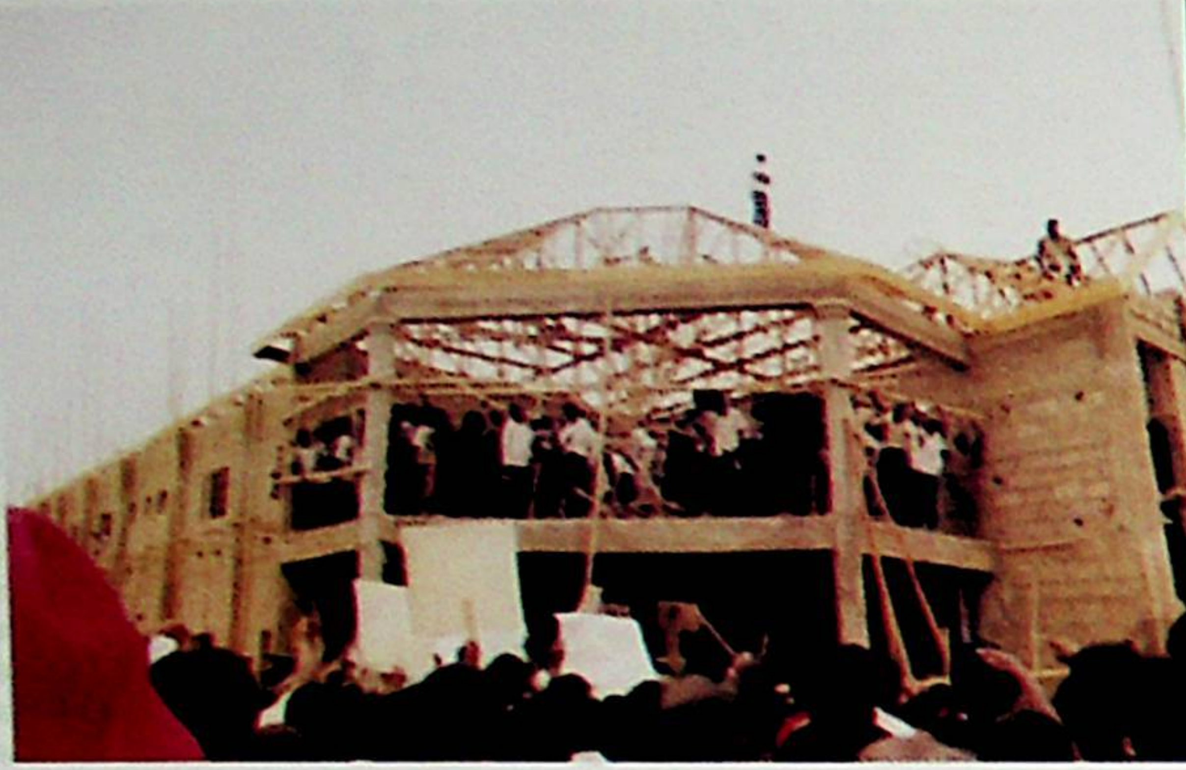
One of the new building projects at Ikwo College of Education
