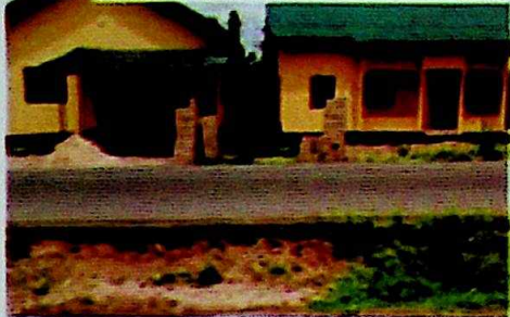
BULU APELEBIRI HEALTH CENTRE AND NURSES QUARTERS AFTER THE RENOVATION
