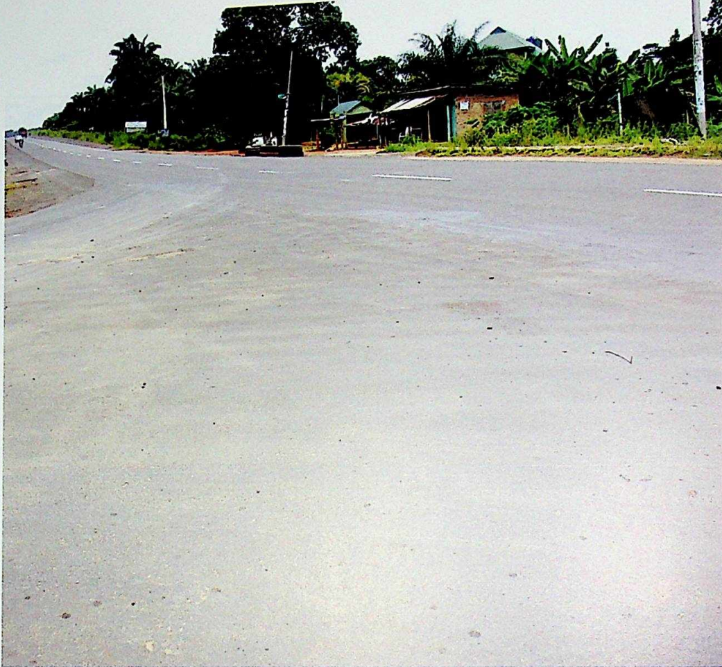
Lilu Road (under construction)
