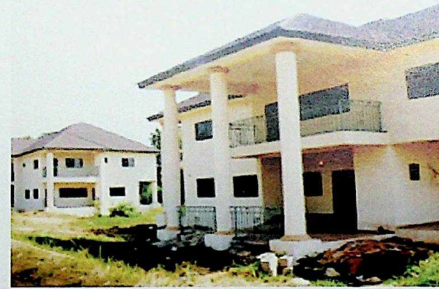
Two of the many buildings at Judges' Quarters, Onitsha, the first ever in the State
