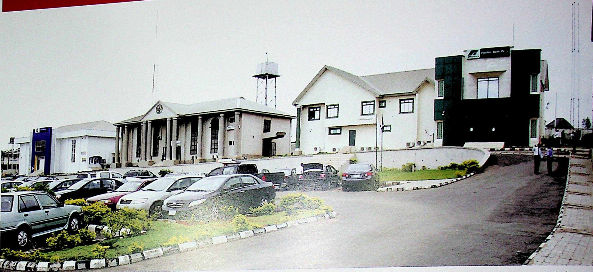
The new business park in Onitsha, part of government's programme to establish modern business parks in commercial centres to promote commerce in the State
