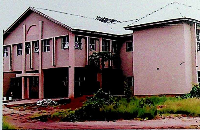
Completed New Aguata Zonal Office of the Ministry of Justice
