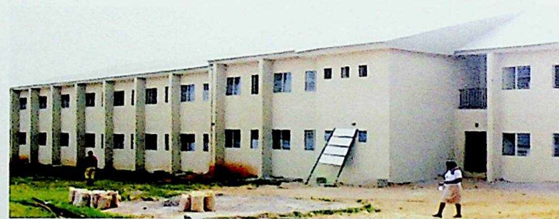
A new 200-bed hostel at the School of Health Technology, Obosi
