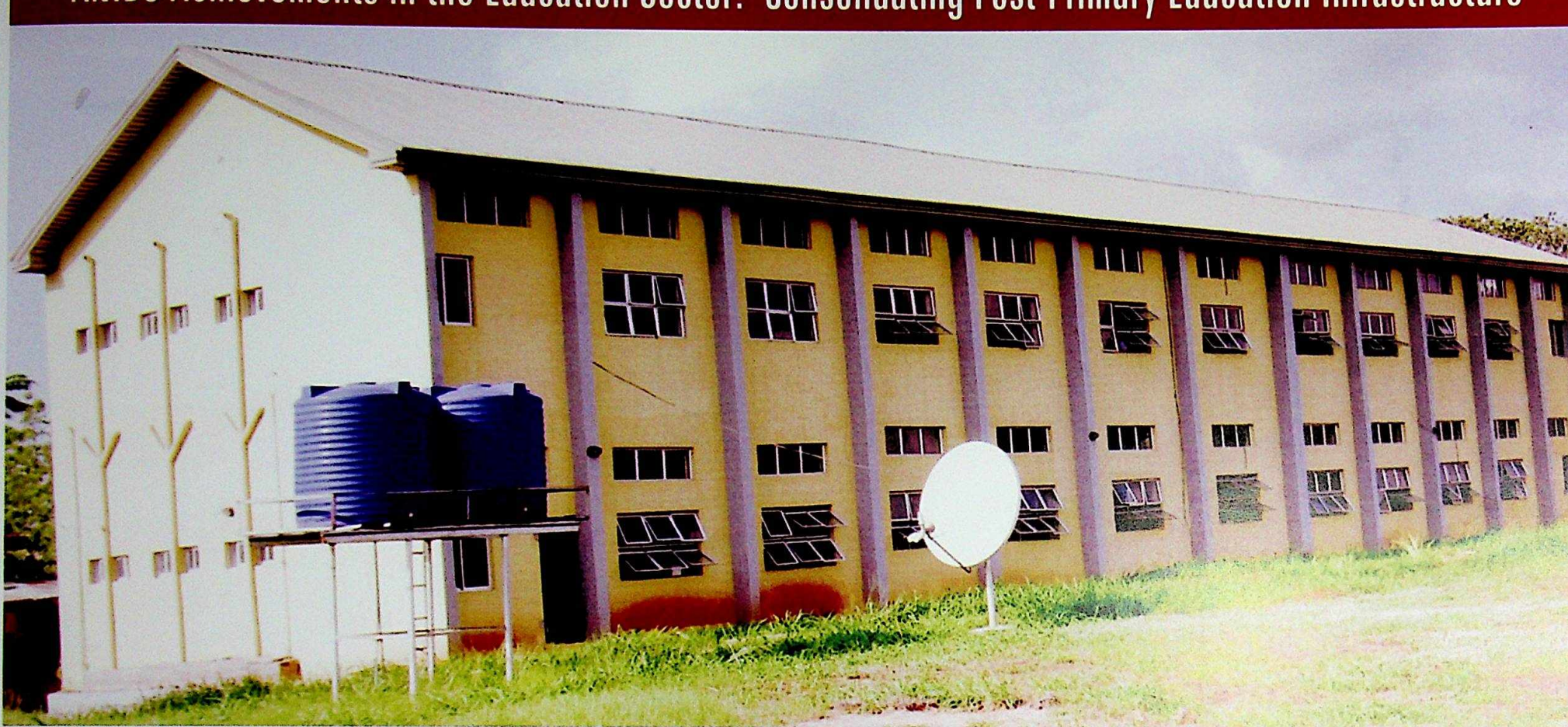
A new classroom block at Nwafor Orizu College of Education, Nsugbe
