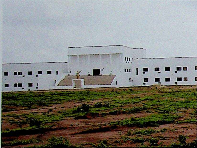
Completed new Nnewi High Court Building
