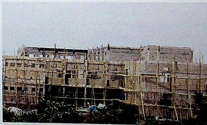
Faculty of Management Sciences building under construction at
