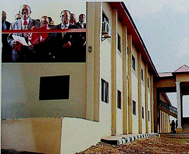
High Court building Onitsha. Inset: Governor Peter Obi during the inauguration
