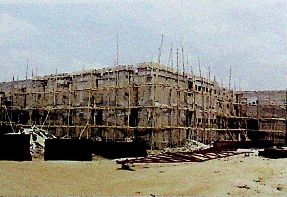
Administrative complex under construction at
