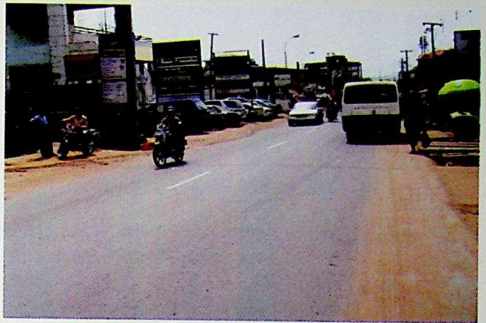
Completed Upper New Market Road, Onitsha.
