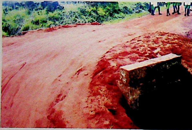
Road under construction at Dunukofia LGA
