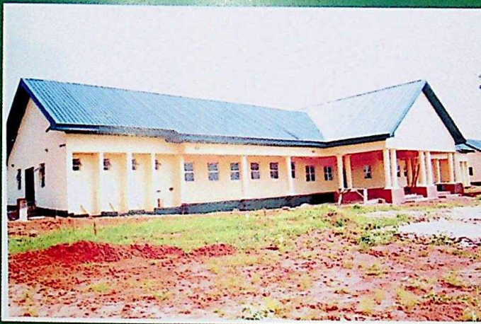
New Male Ward Complex constructed by the Obi Administration at Umuleri General Hospital
