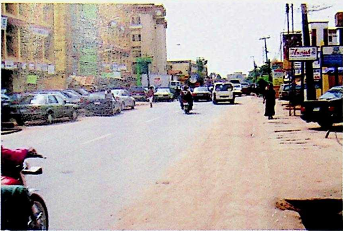
Completed Old Market Road, Onitsha.
