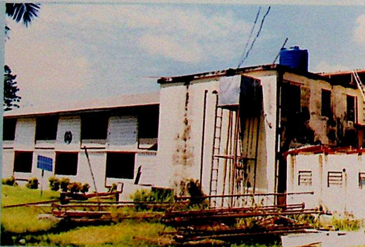
Renovated Secretariat Building, Ogbaru LGA
