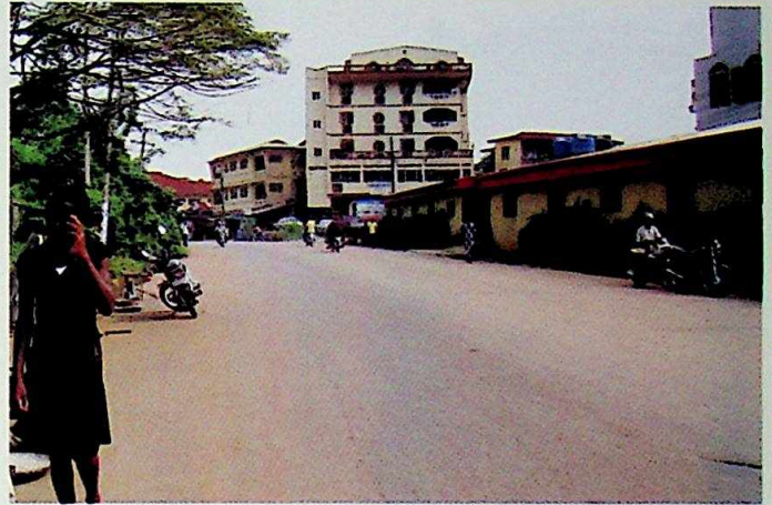
Completed Modebe Avenue, Onitsha
