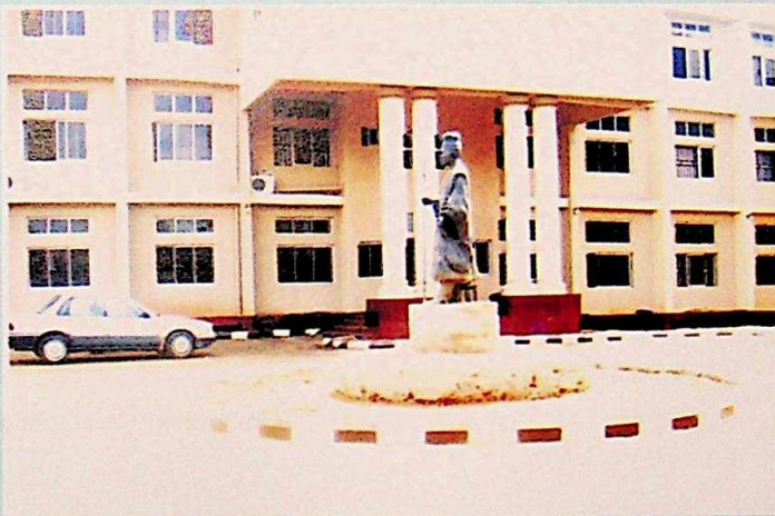
New Onitsha North Secretariat Building
