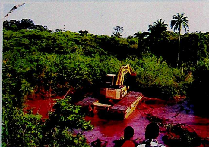
Ongoing dredging of Obizi Regional Water Scheme Uga, Aguata LGA
