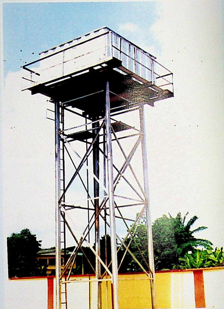
Water Borehole Project at Oyi LGA Hqtrs
