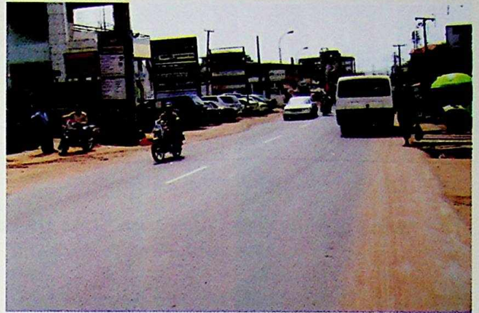
Completed Upper New Market Road, Onitsha.
