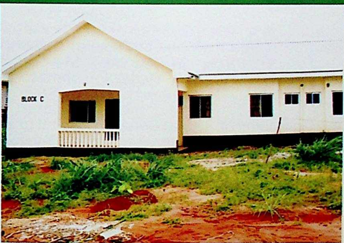
One of the newly constructed House Officers Quarters by the Obi Administration at General Hospital Onitsha
