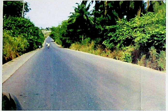
Partly completed Amansea - Ebenebe Road
