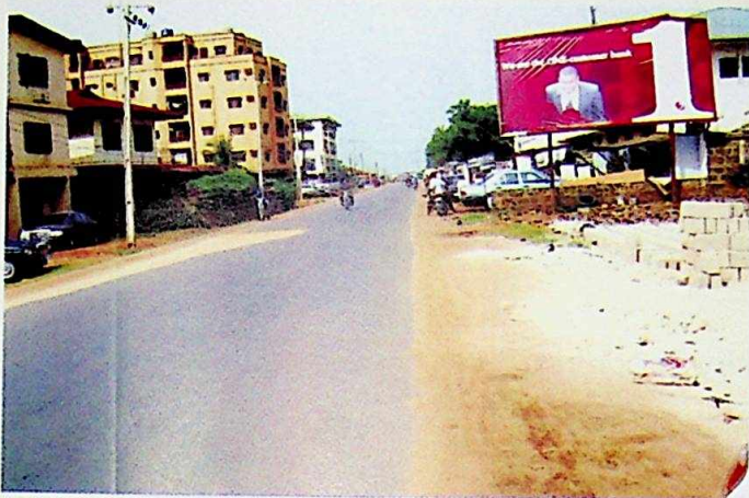
Completed Creek Road Fegge, Onitsha.
