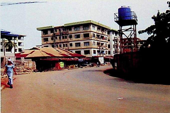
Completed Uzodinma Street, Fegge, Onitsha.
