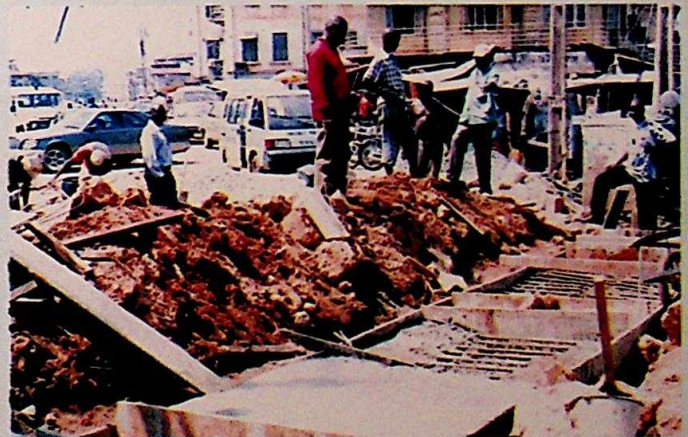
Construction of culvert at Iweka/Venn Rd Junction, Onitsha South LGA
