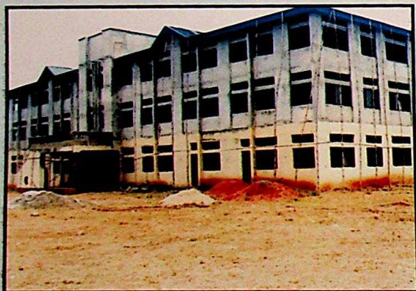
Newly completed Awka North Secretariat Building
