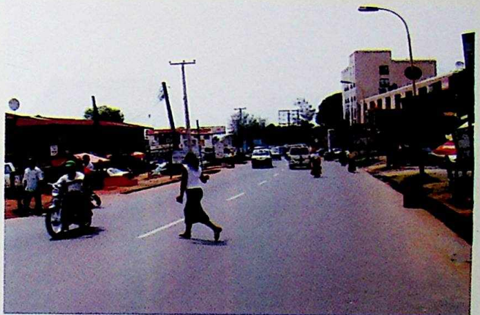
Completed Awka Road, Onitsha.
