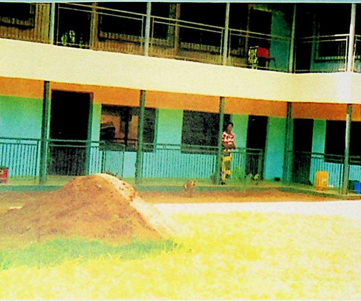
Rehabilitated Primary Health Centre, Akweze
