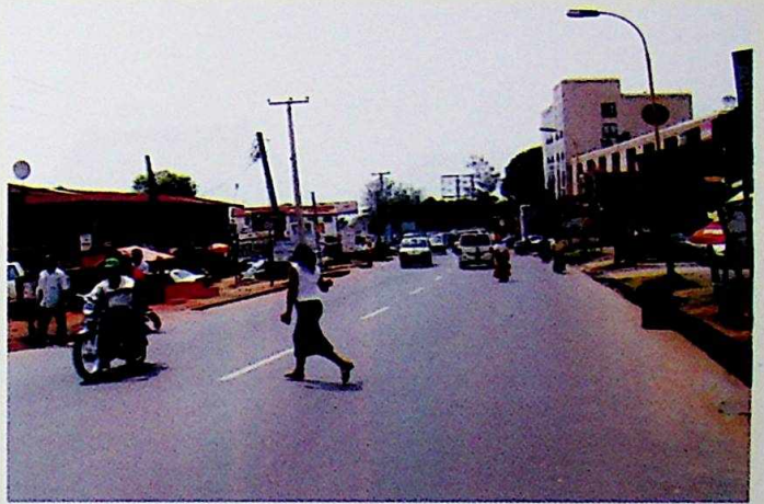
Completed Awka Road, Onitsha.
