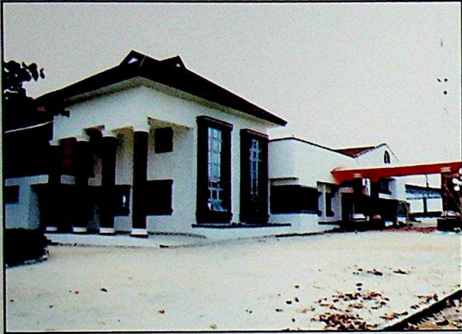
Governor's Lodge Amawbia: reconstructed and modernised by Governor Obi
