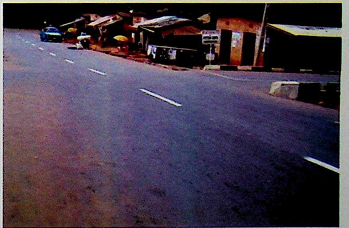
Completed Late Igwe Ejidike Road, Agulu
