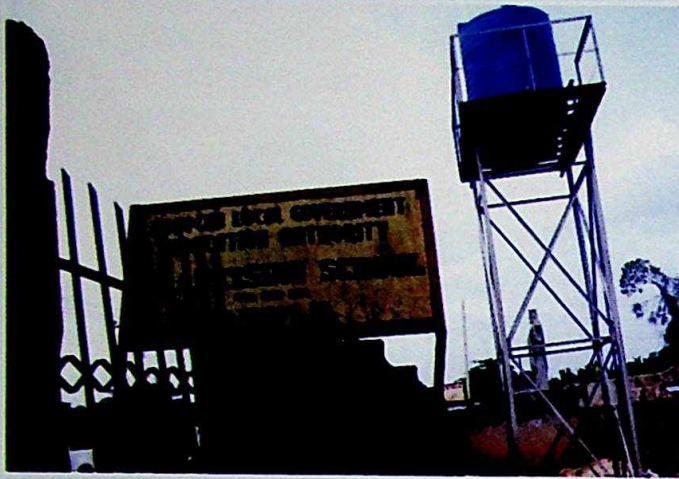
Solar-powered water borehole at Agulu Community
