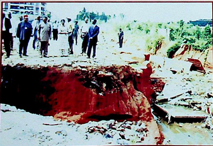
His Excellency inspecting an erosion site: the Government is tackling the erosion menace at numerous sites all over our erosion-ravaged State
