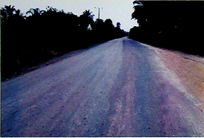
Partly completed Ajali - Ogboji Road
