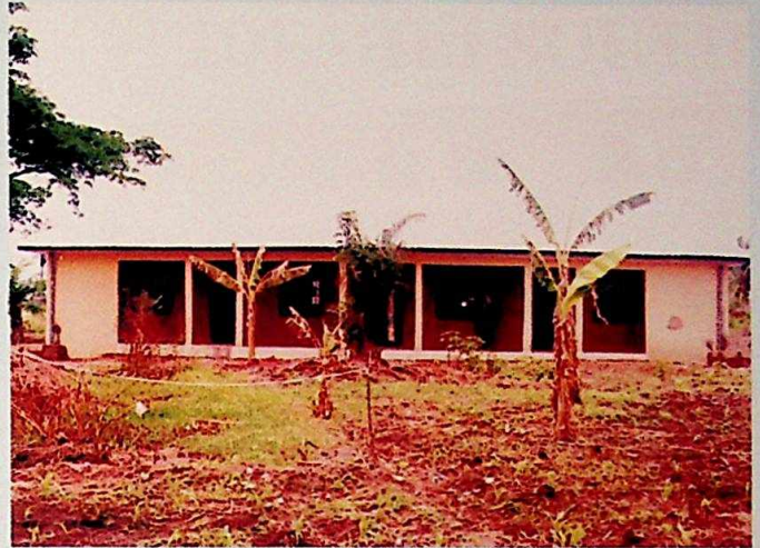
New Health Centre at Umumbo
