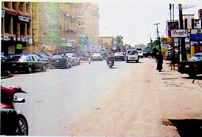
Completed Old Market Road, Onitsha.
