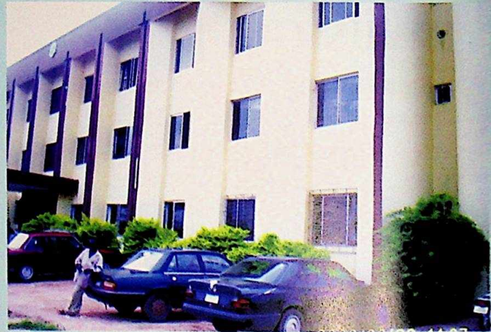
Renovated Oyi LGA Secretariat
