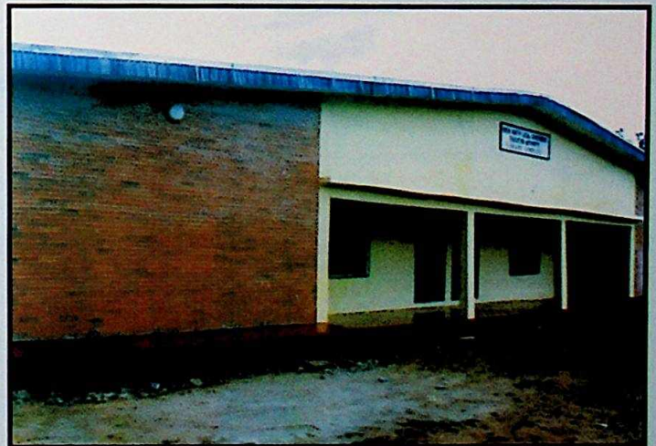
Renovated Library Complex at Nnewi North LGA
