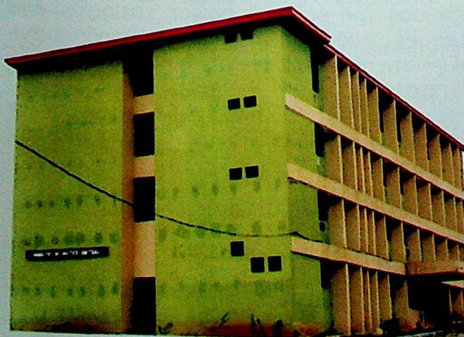
Completed office block of Ministry of Justice, Onitsha
