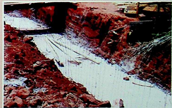
Reinforcement of Flood channel with BRC mesh.
