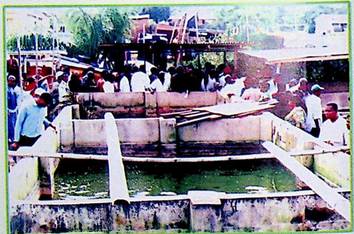
The newly rehabilitated Ufuma Fish Farm
