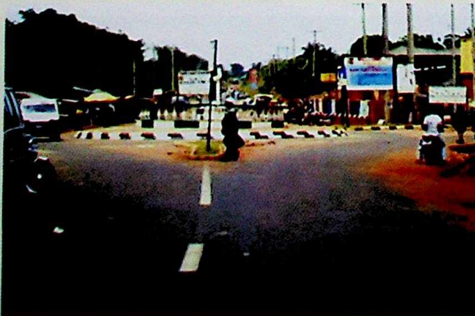
Completed Otuocha - Aguleri Road
