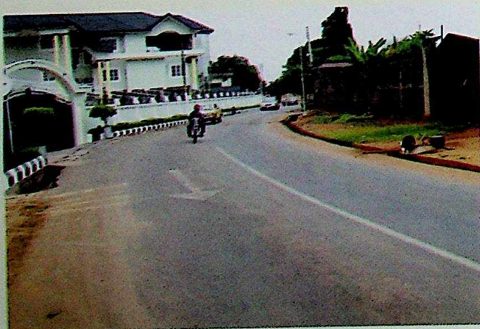
Completed Bent Lane G.R.A., Onitsha.
