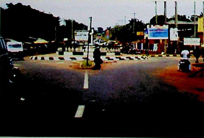
Completed Otuocha - Aguleri Road
