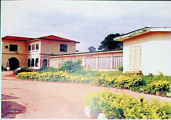
The refurbished Onitsha General Hospital
