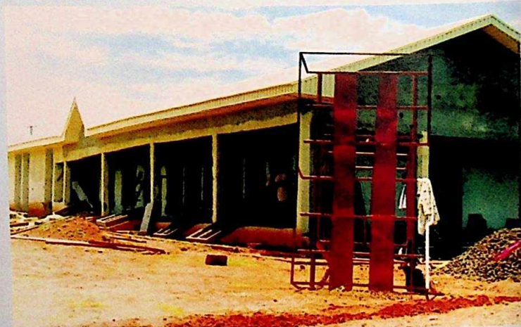
New Magistrate Court Building, Anambra East LGA
