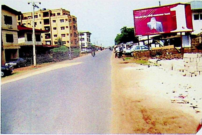
Completed Creek Road Fegge, Onitsha.
