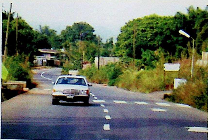
Completed Nanka - Oko Bypass Road
