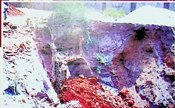
The Gully head to be completely reclaimed.
