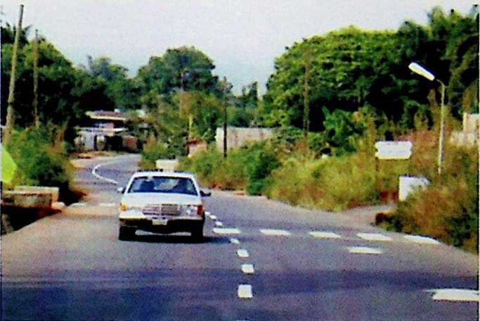
Completed Nanka - Oko Bypass Road
