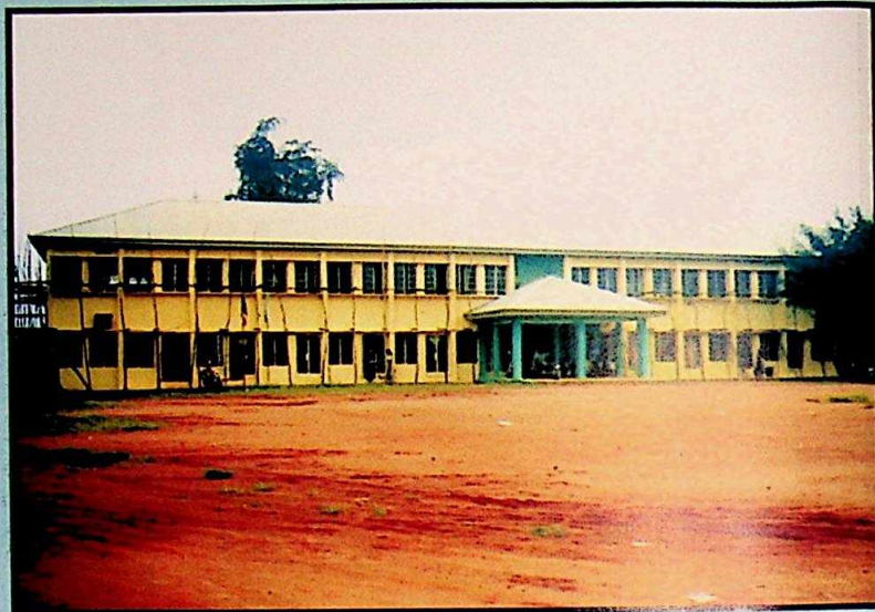
Renovated Admin block, Aguata LGA
