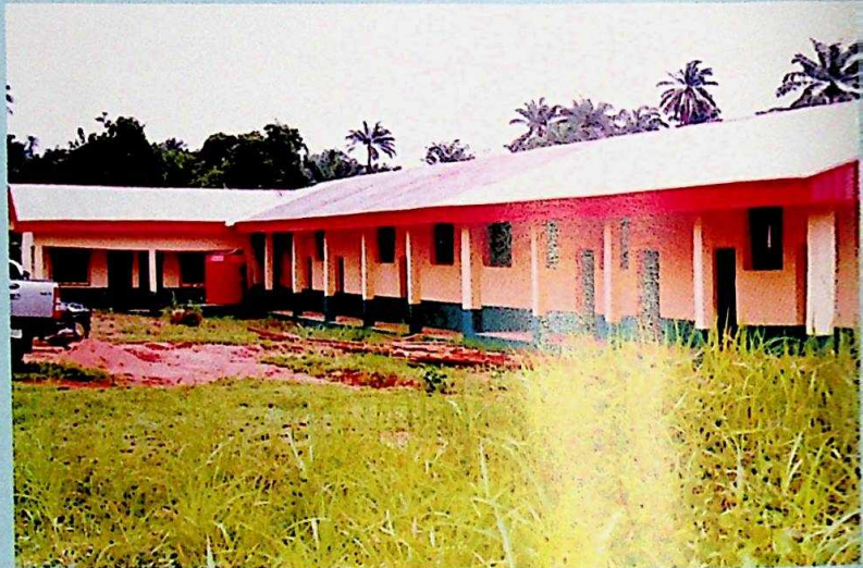
Newly completed school project at Umudiala, Ezenifite, Nnewi South LGA
