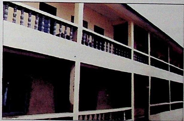
A HOSTEL BLOCK AT THE SCHOOL OF NURSING, AMACHARA
