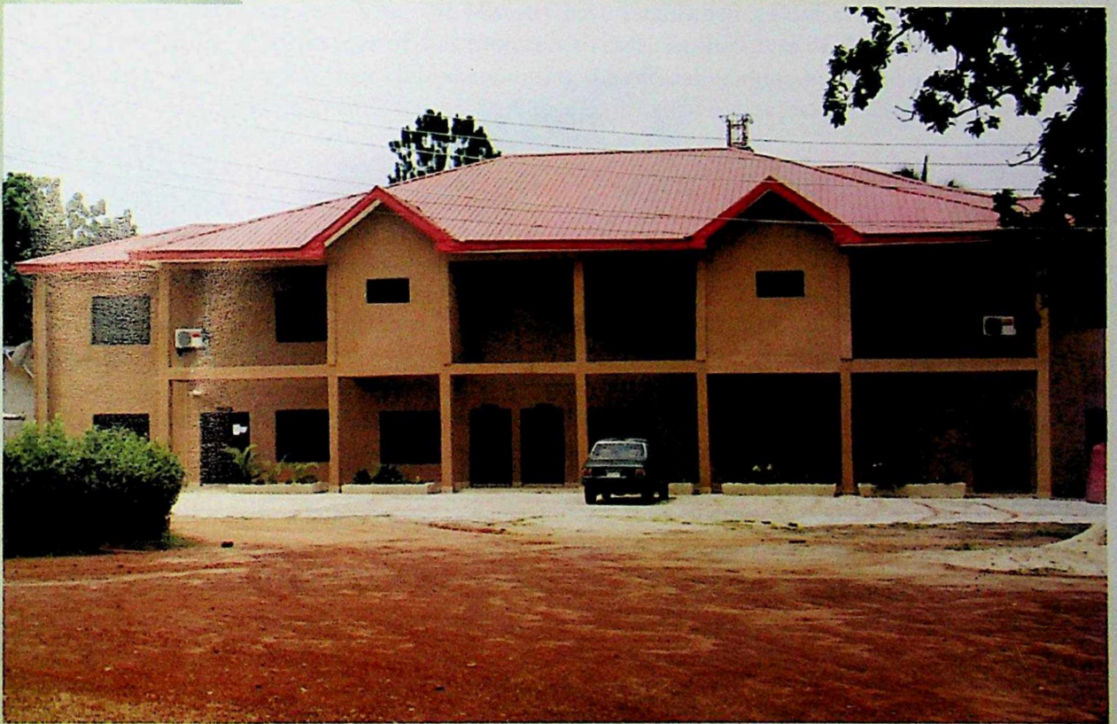
NEW ADMINISTRATIVE BUILDING AT THE MINISTRY OF JUSTICE
