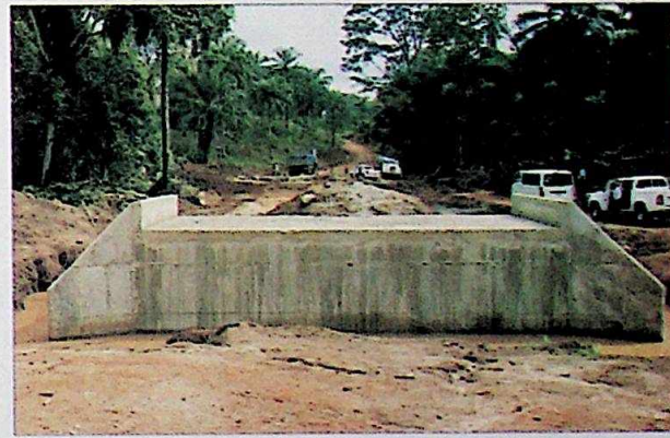
ONE OF THE 4 BOX CULVERTS ON AMAOGGWUGWU-UMUEKWULE-UMUKABIA ROAD.
