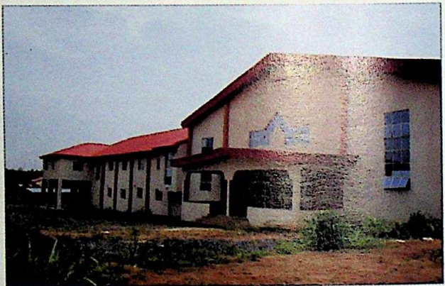
COMPLETED SECRETARIAT OF THE ABIA STATE COUNCIL OF TRADITIONAL RULERS
