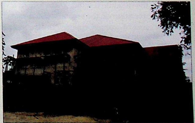
DEPUTY GOVERNOR'S LODGE NEARING COMPLETION
