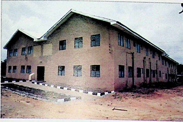
COMPLETED HOSTEL BLOCK AT THE SCHOOL OF NURSING QUEEN ELIZABETH HOSPITAL, UMUAHIA
