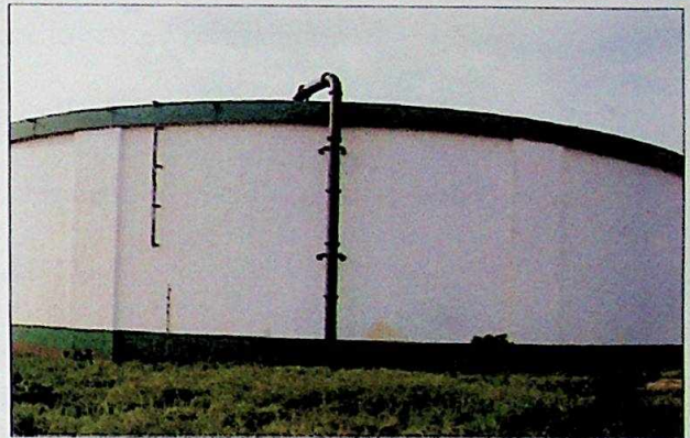
FENCING IN PROGRESS OF THE WATER RESERVOIR AT BENDE ROAD
