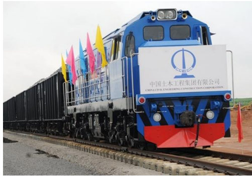
Abuja – Kaduna Rail line
