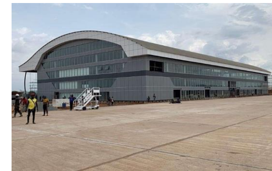
Anambra State International Airport
