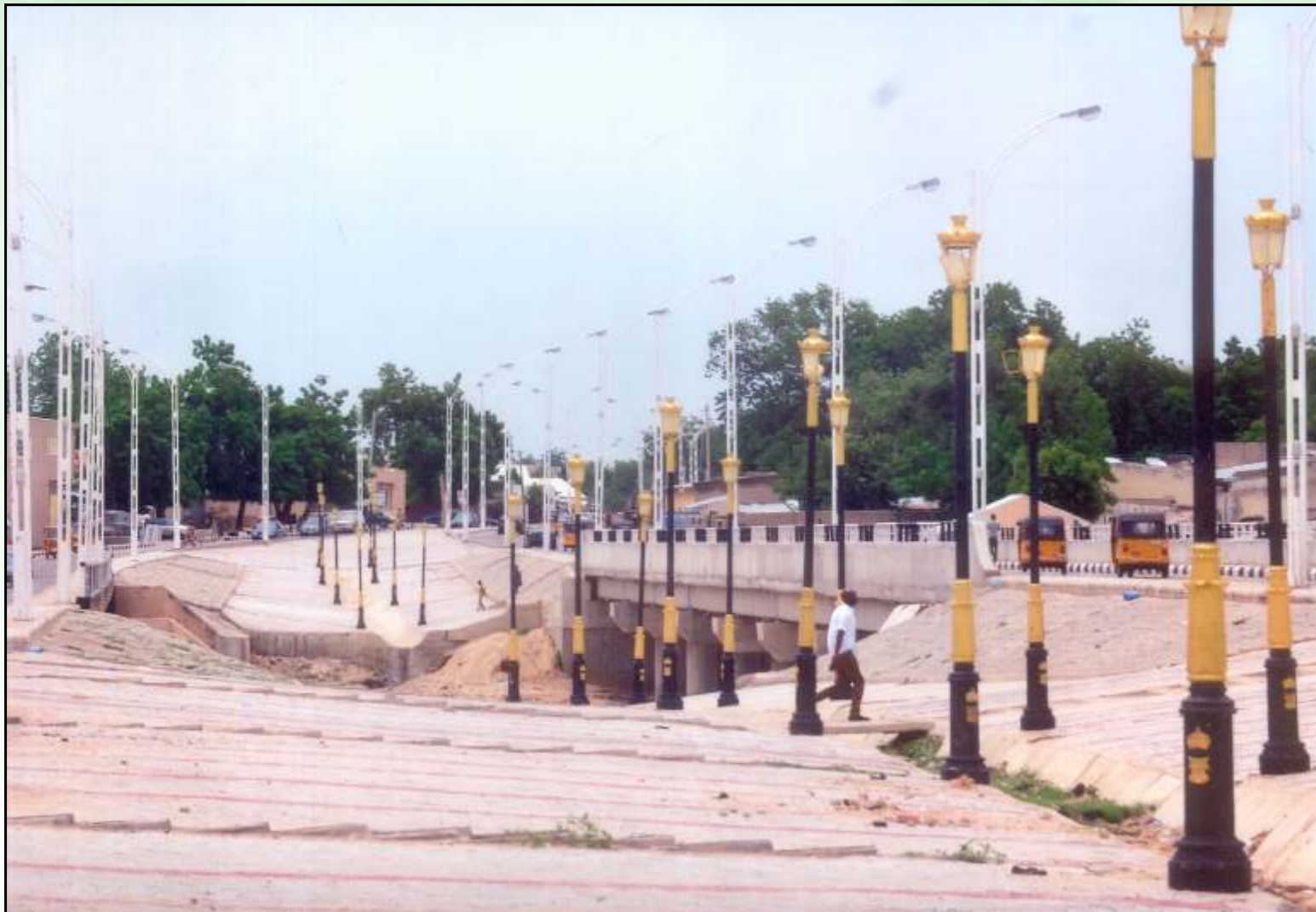
Dual - Carriage Bridge, Lagos Street, Maiduguri
