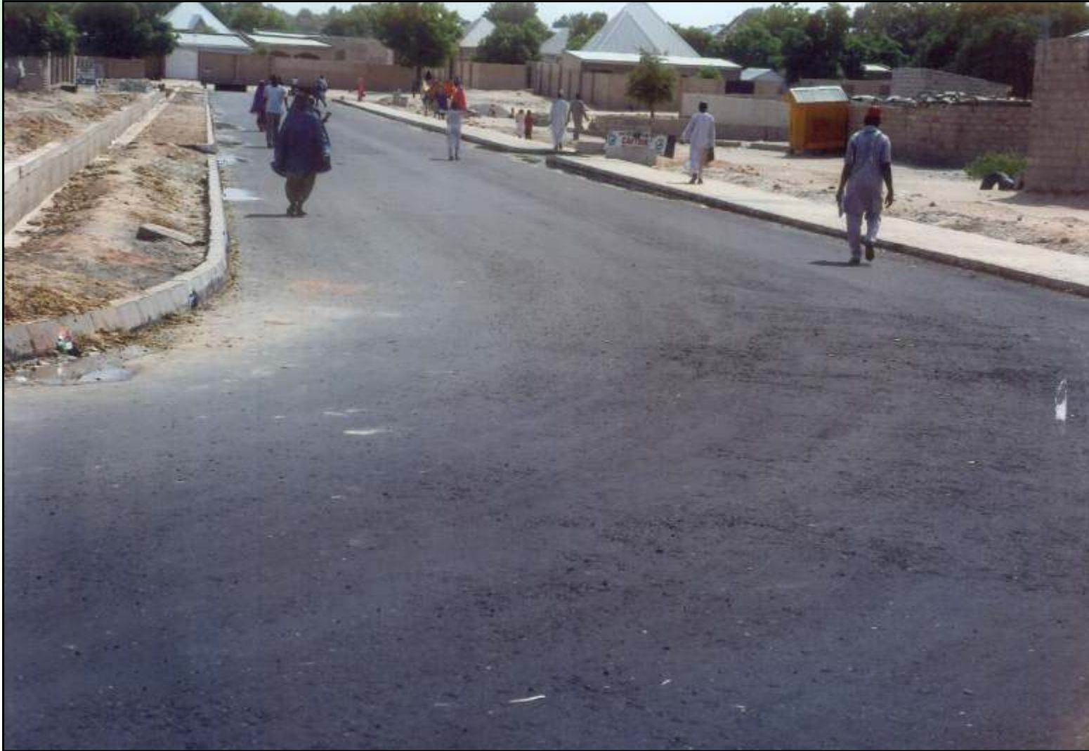
Fori - Galtimari Road Construction and Drainage, Maiduguri
