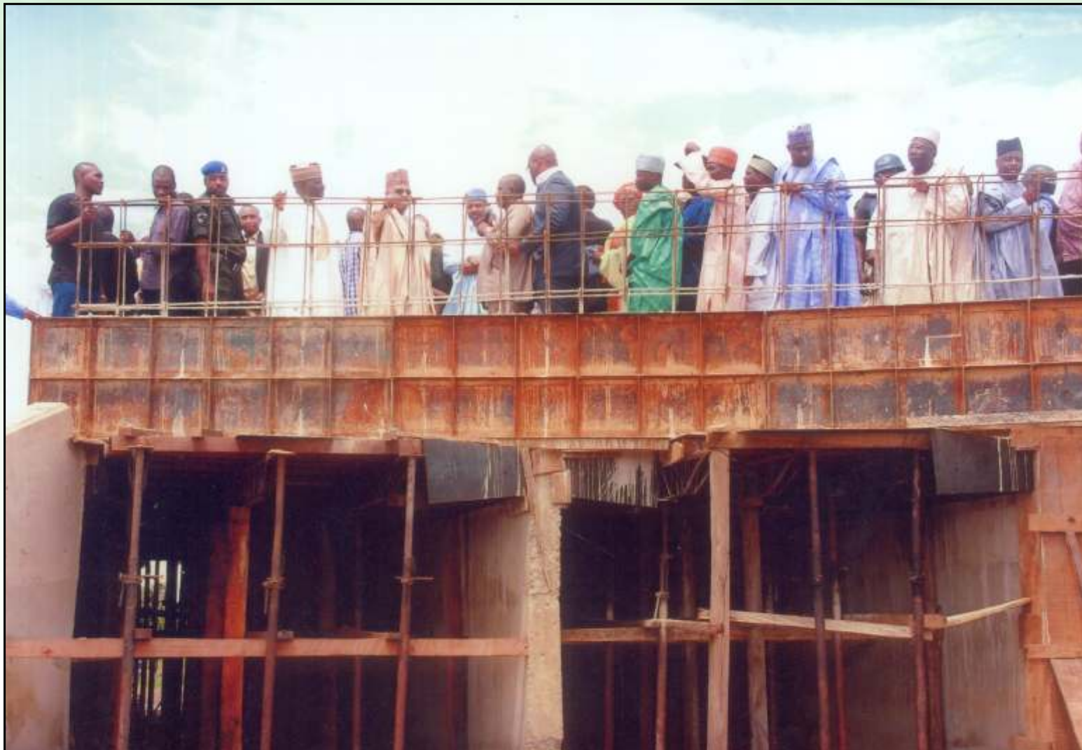
Garubula Double Culvert Under Construction on Miringa-Gurda Road, Biu Local Government
