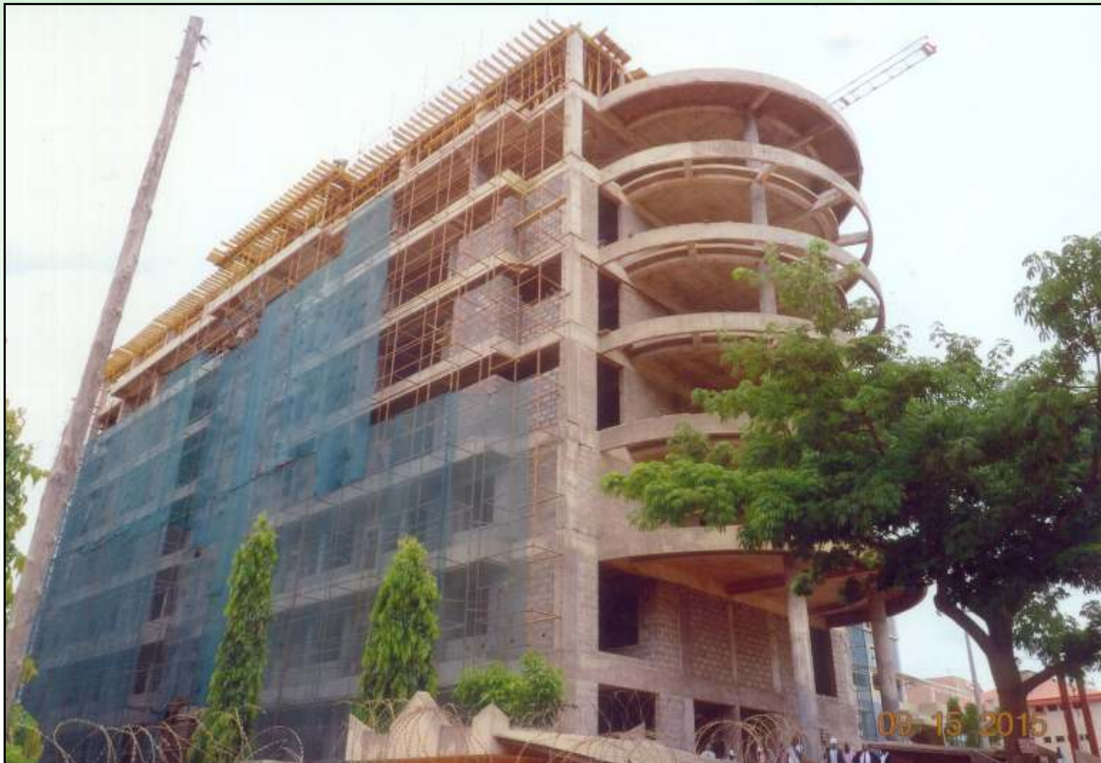
New Borno House Abuja Under Construction
