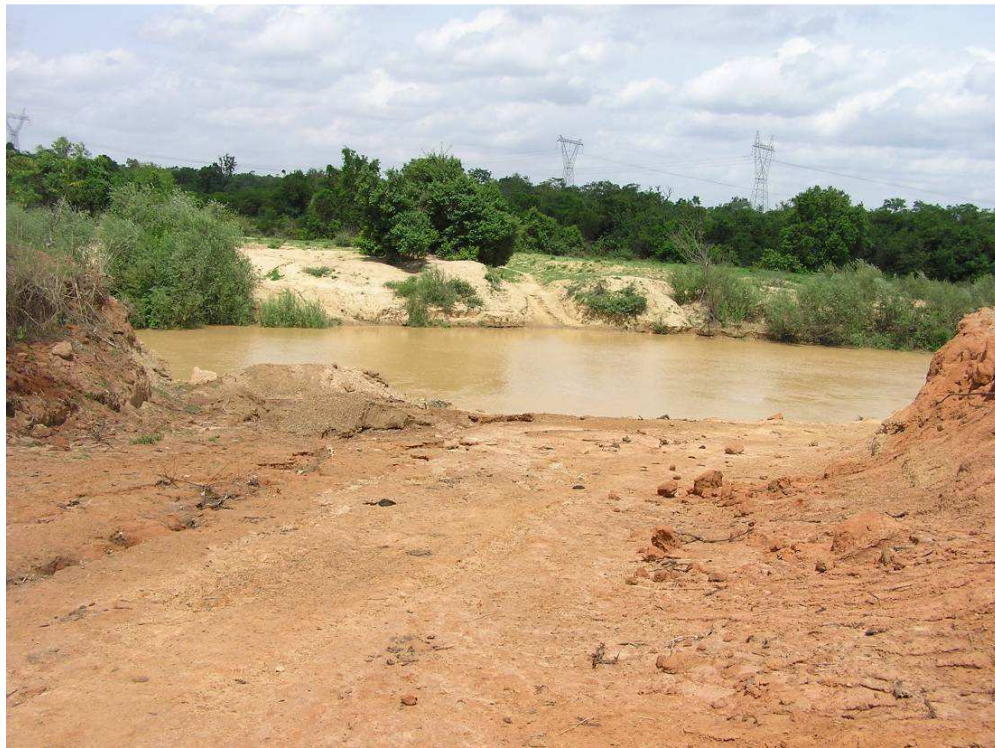
Photo 2 : General view of Masaka dam site
