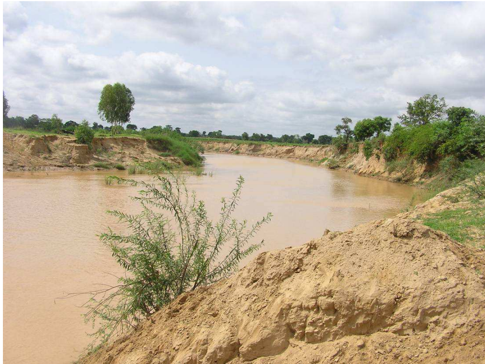
Photo 1 : General view of Yola Buruku dam site
