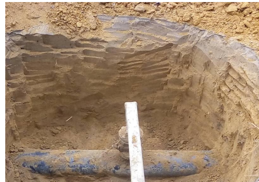
Some of the 41 illegal connections discovered on the 6.7km to Imo River Line (2.5km stretch) 5/6/2021
