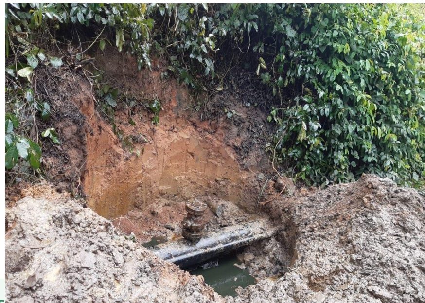
Some of the 41 illegal connections discovered on the 6.7km to Imo River Line (2.5km stretch) 5/6/2021
