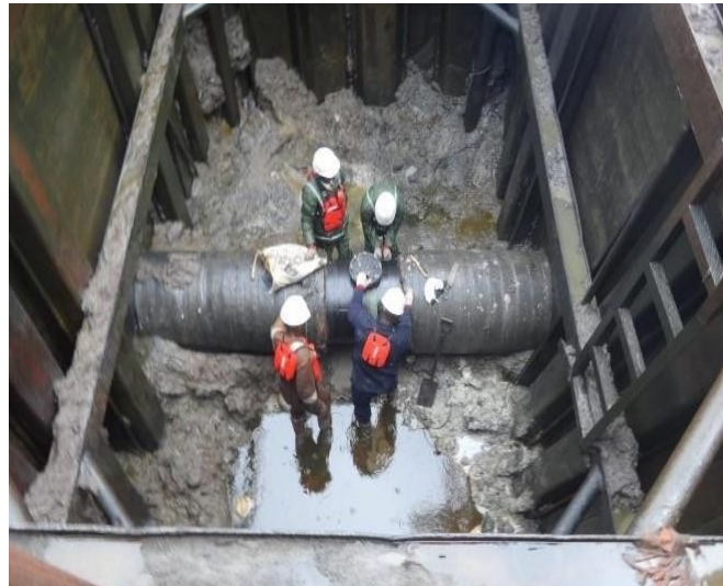
Crude Oil theft points under repair
