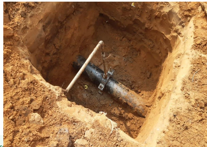
Some of the 41 illegal connections discovered on the 6.7km to Imo River Line (2.5km stretch) 5/6/2021
