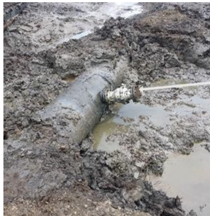
16" Nun River TL blown up using explosive. (sabotage)
