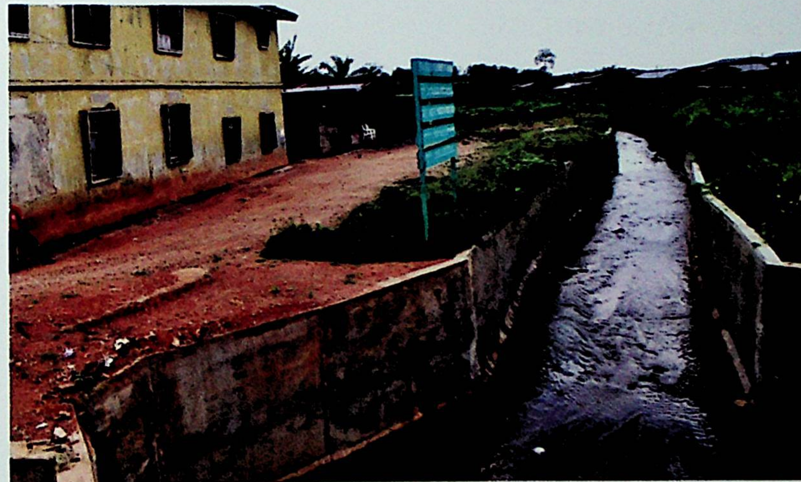
Newly constructed storm water channel at Oke-Aro, Akure
