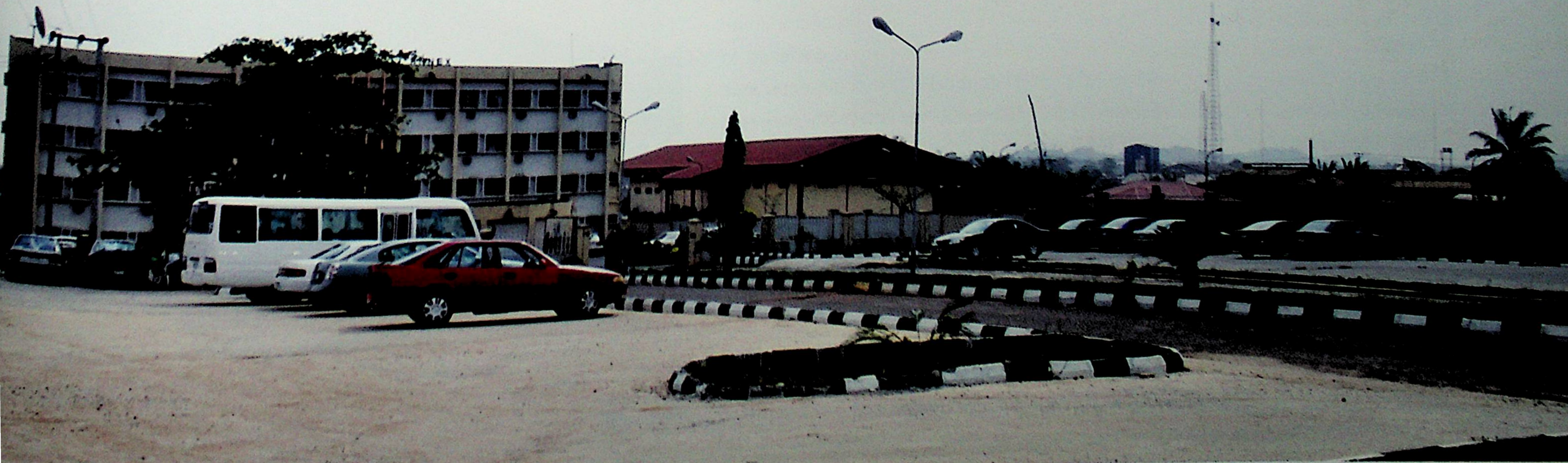
Newly constructed Parking Lots at Secretariat Annex Ilesha-Owo Expressway, Akure
