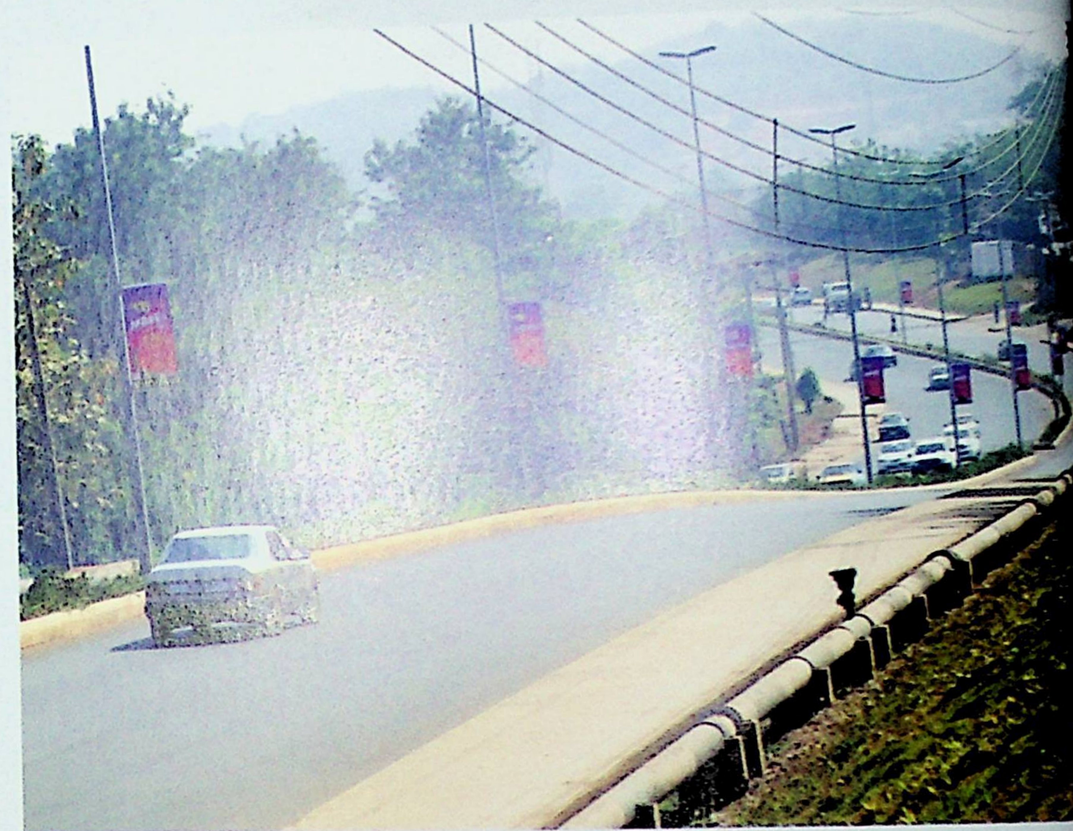
Section of Oba Adeshida newly completed with Street Lights & Landscaping
