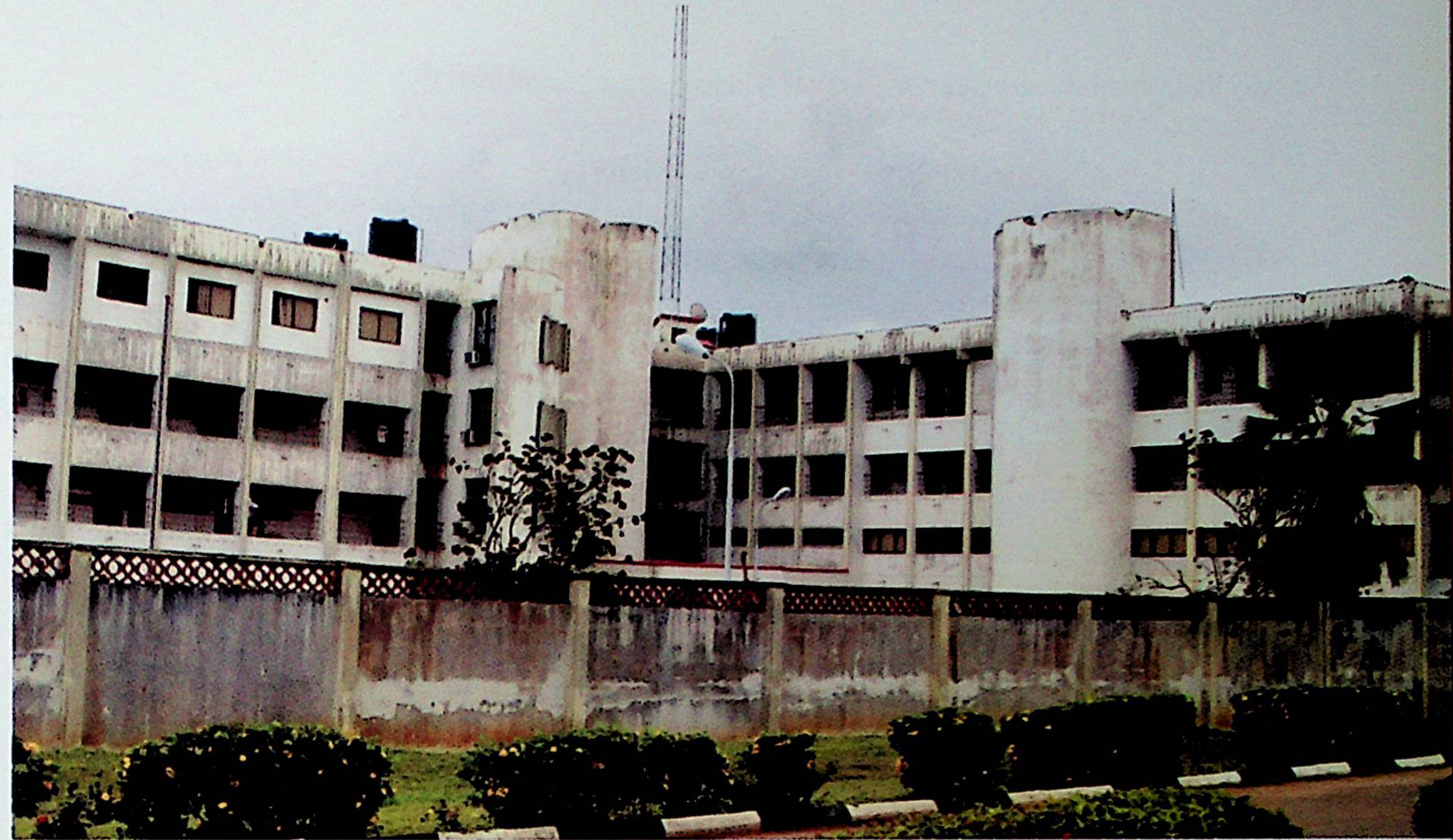
Government Secretariat Building Alagbaka, prior to comprehensive renovation
