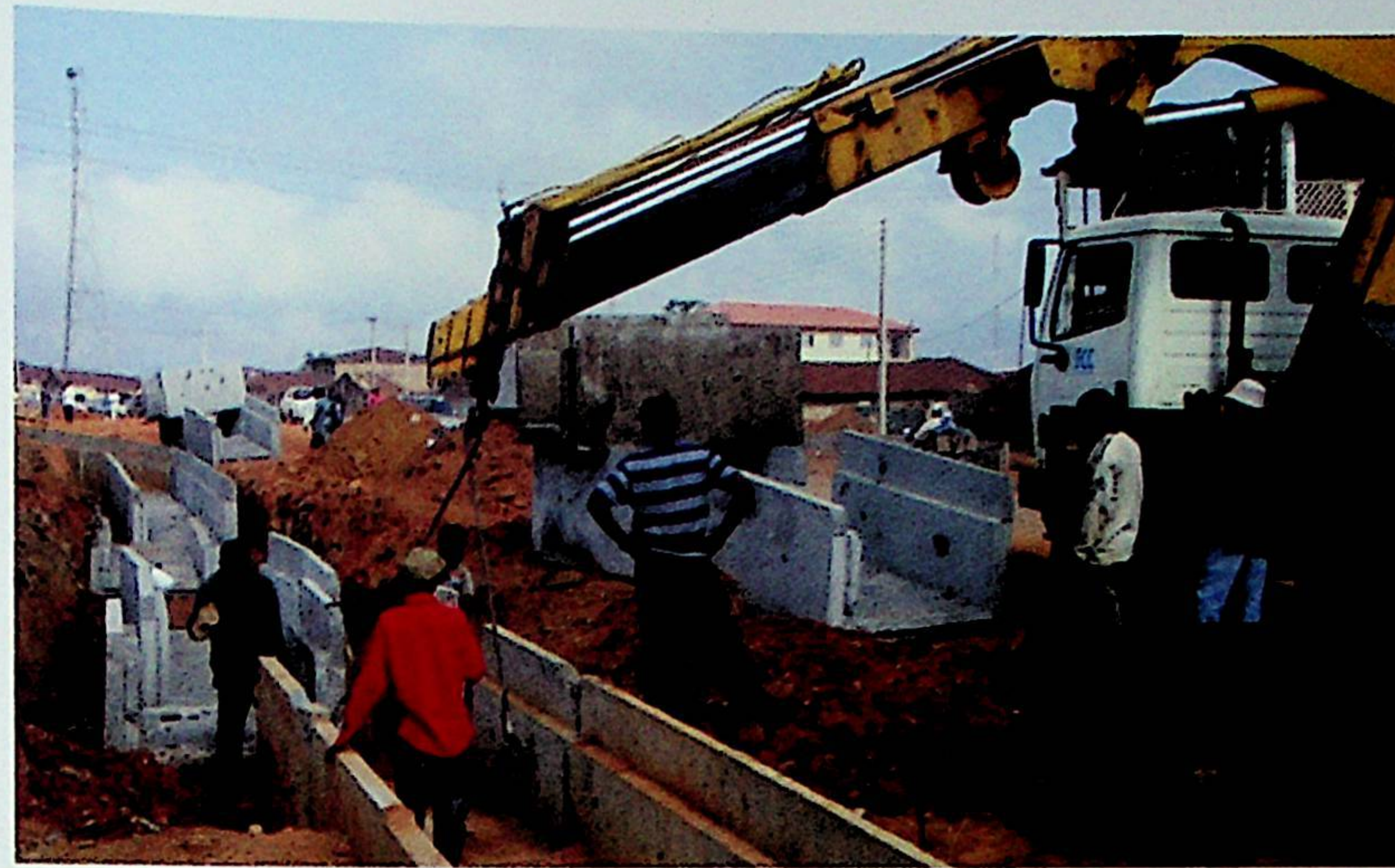
Construction of Drainage at Arakale, Akure
