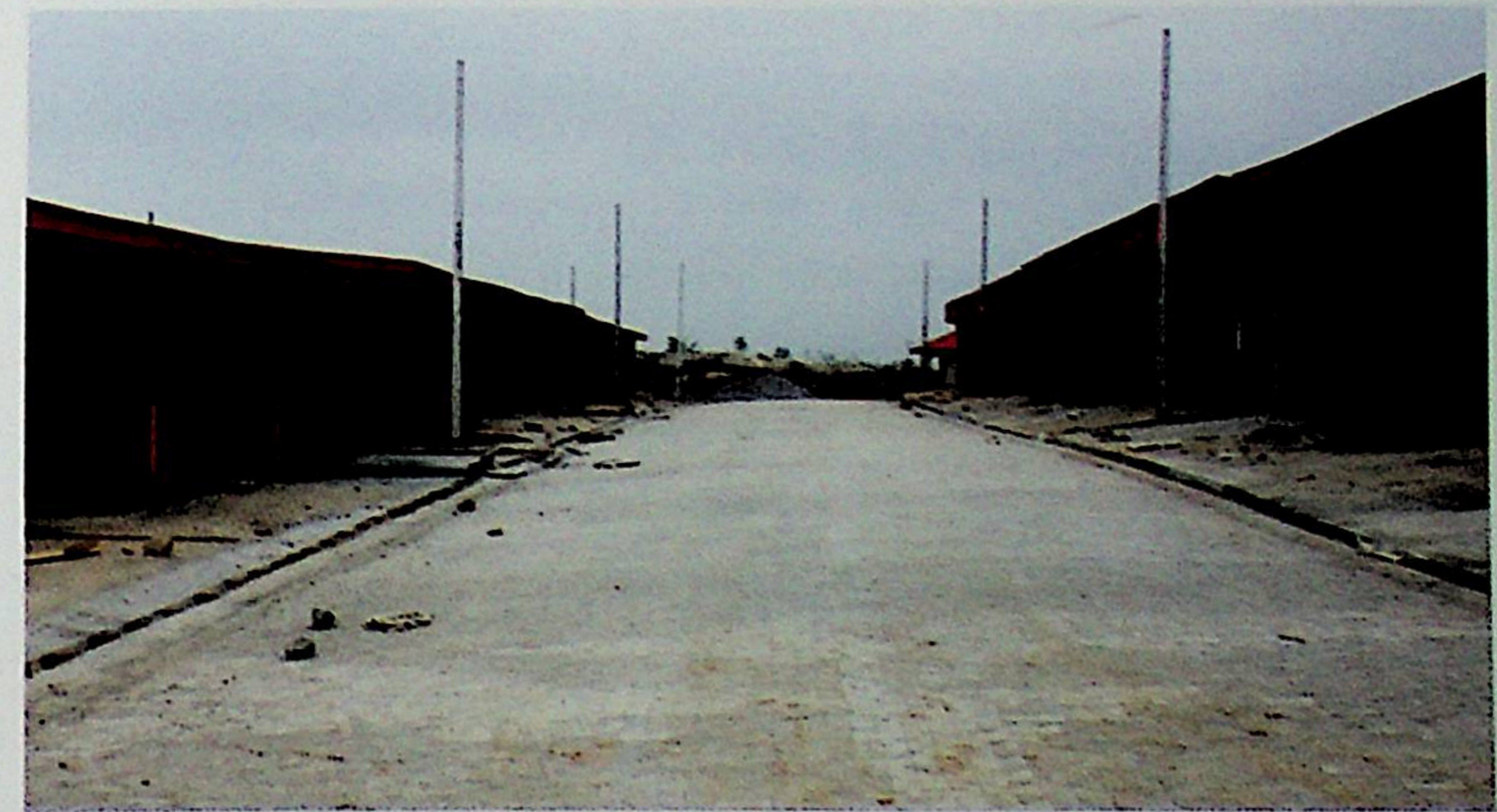
A Section of the on-going works at Modern Mechanic Village, Akure
