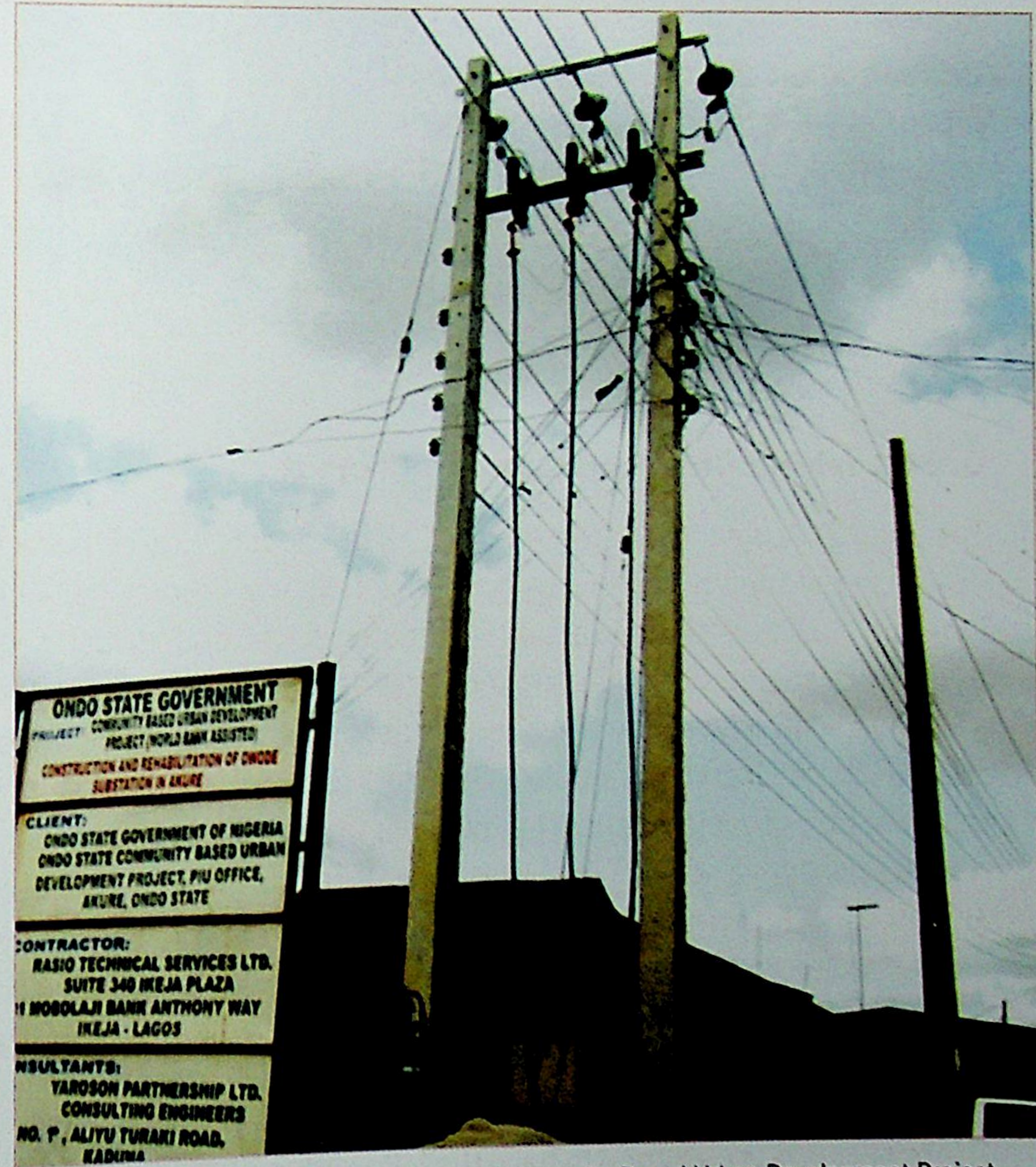
Electrification component of the Community-Based Urban Development Project
