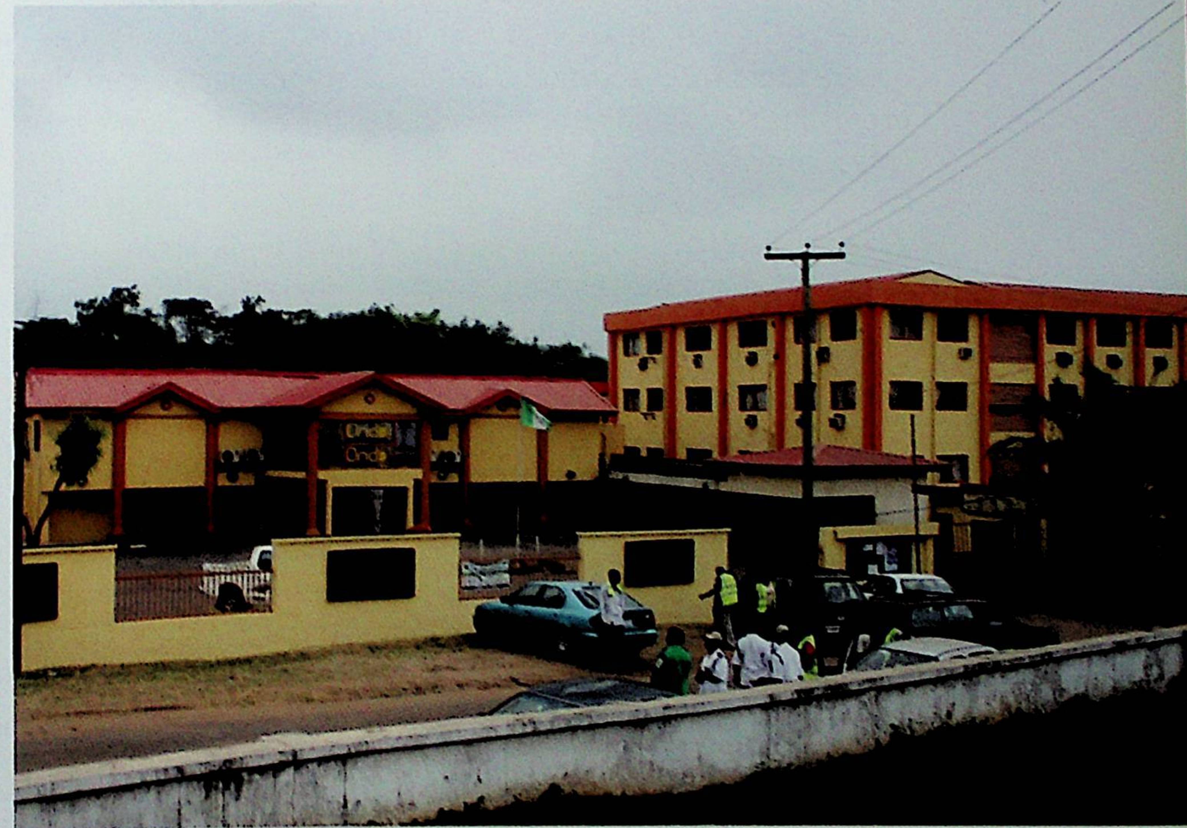
Renovated Ondo State Cultural Centre (Adegbemile), Akure
