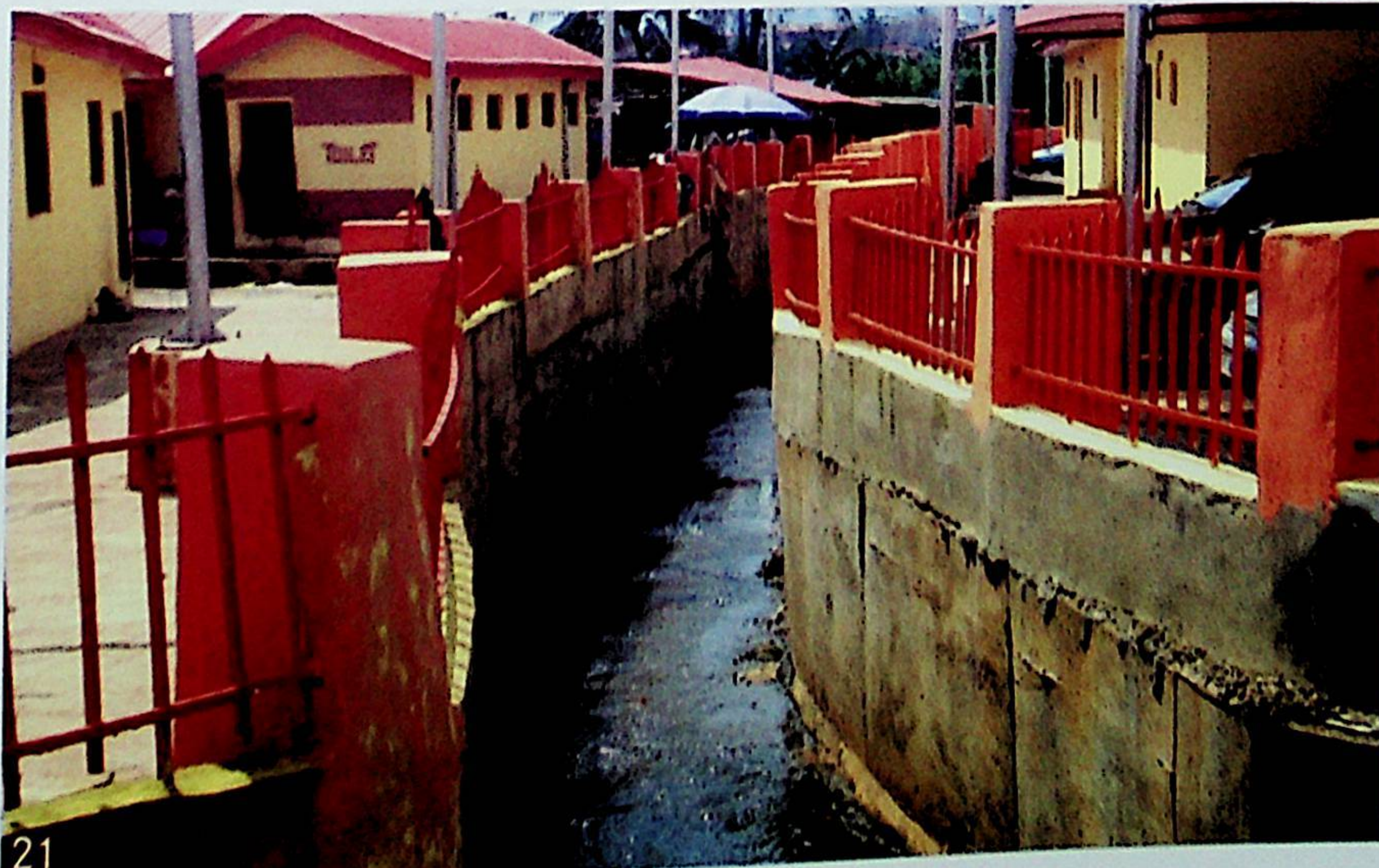
Storm Water Drainage
