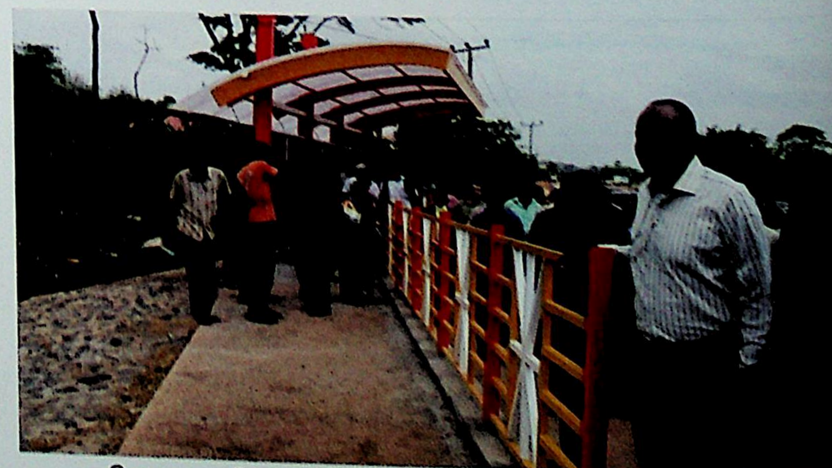
Governor Olusegun Mimiko on an Inspection of Road Project
