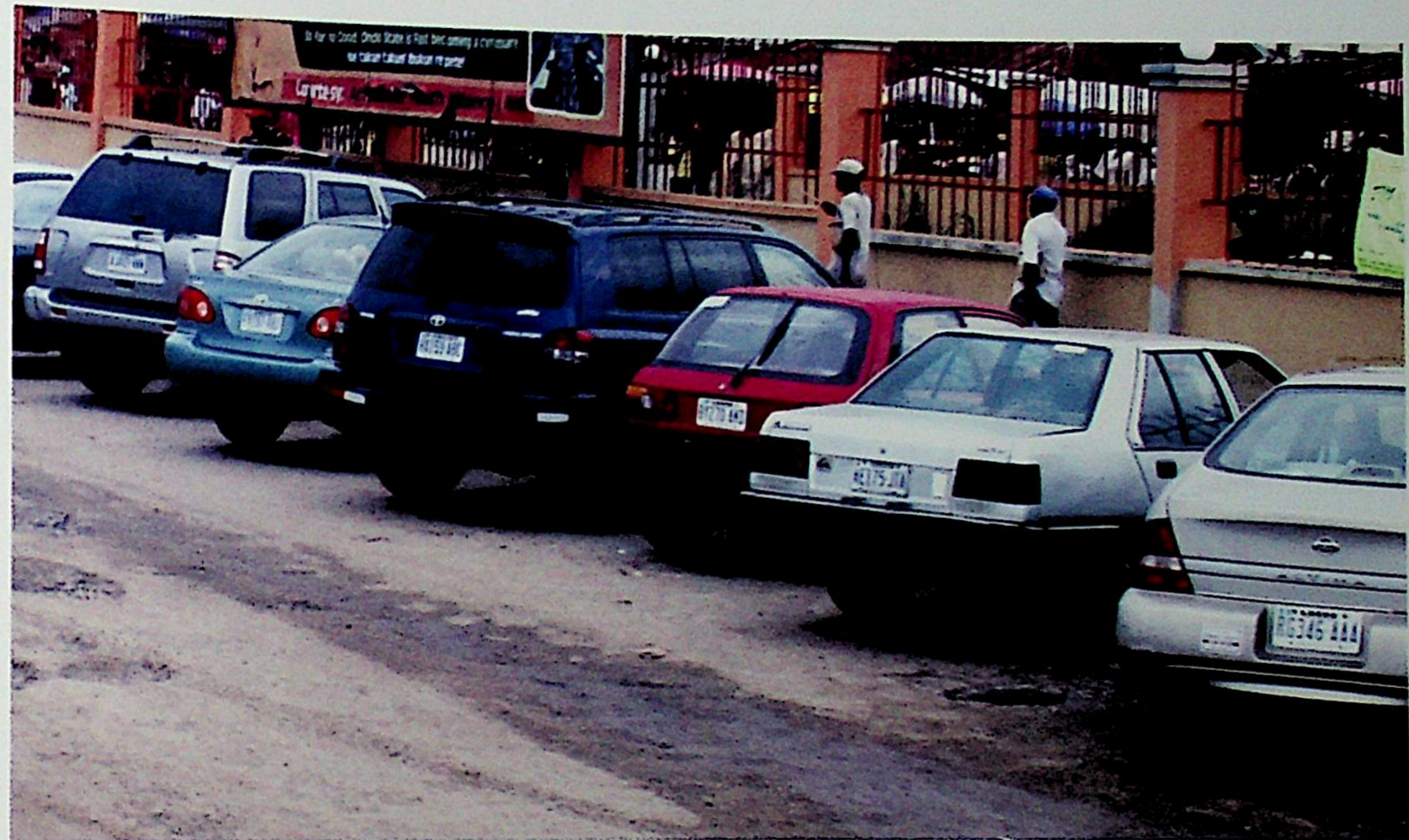
Newly constructed City Parking Lots at Olukayode Shopping Complex, Akure
