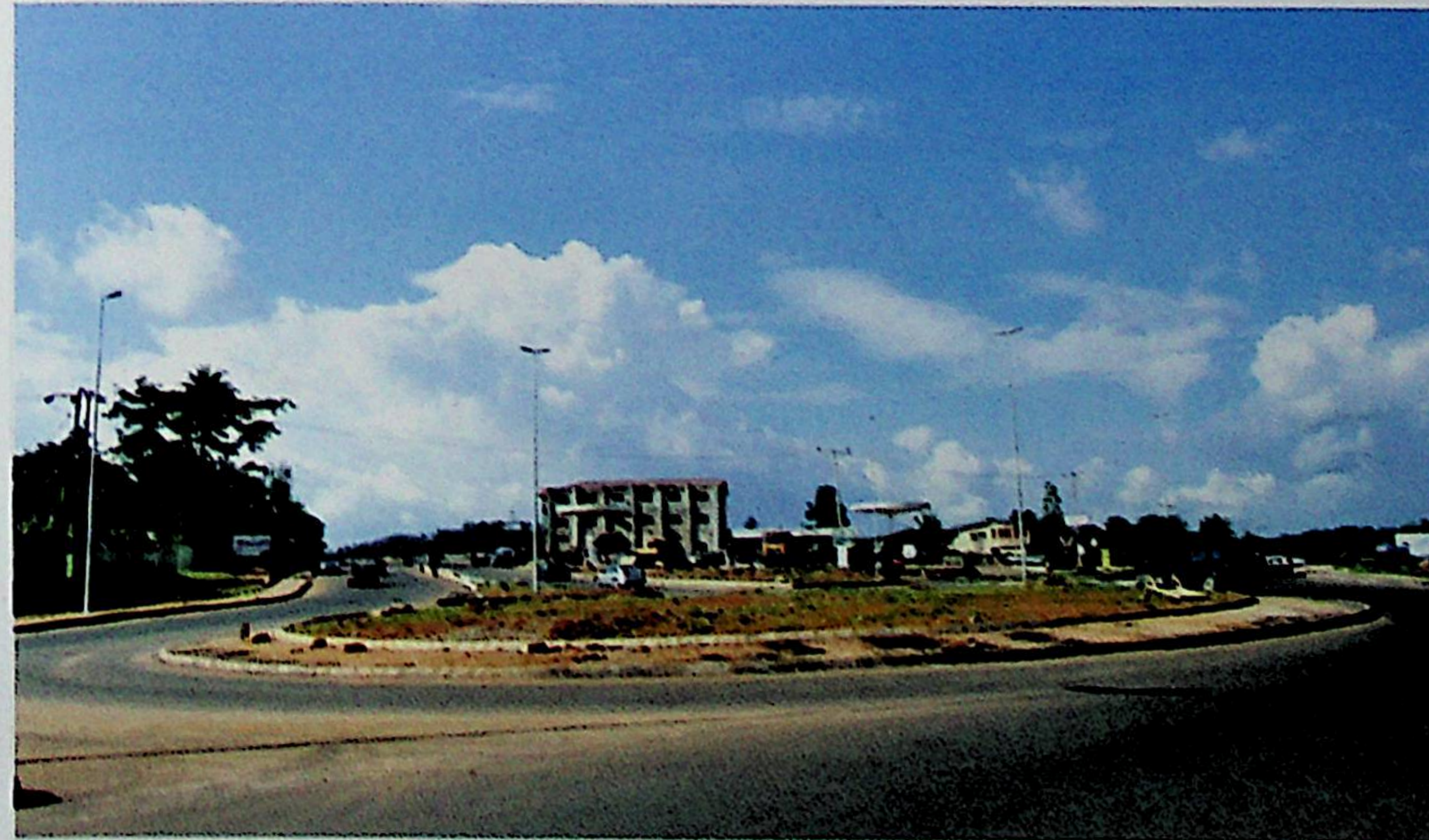
Cross section of on-going massive road construction to improve traffic flow in the State
