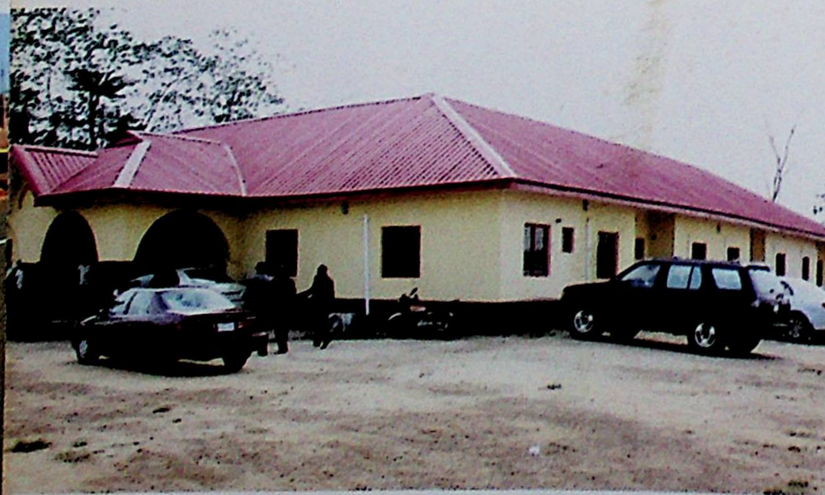
Administrative Block of Odigbo LGA Secretariat, Ore
